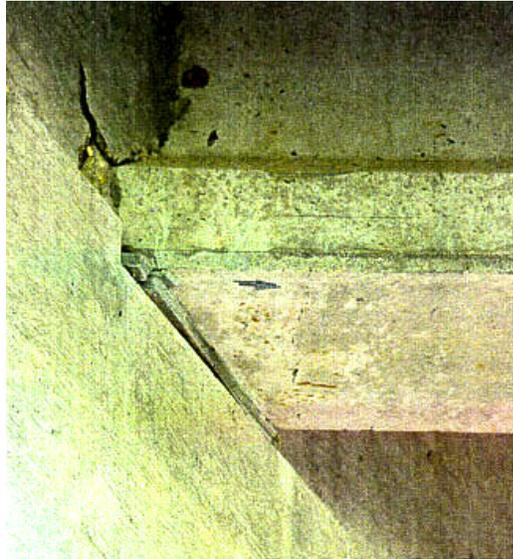
**Figure 0.2 Cracking in the Diaphragm Also Indicates Pull-out/Push-in Type of Loading of the Girders under Service Conditions**
