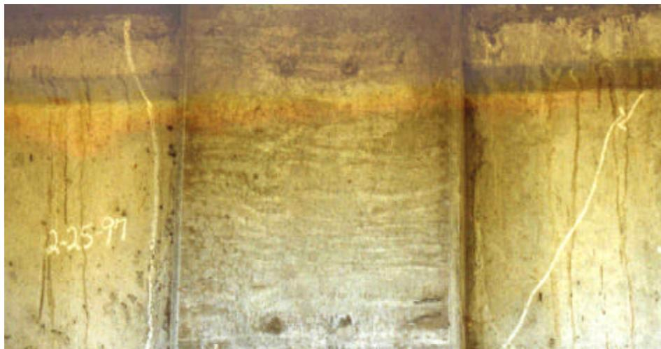
Note: The right girder demonstrates a typical crack due to diagonal tension, and the left girder shows a typical vertical crack
