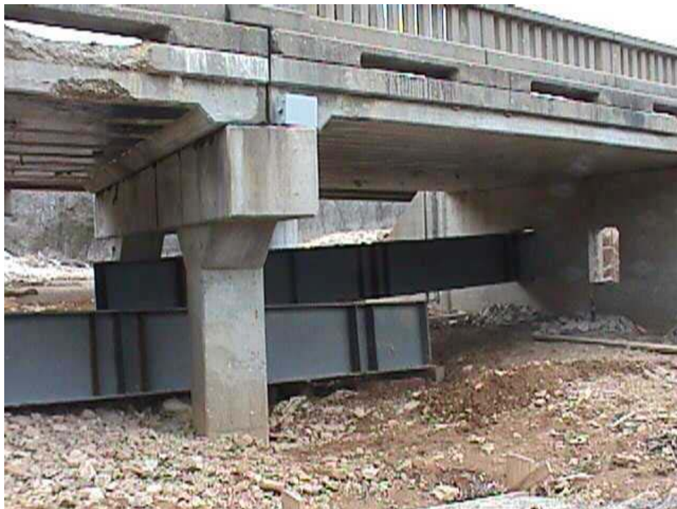
Figure 4.12. Installation of the steel girders.
