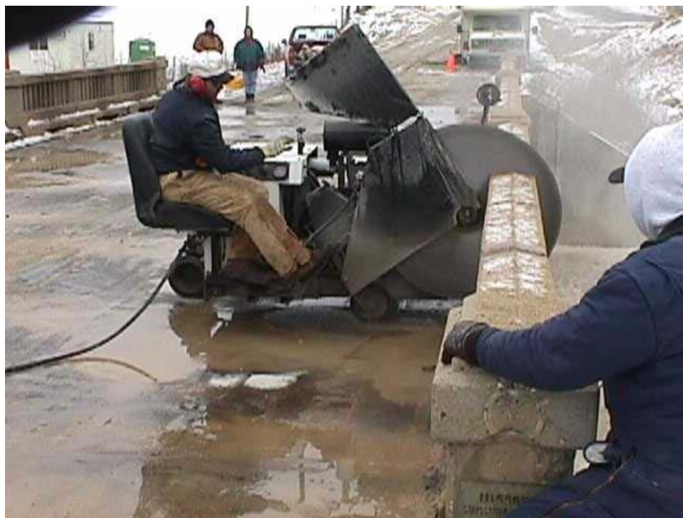
Figure 4.16. Cutting bridge parapet walls.
