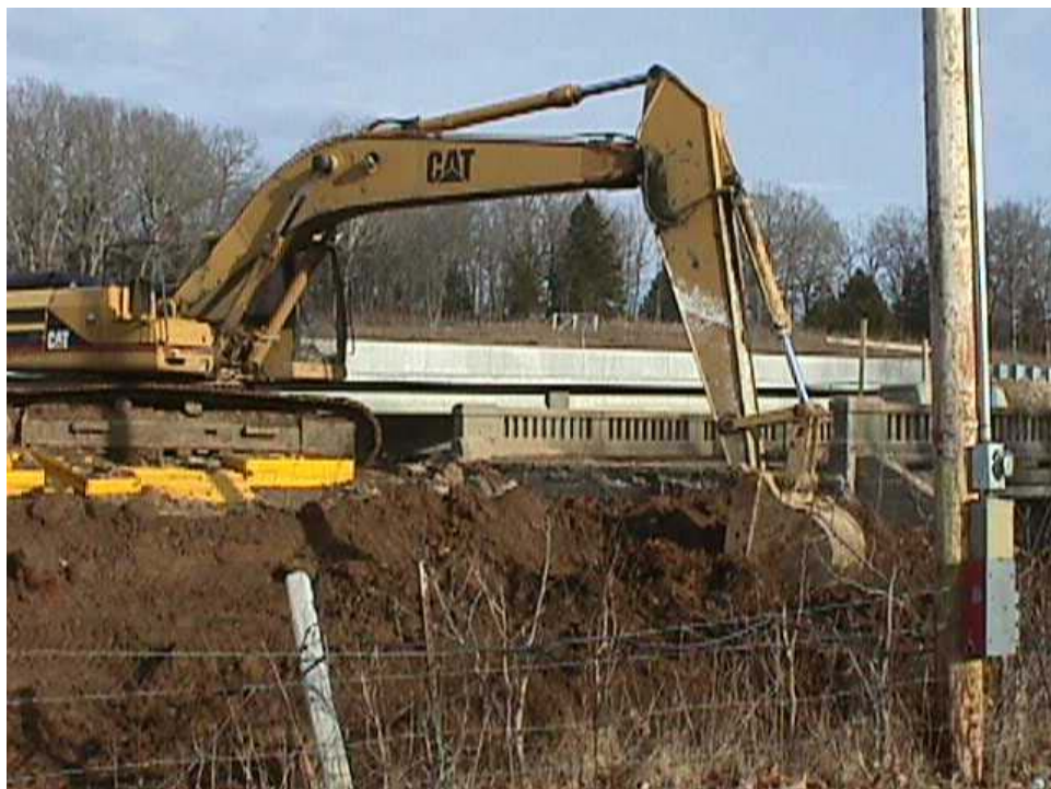
Figure 4.10. Excavating behind the bridge abutment.
