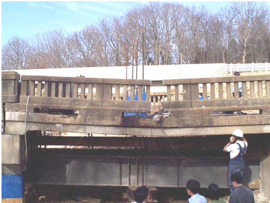
Figure 5.17. Deck 3 at failure.
