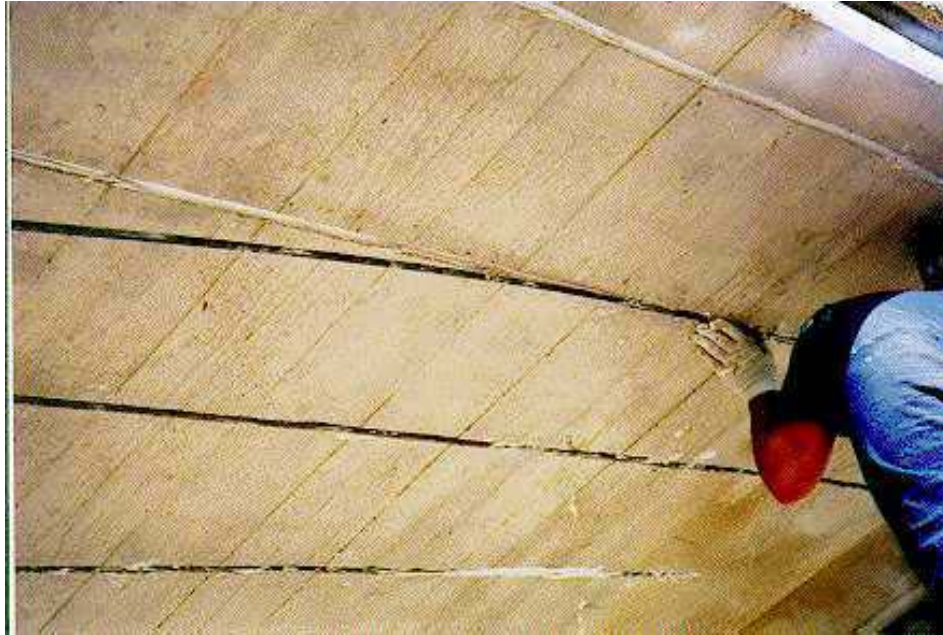
Figure 3.5. Installing the CFRP rods after filling the grooves halfway with epoxy paste.
