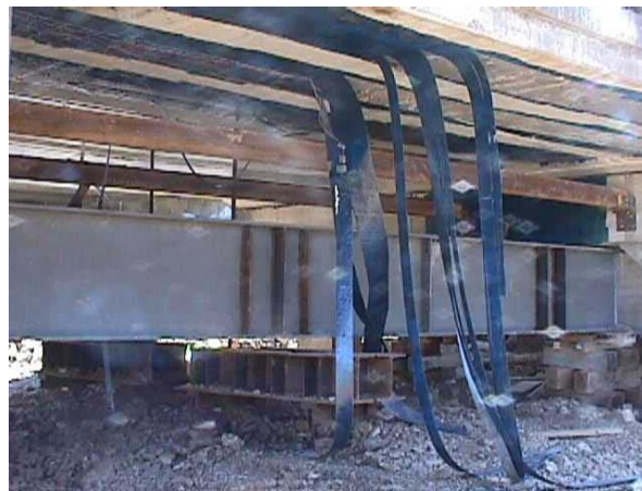
(b) Peeling of CFRP sheets
