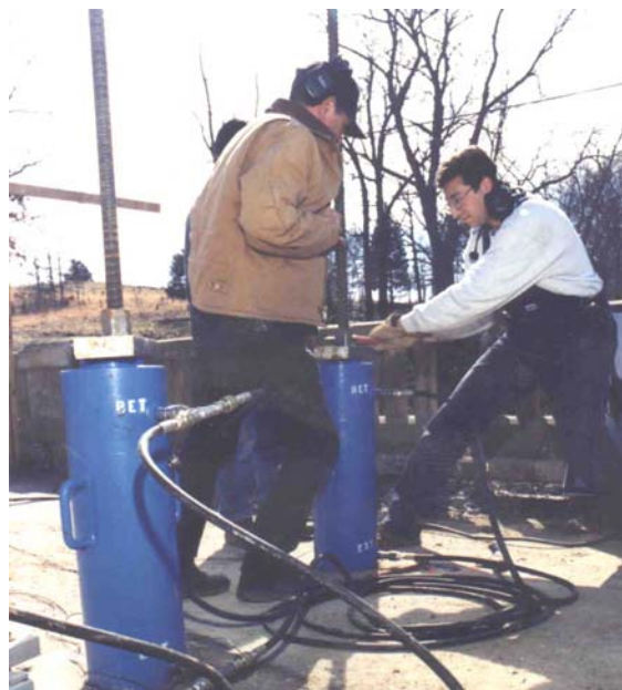
Figure 4.24. Tightening the nuts on the jacks in order to raise the steel girders.
