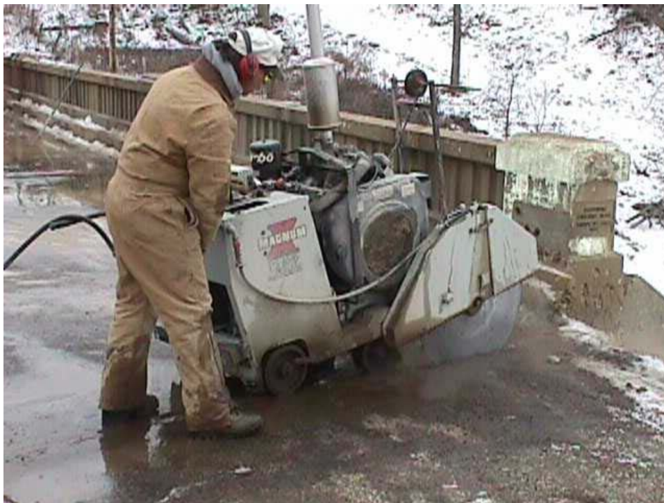
Figure 4.15. Cutting bridge deck joints.
