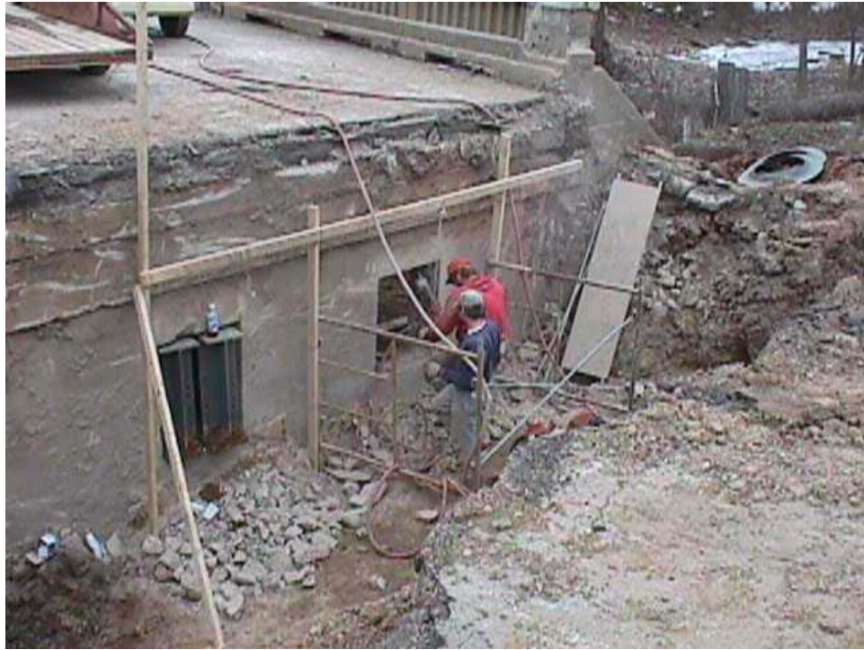
Figure 4.11. Bridge abutment after excavation and cutting.
