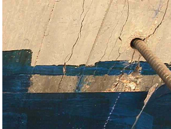
(a) Rupture of CFRP at formlines
