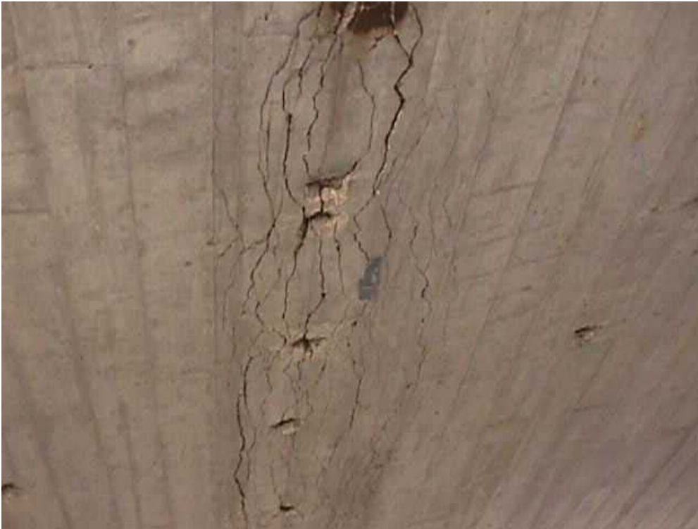
(a) Cracks on the deck soffit testing
