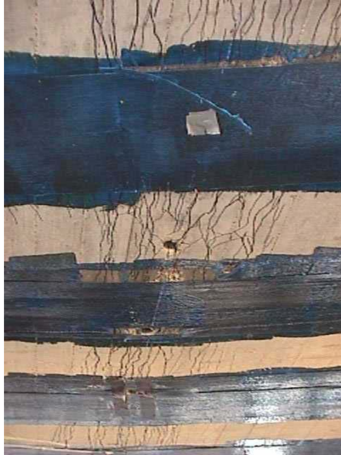
(a) Cracks on deck soffit
