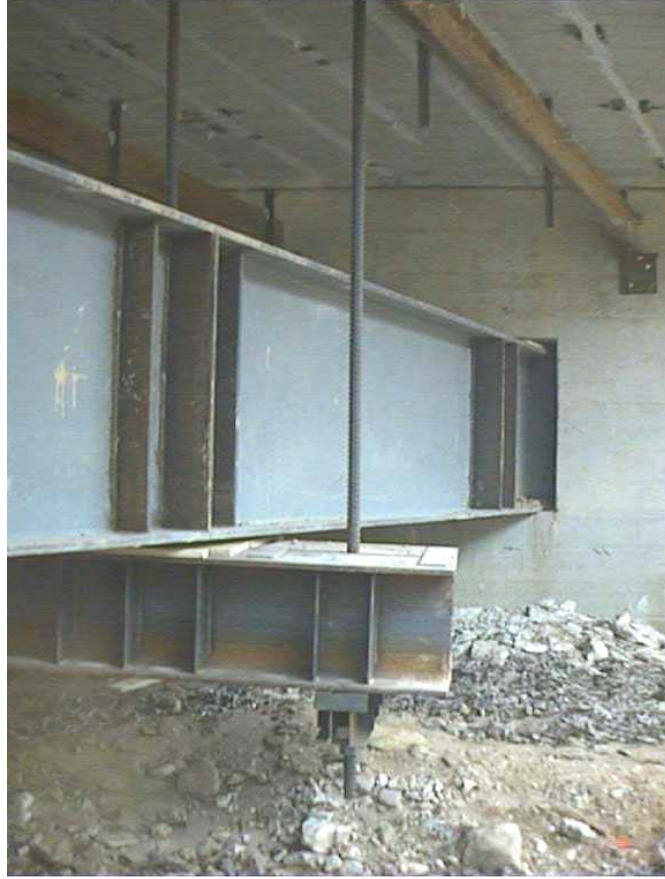
Figure 4.13. Assembled test setup for an end deck.
