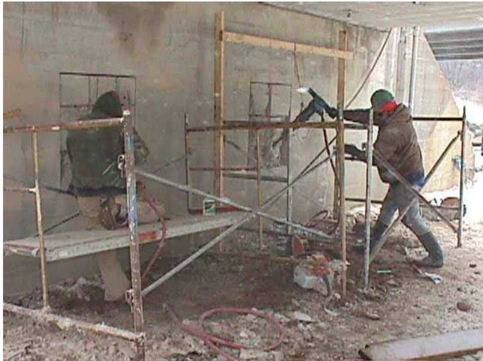
Figure 4.9. Cutting the bridge abutment.
