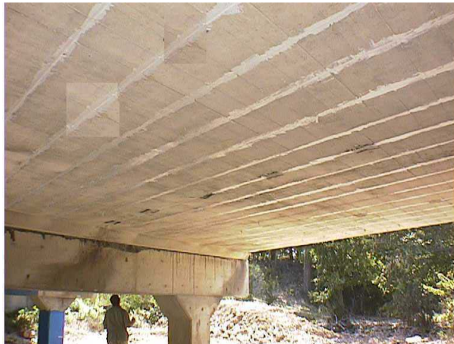
Figure 3.8. Deck 1 after strengthening with NSM rods.
