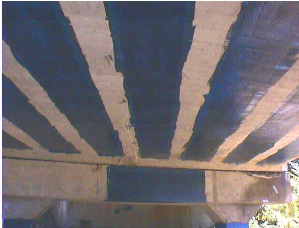
Figure 3.10. Deck 2 after strengthening with CFRP sheets.
