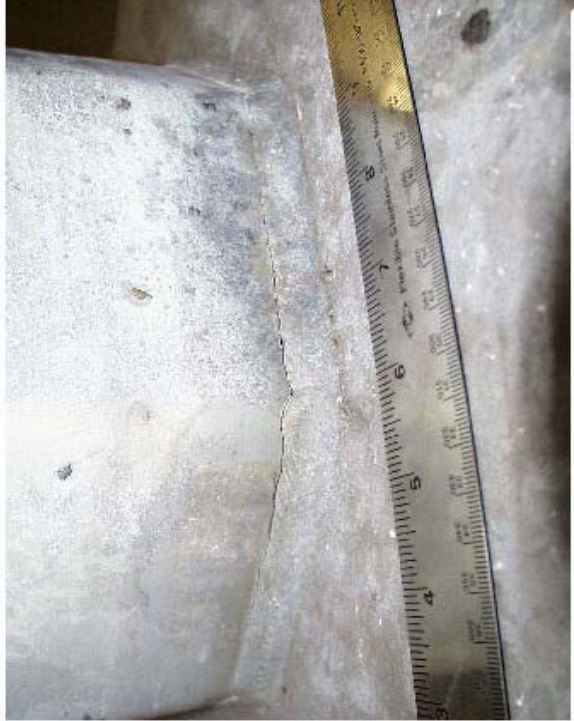
1 Figure2.4 View of the typical outer weld on the luminare stanchion
