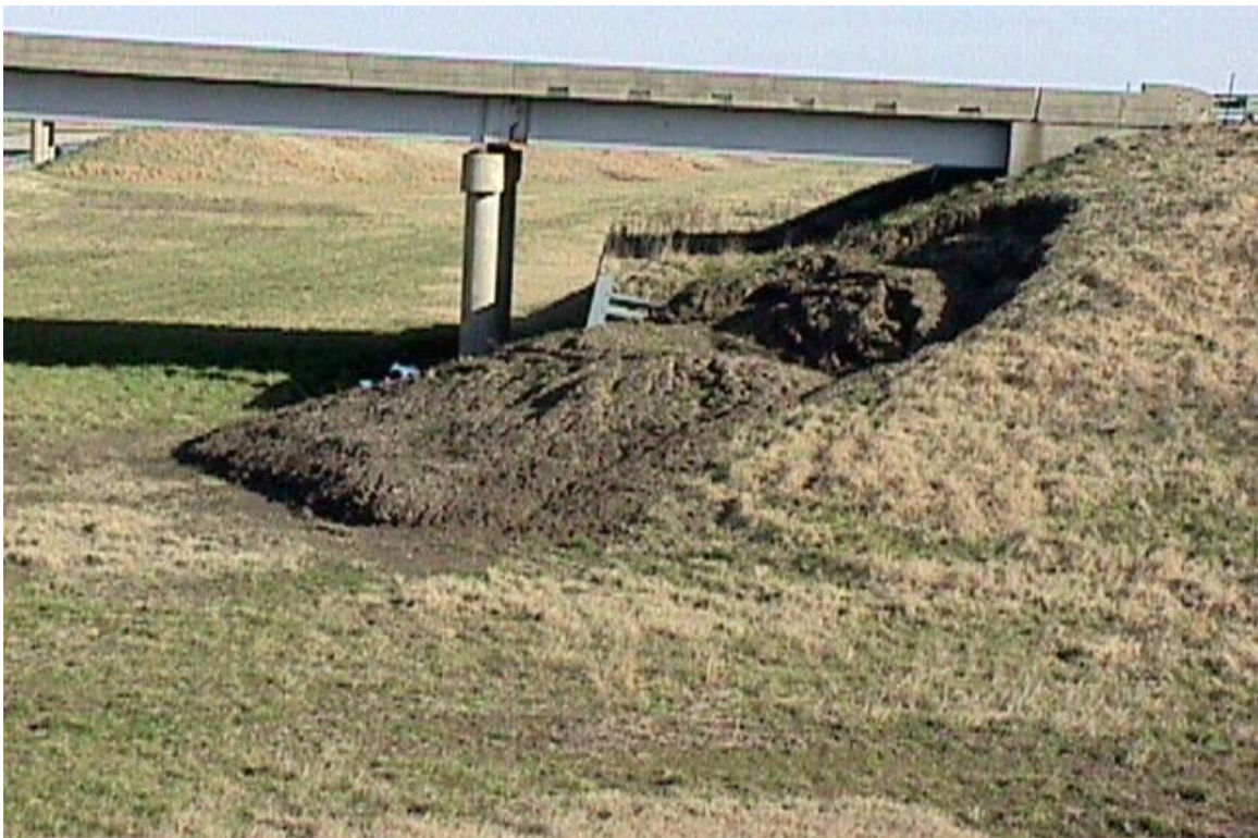
Figure 2. Slope Failure at MM 17 of I-55, North Bound Bridge
