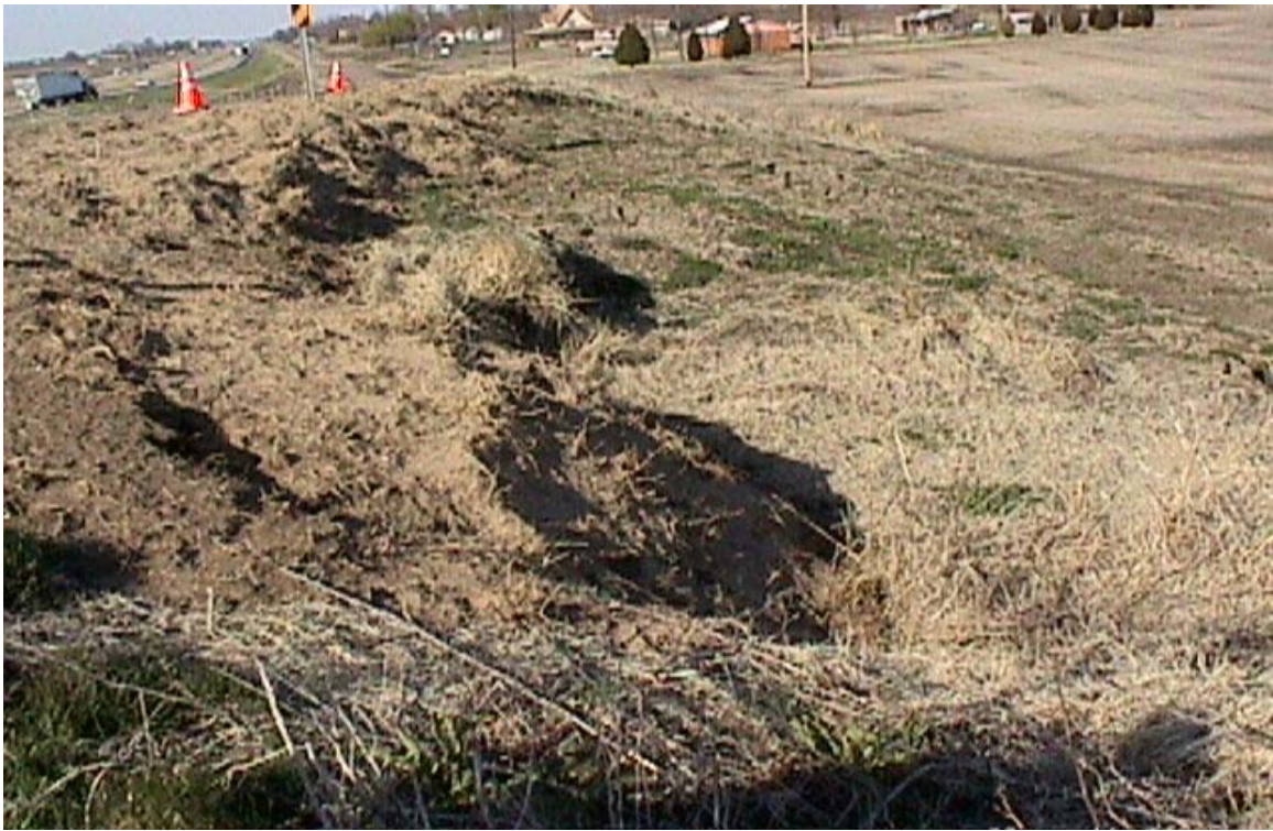
Figure 1. Slope Failure at MM 24 of I-55, East Access Road
