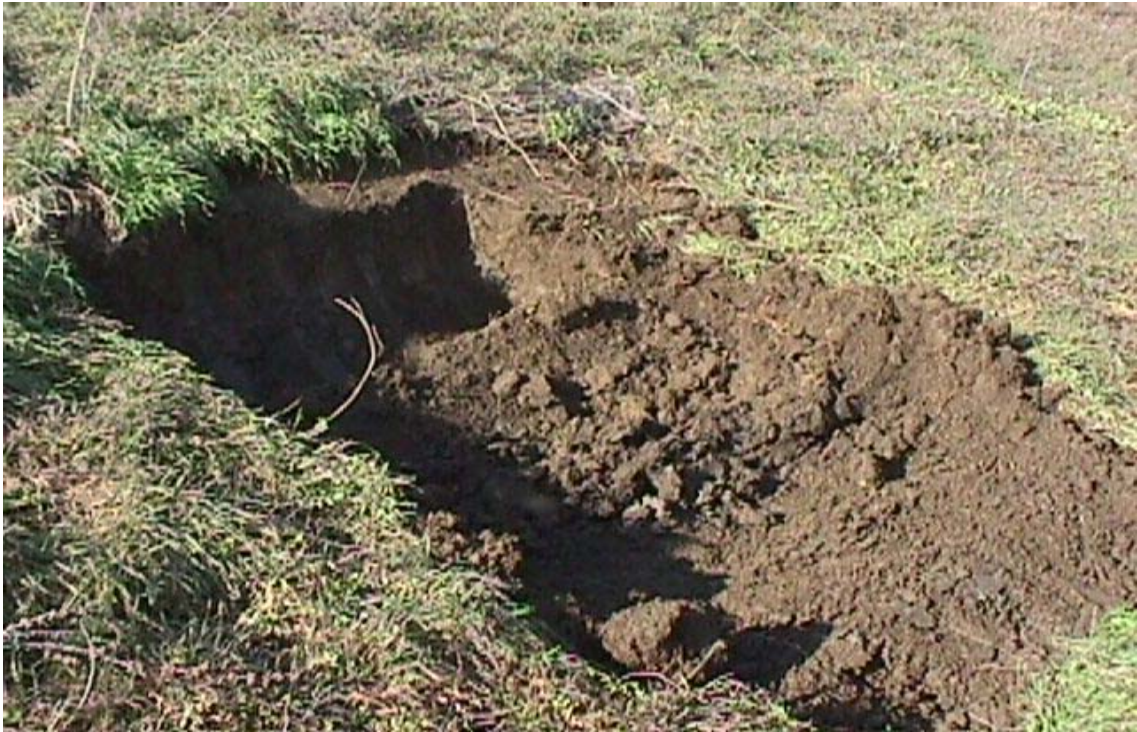
Figure 5. Sampling Trench for Silty Soil at MM 24
