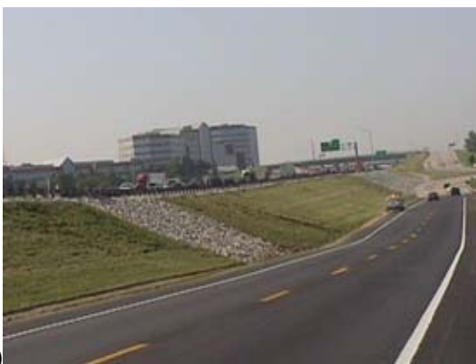
Figure 6 – (a) Repair embankment slide along I-270 and (b) Slide in a cut slope along US-65
