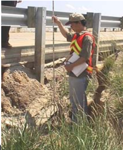
Figure 15 – (a) Erosion at the edge of shoulder concrete on Spencer road ramp on to Mo-370. (b) Erosion problem near I-170 and I-70 intersection.
