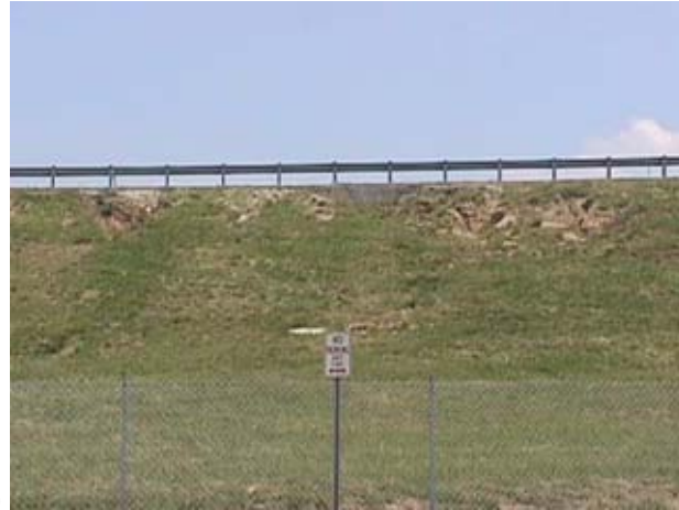
Figure 15 – (a) Erosion at the edge of shoulder concrete on Spencer road ramp on to Mo-370. (b) Erosion problem near I-170 and I-70 intersection.
