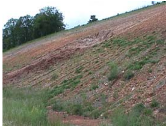
Figure 6 – (a) Repair embankment slide along I-270 and (b) Slide in a cut slope along US-65
