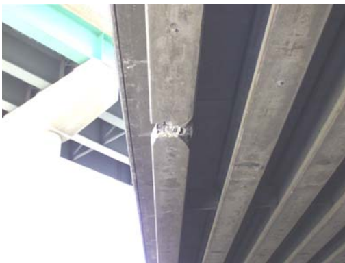
(a) Overall View of the Damage
