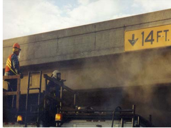
(b) Surface Sandblasting
