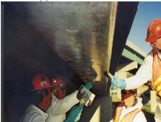
(c) Application of Putty
