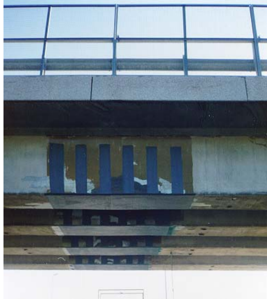
Figure 1.2. Pattern of CFRP Strips
