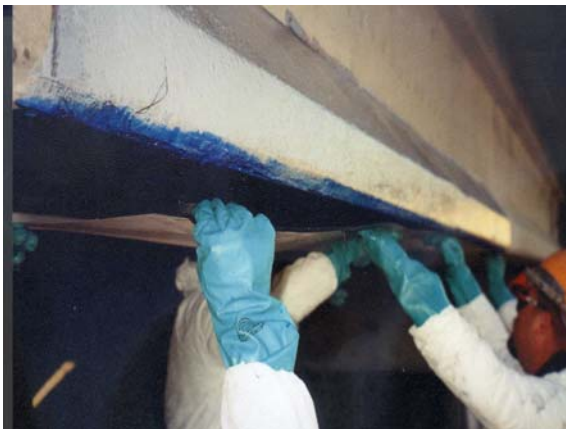
(e) Manual Lay-up of CFRP Sheet
