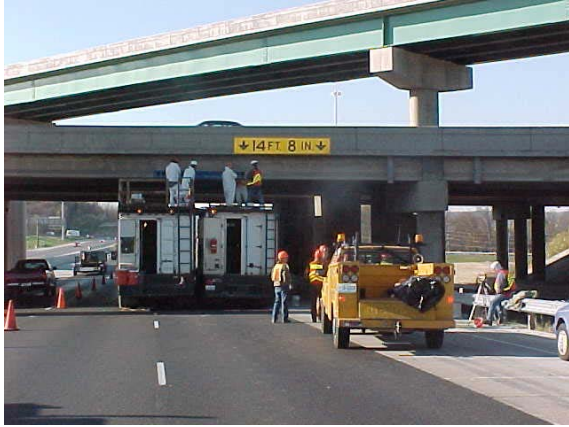
(a) Overall View
