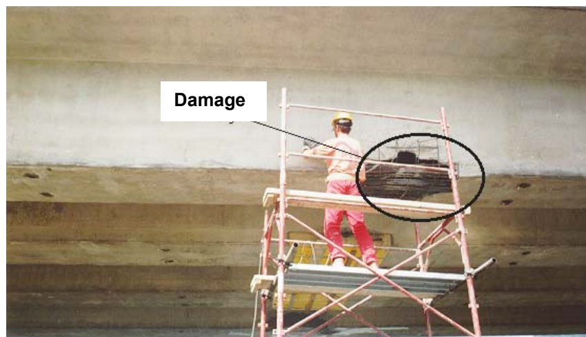
Figure 1.1. Girder Damage due to Vehicular Impact
