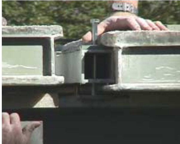
Figure 4.1 Cross Section of Panel Joint and Clamp Assembly – St. Johns Street
