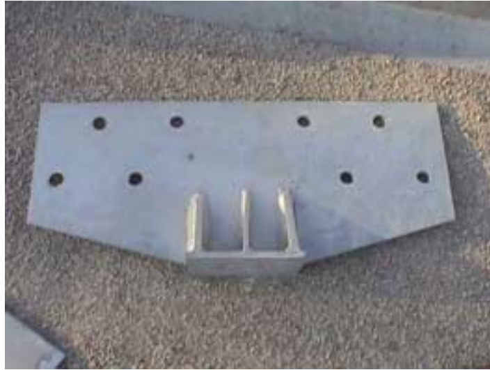
Figure D.19 Steel Plate Utilized to Attach Guardrail Posts to the Panels – St. Francis Street
