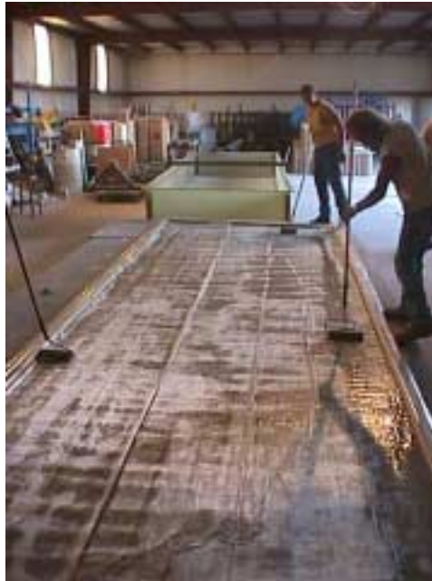
Figure A.2 Manual Lay-up of the Bottom Face
