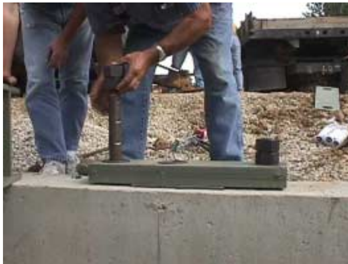
Figure D.2 Installation of the Bearing Pads, Steel Plates and Anchor Bolts – St. Johns and Jay Street
