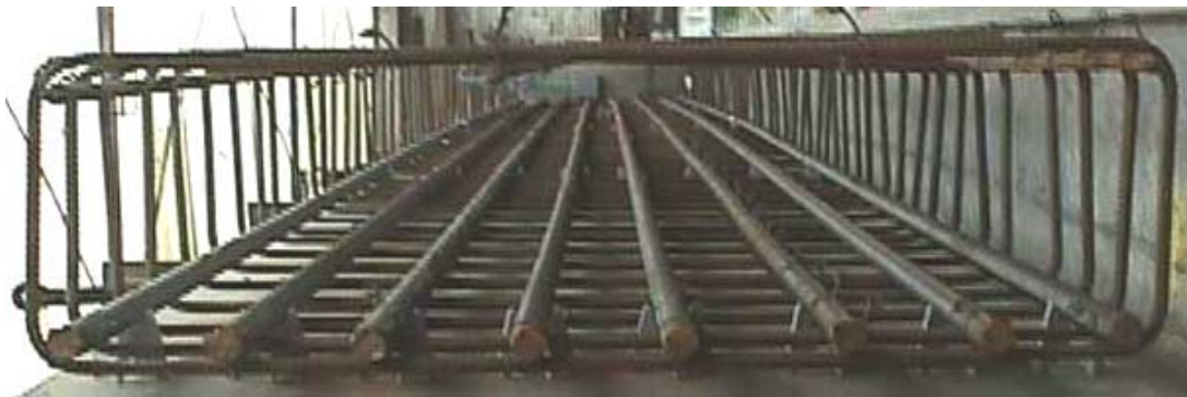
Figure 6.4 Steel Reinforcement Layout
