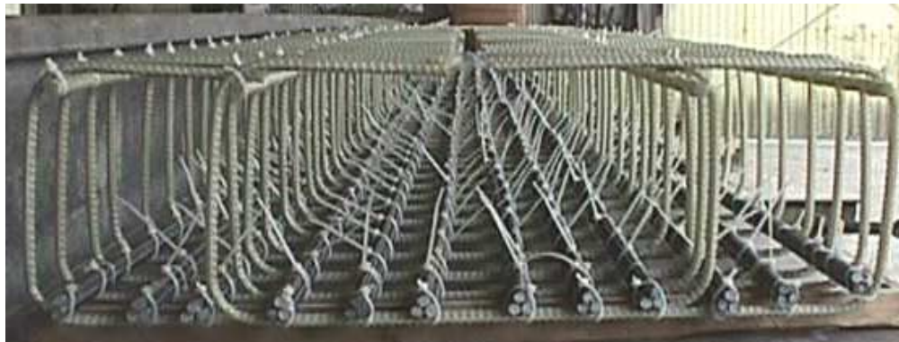
Figure 3.7 FRP Reinforcement Layout
