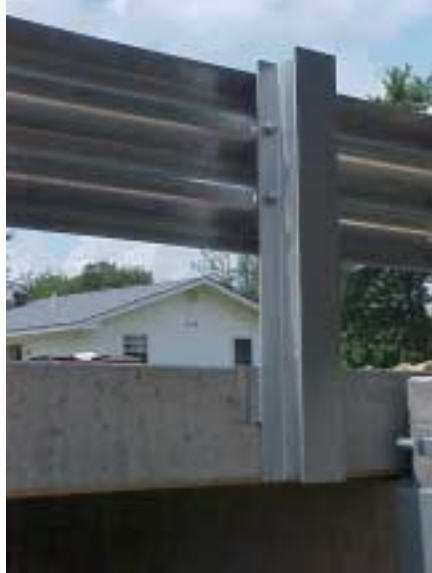
Figure D.25 Installed Guardrail – Walters Street
