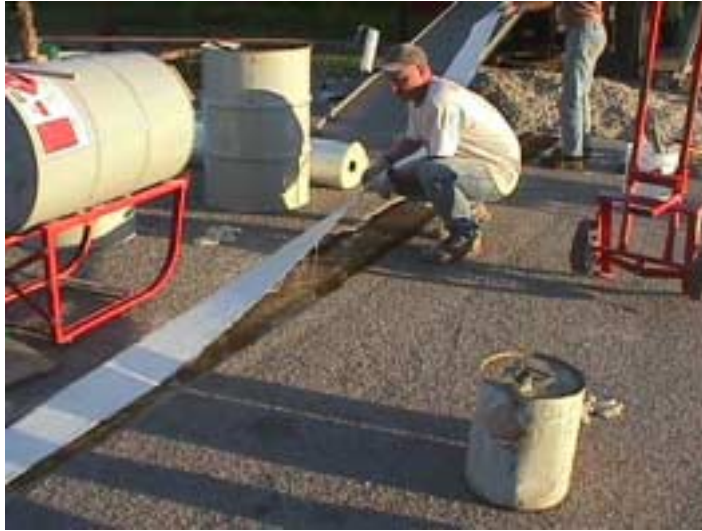
Figure D.15 Lay-up of FRP Layers over the Joint Space – Jay Street
