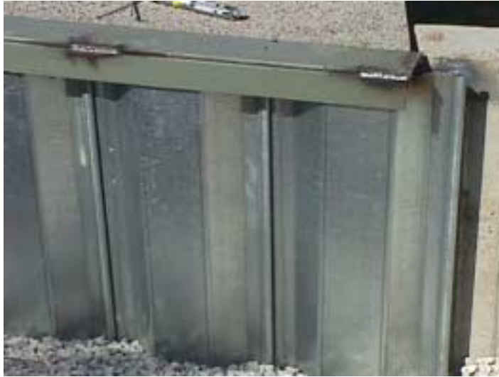
Figure D.13 Completed Abutment Assembly – St. Johns and Jay Street
