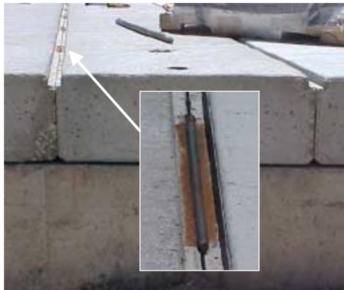
Figure 4.6 Panel Connection Detail
