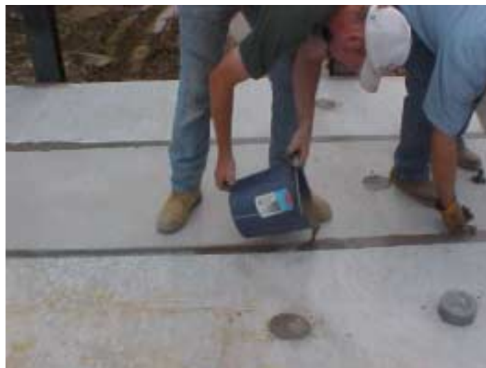
Figure D.24 Filling Panel Joints and Abutment Anchor Holes with Grout – Walters Street
