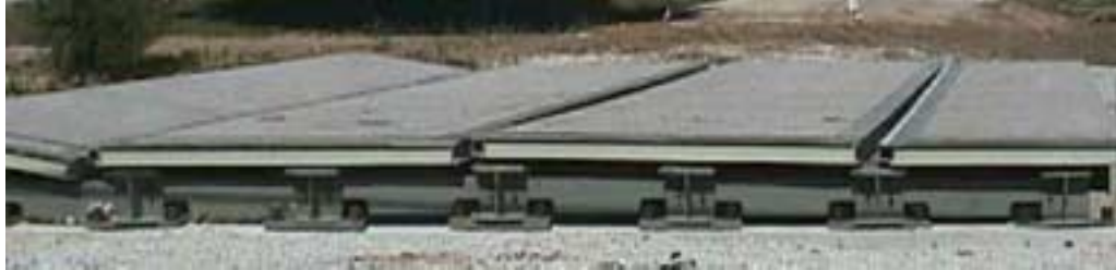
Figure 3.4 Jay Street Bridge Structure
