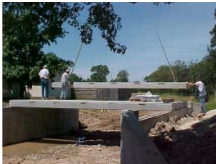
Figure D.22 Setting of the Bridge Panels – Walters Street
