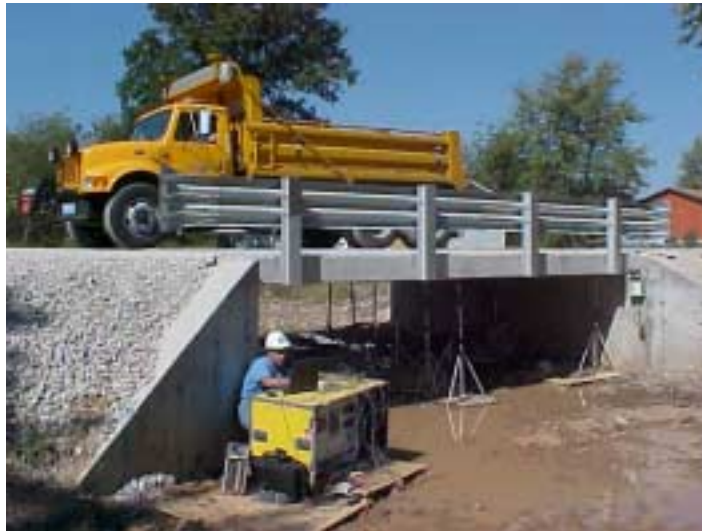
Figure 7.37 In-situ Bridge Load Test – Walters Street
