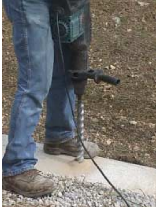
Figure D.1 Drilling of the Holes for the Anchor Bolts – St. Johns and Jay Street
