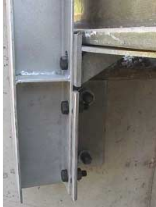
Figure D.21 End Guardrail Post with Additional Connection to the Abutment – St. Francis Street
