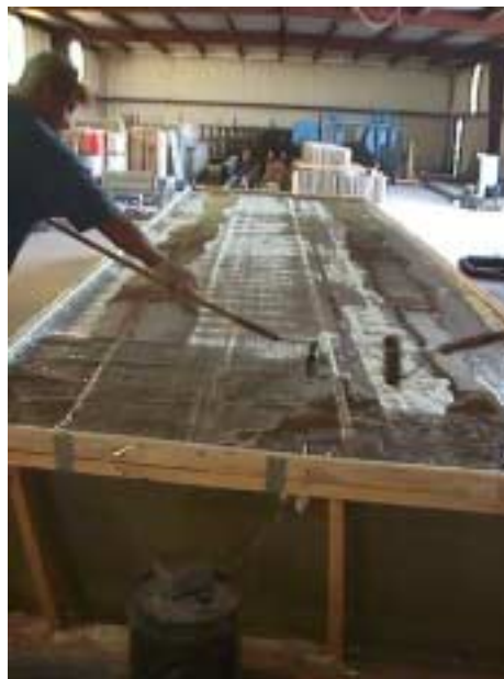
Figure A.6 Manual Lay-up of the Top Face
