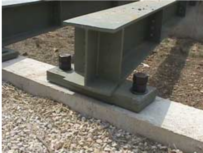
Figure D.3 Installation of the Girders – St. Johns and Jay Street
