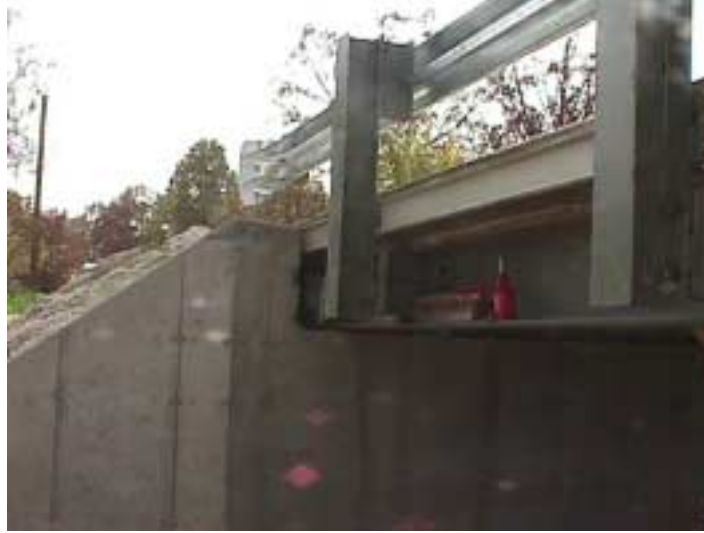
Figure D.17 Guardrails Installed – St. Johns and Jay Street
