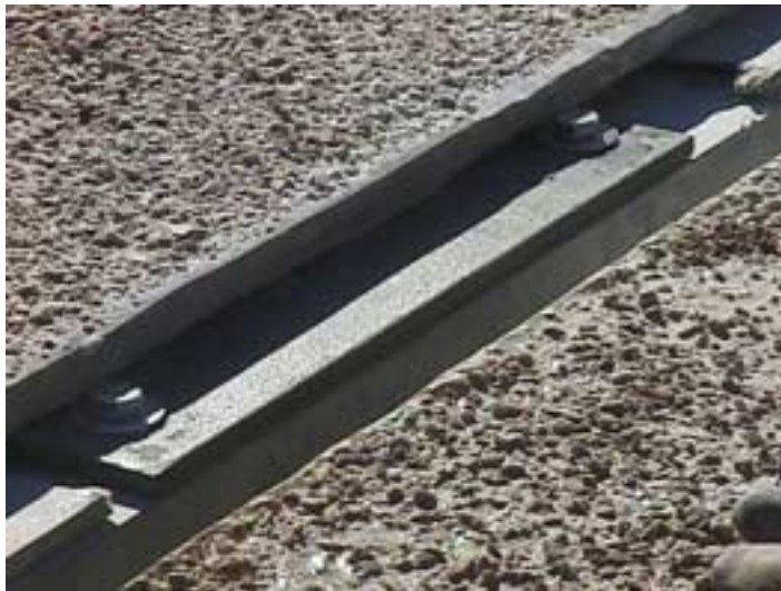
Figure D.8 Top View of Clamping Assembly – St. Johns Street
