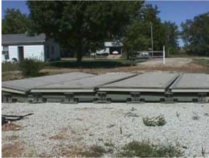
Figure D.7 Setting the Panels onto the Girders– Jay Street
