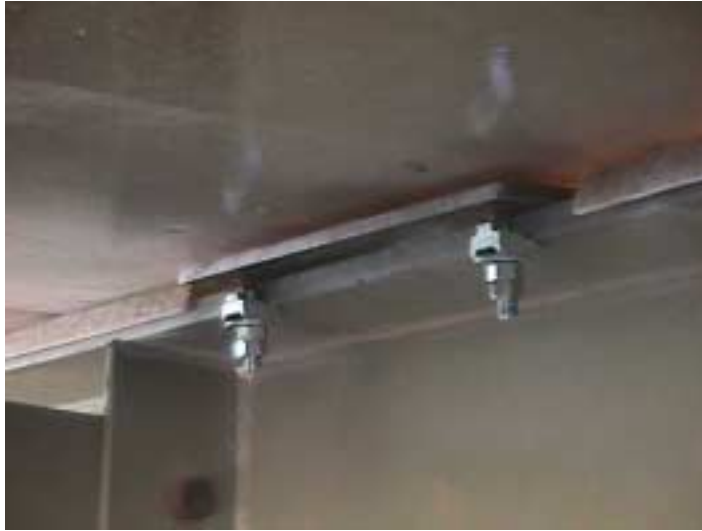
Figure D.11 Underside View of Clamping Assembly– Jay Street
