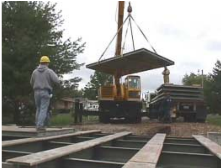
Figure D.6 Setting the Panels onto the Girders– St. Johns Street
