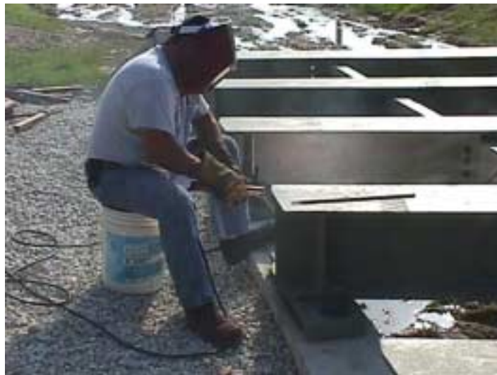
Figure D.4 Welding of the Girders to the Anchored Plates – St. Johns and Jay Street
