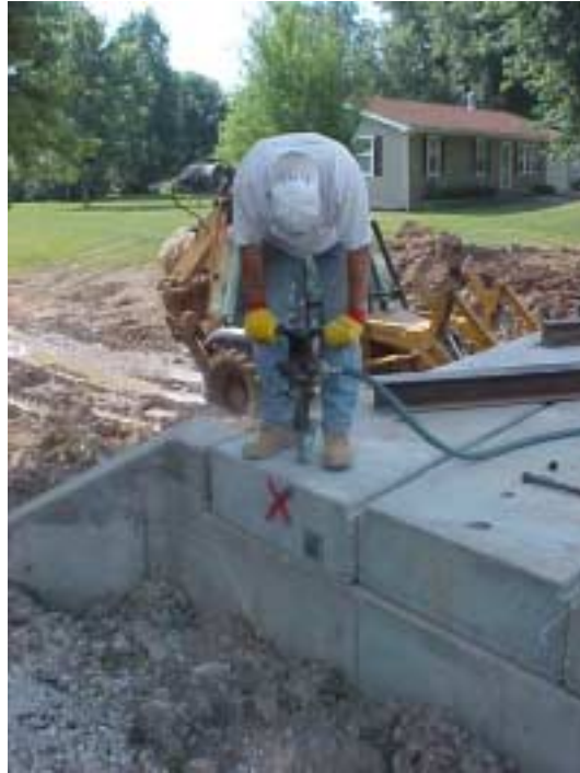
Figure D.23 Drilling Holes to Anchor the Panels to the Abutments – Walters Street
