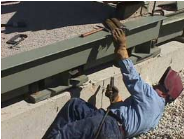
Figure D.12 Connection of the T-beam to the Girders– St. Johns and Jay Street
