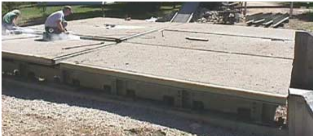
Figure 3.3 St. Johns Street Bridge Structure
