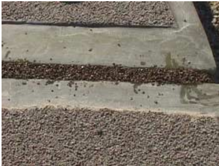
Figure D.14 Filling of Joint Space with Polymer Concrete – St. Johns and Jay Street
