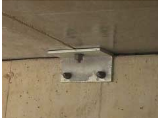
Figure 4.5 Abutment Connection Detail
