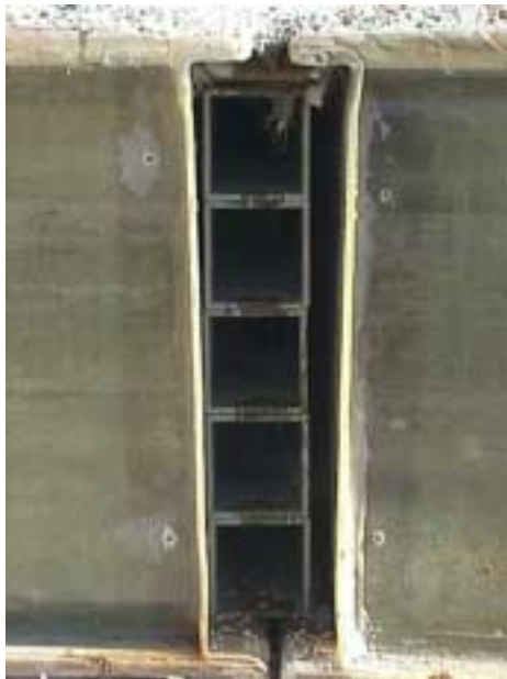
Figure 4.4 Cross Section of the Panel Joint – St. Francis
