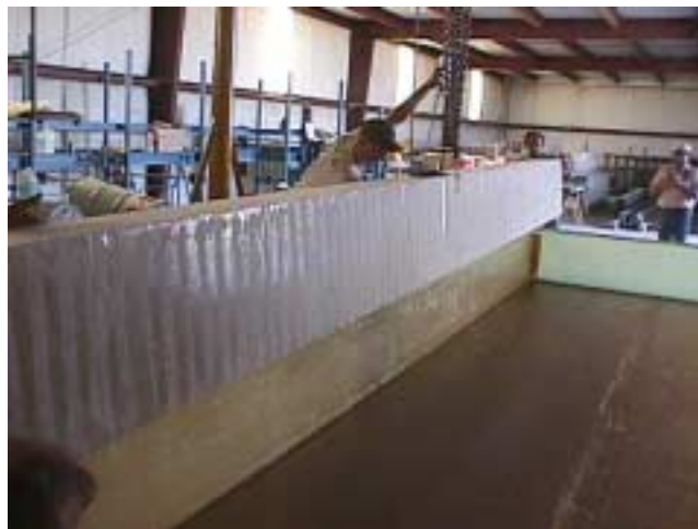
Figure A.4 Installation of the Core Sections
