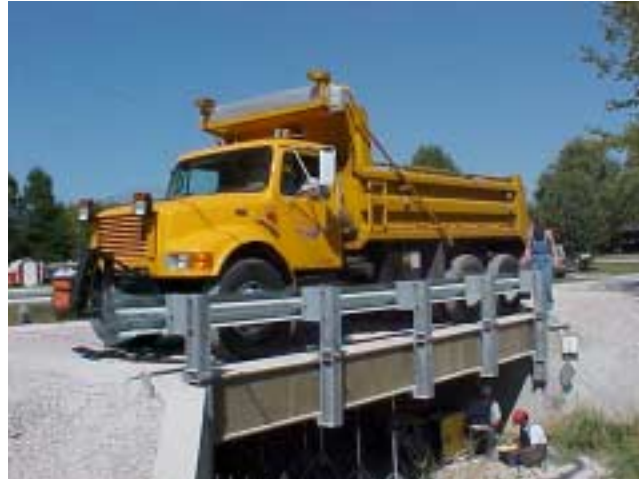
Figure 7.27 In-situ Bridge Load Test – St. Francis Street
