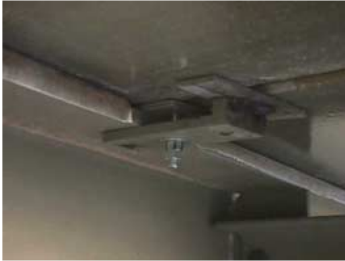
Figure D.9 Underside view of Clamping Assembly– St. Johns Street
