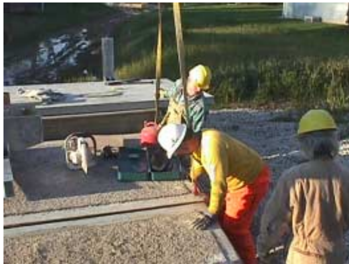
Figure D.18 Setting of the Panels onto the Abutments – St. Francis Street
