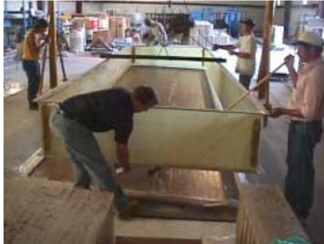
Figure A.3 Installation of the Panel Edges
