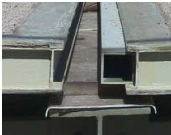
Figure 4.2 Cross Section of Panel Joint– Jay Street
