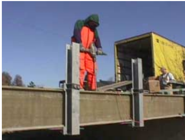
Figure D.20 Drilling Holes through the Deck to Attach the Guardrails to the Panels – St. Francis Street
