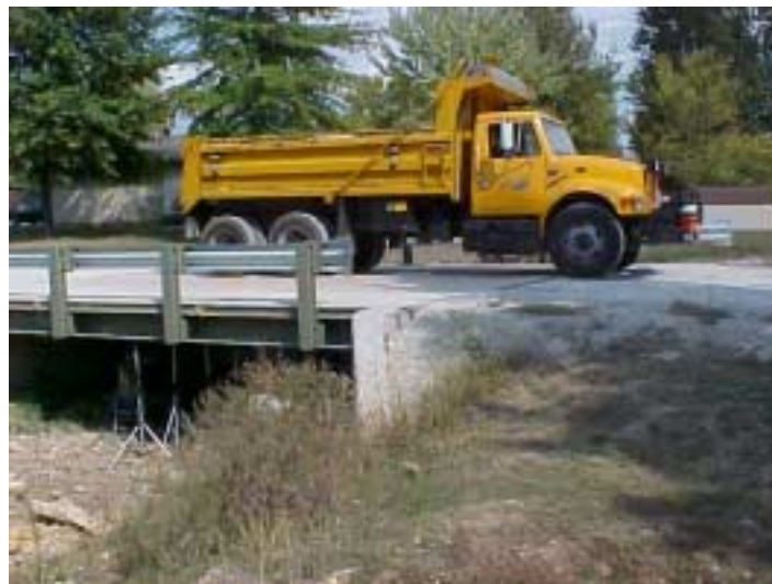
Figure 7.3 In-situ Bridge Load Test – St. Johns Street
