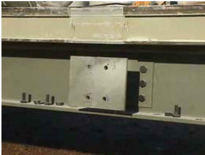
Figure D.16 Spacer Block Between the Girders and the Guardrail Posts – St. Johns and Jay Street
