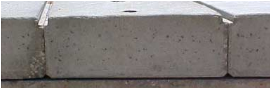
Figure 3.8 Walters Street Bridge Structure
