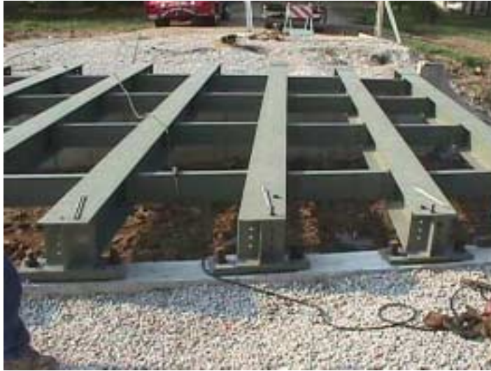
Figure D.5 Installed Steel Diaphragms – St. Johns and Jay Street
