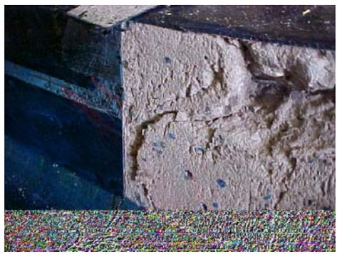
**Figure 6-18: Shear Cracks**
