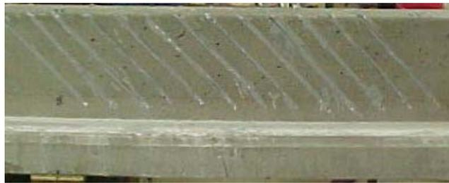
Figure 4-6: NSM Applied to Girder
