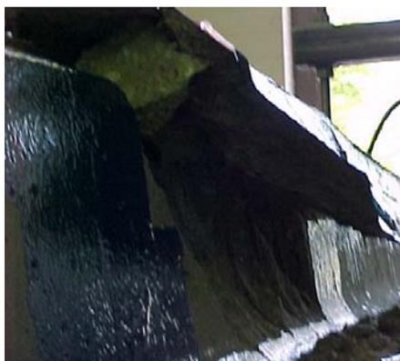
**Figure 6-14: 2-Sufficient Shear Crack at Debond**
