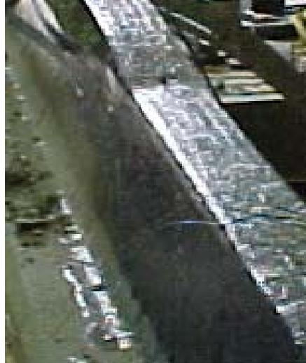
**Figure 6-10: Debond Termination in U-Wrapped Anchored Region**
