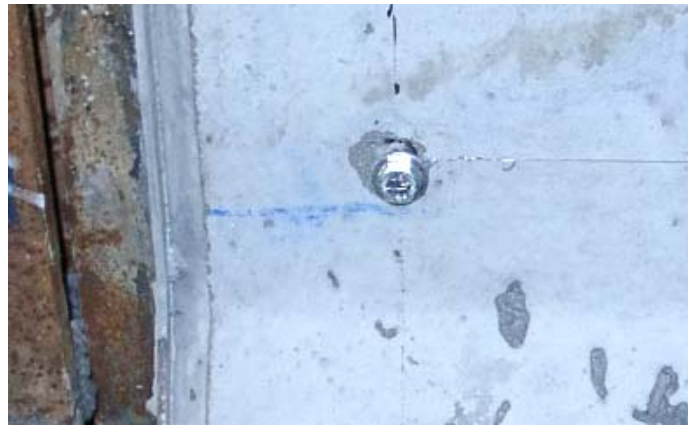
Figure 3.10. Anchor for Tension-Wire System
