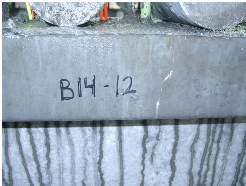
Figure 9.5. Crack After Strands Release
