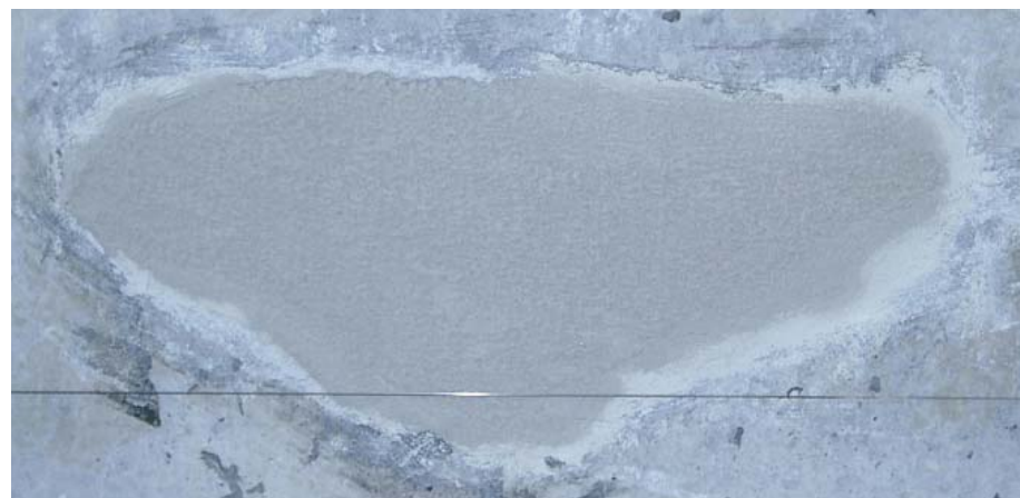
c.) Patched Void
