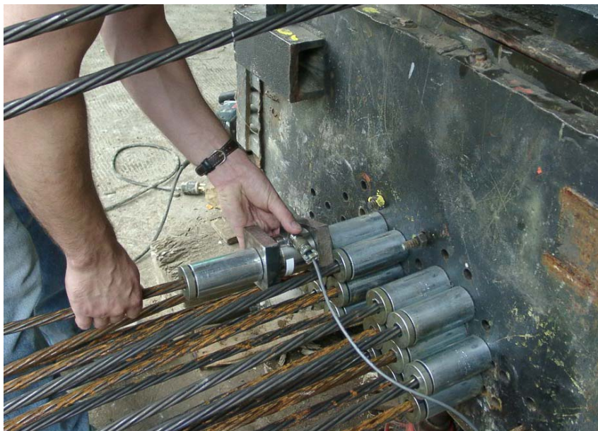
Figure 3.30. Installation of Loadcell
