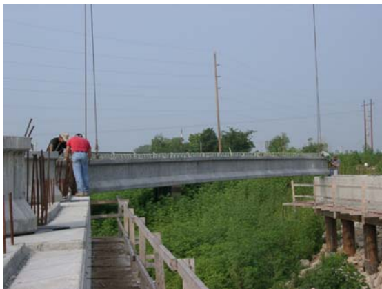
Figure 9.9. Girders on the Bents
