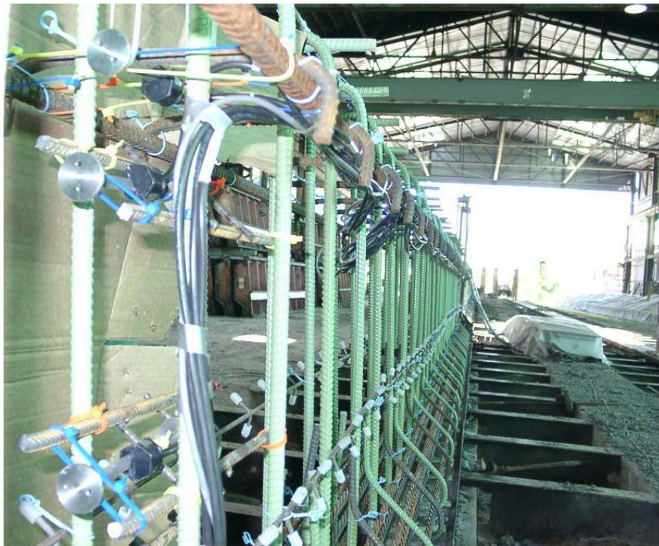
Figure 3.32. Gauges Installed at Designed Locations
