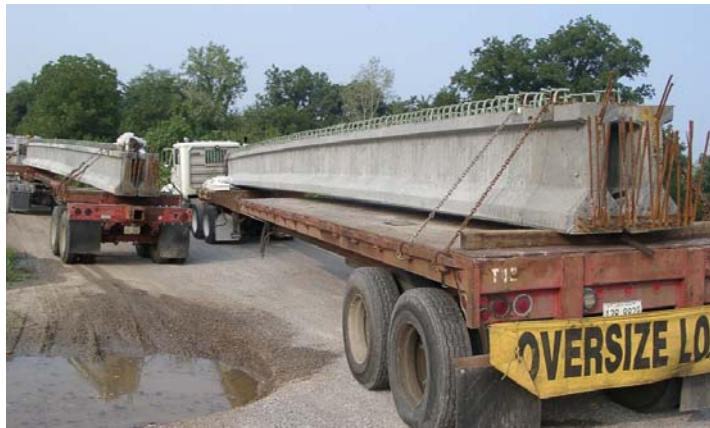
Figure 9.7. Shipping of the Girders to the Bridge Jobsite
