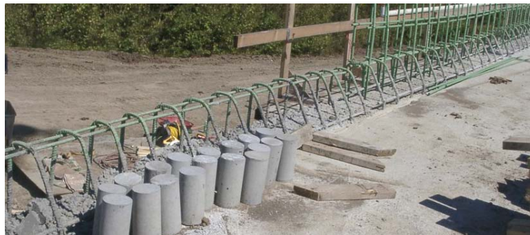
Figure 2.6. Member-Cured Specimens for CIP Deck
