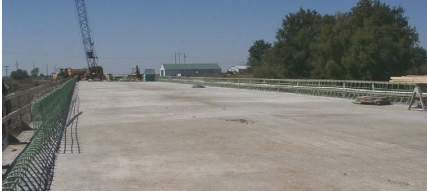
Figure 9.13. Surface of CIP Deck After Wet Mat Curing
