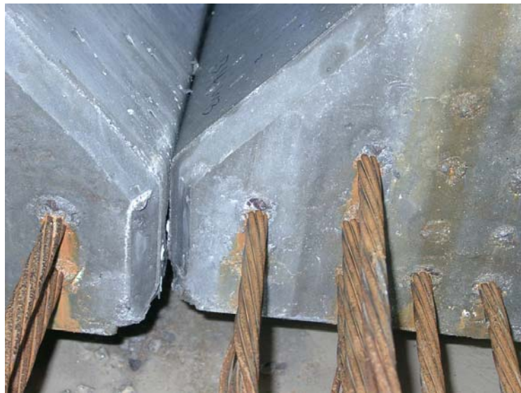
Figure 3.46. Girders Stored in Precast Plant
