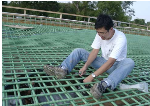
Figure 3.42. Bonding Strain Gauges and Thermocouples to the Steel
