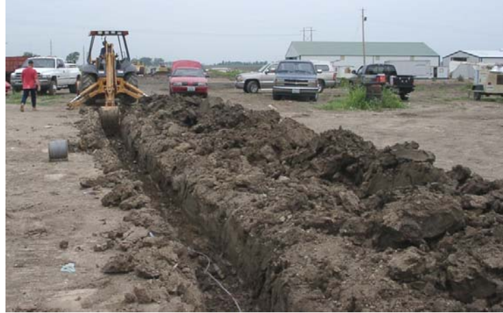
Figure 3.41. Trench Preparation for DAS Power Source
