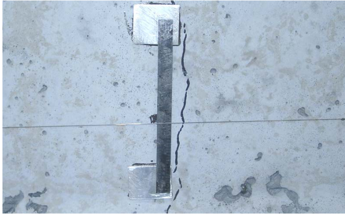
Figure 3.9. Precision Scale for Tension-Wire System
