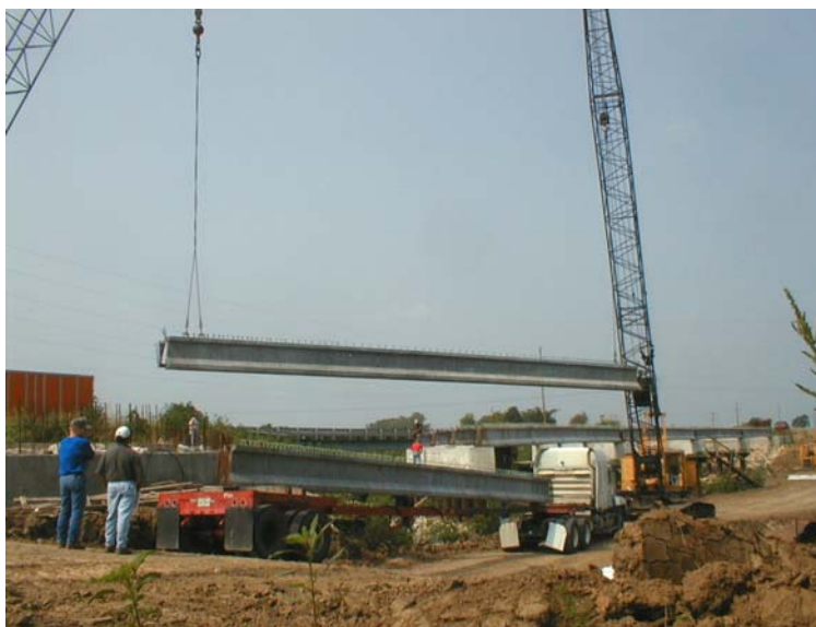
Figure 9.8. Girders Erection
