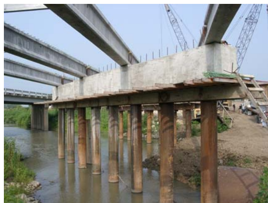
Figure 9.9. Girders on the Bents
