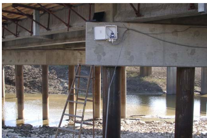
Figure 3.21. Data Acquisition System at Jobsite
