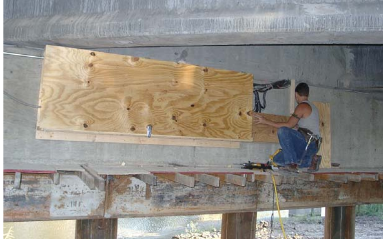
Figure 3.44. Wood Box for DAS
