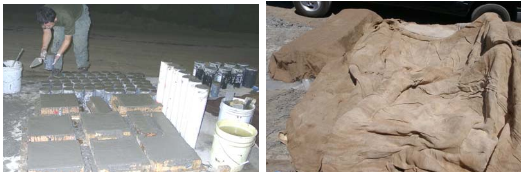
Figure 2.2. Specimens Cast at Bridge Jobsite
