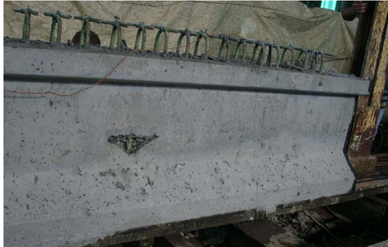
a.) Void Near End of Girder
