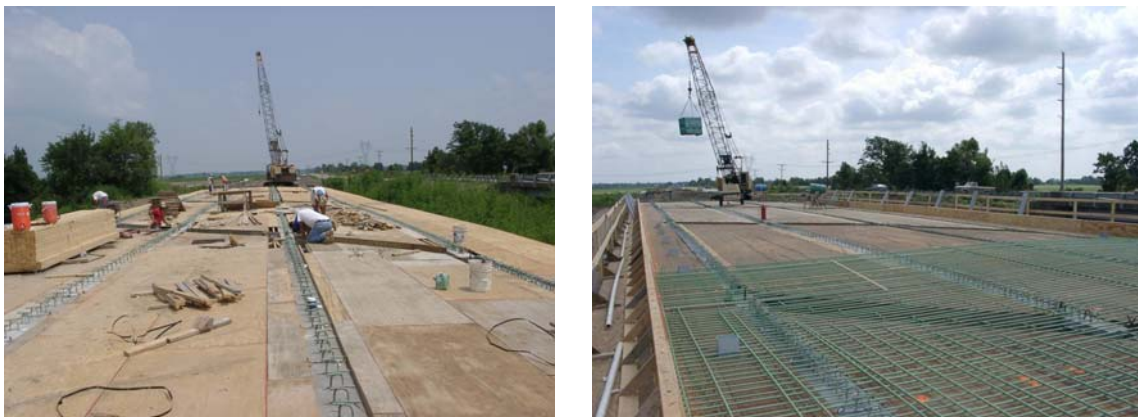
Figure 9.10. Formwork and Steel for the Deck
