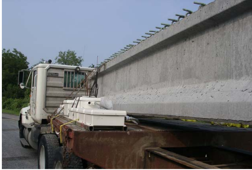
Figure 3.38. Shipping of the Girders to the Bridge Jobsite
