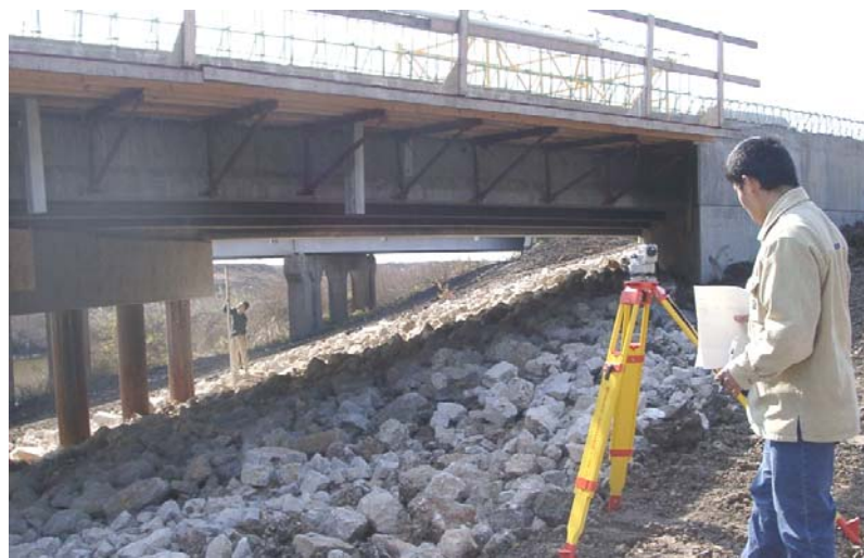
Figure 3.12. Precision Surveying System for Deflection Monitoring before Deck Casting
