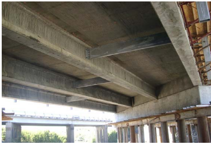
Figure 9.14. Bottom of CIP Deck After Wet Mat Curing
