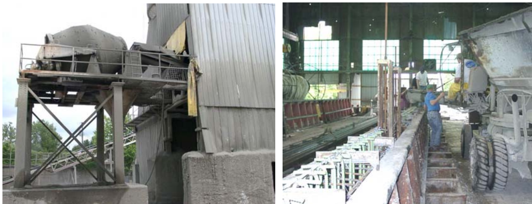
a.) Concrete Mixing
