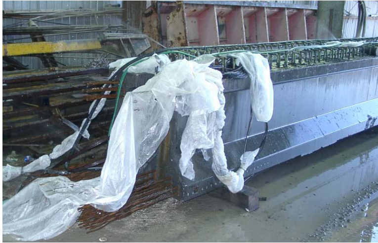
Figure 3.45. Water Curing of the Girders
