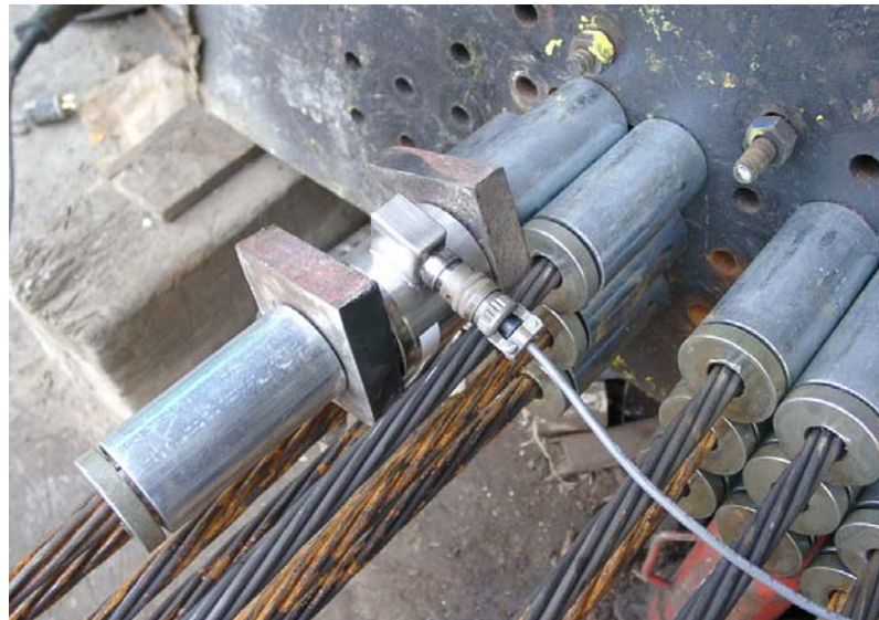
Figure 3.5. Load Cell for Prestress Losses
