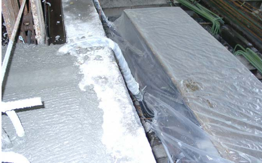
Figure 3.33. Protected DAS during Concrete Placement
