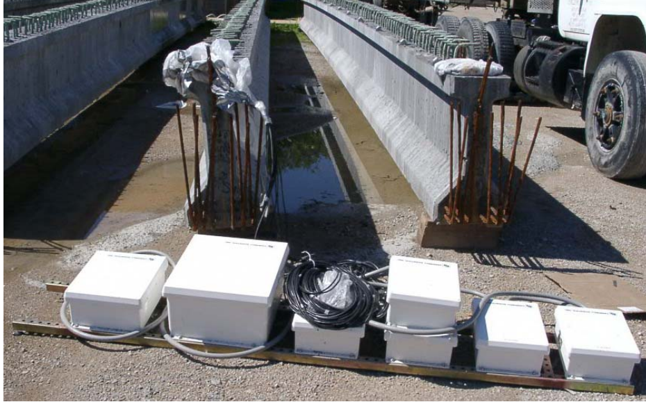
Figure 3.36. Instrumentation When the Girders Were Stored in Precast Plant
