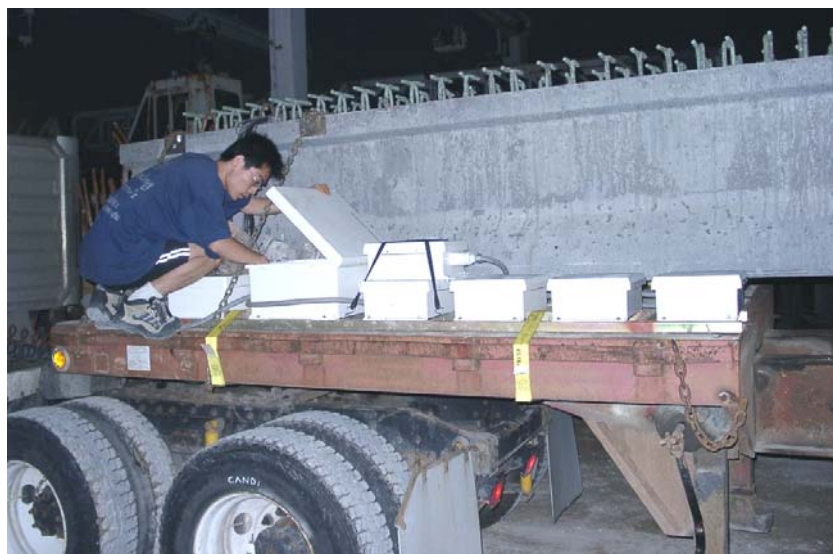
Figure 3.37. Preparing for Shipping of the Girders to the Bridge Jobsite
