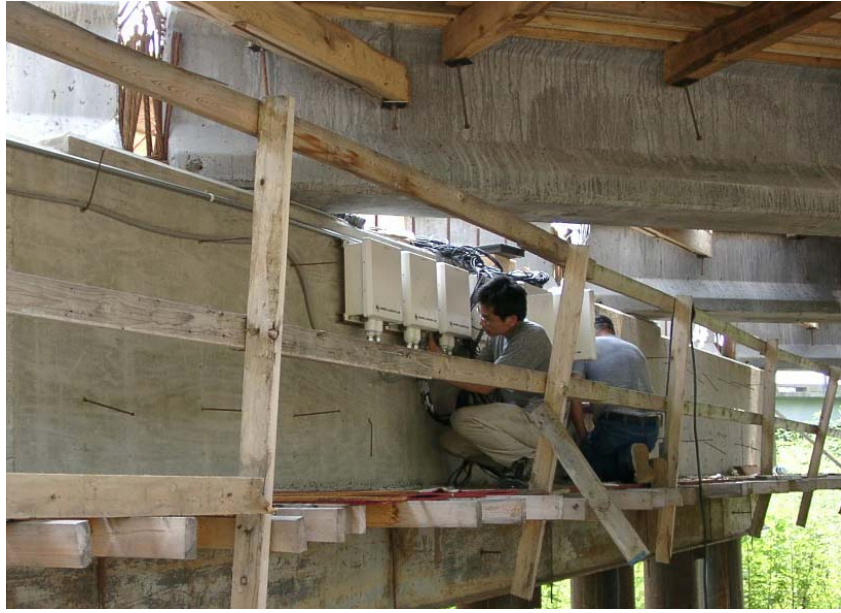
Figure 3.39. Data Reading for Girders and Deck with DAS
