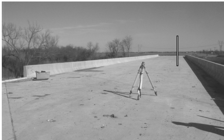
Figure 3.13. Precision Surveying System for Deflection Monitoring after Deck Casting
