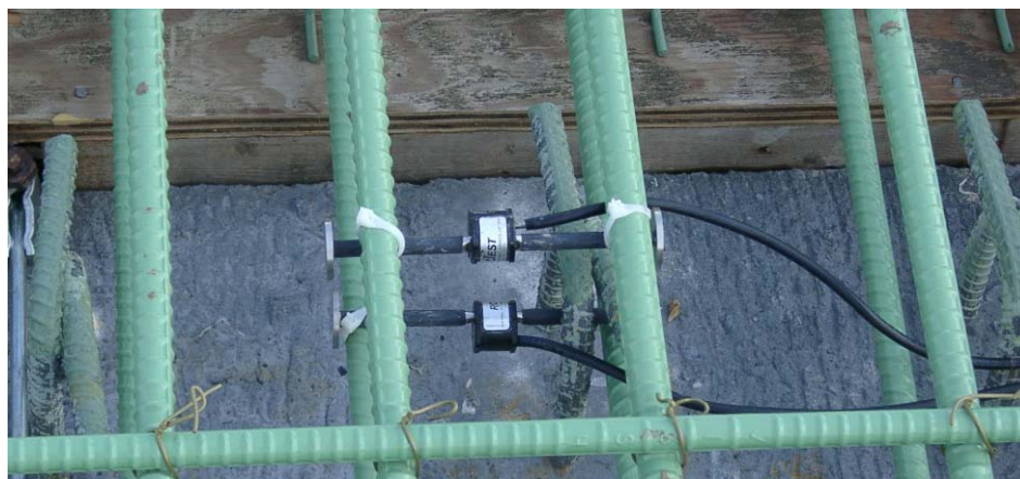
Figure 9.11. Sensors Embedded in the DECK
