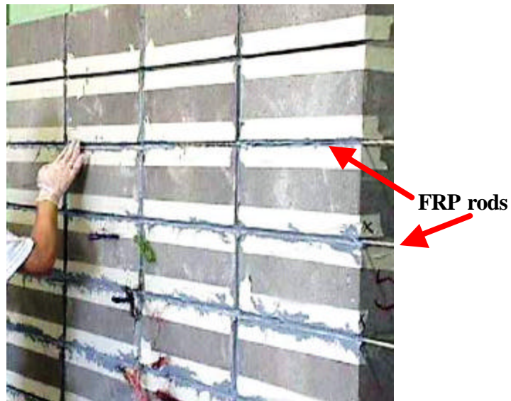
Figure 2: FRP installation for structural repointing in masonry walls
