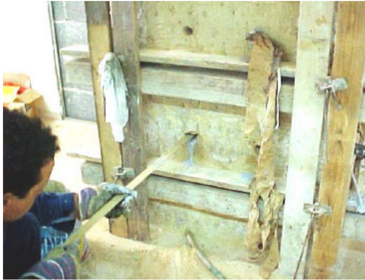
Figure 3: Column confinement with AFRP rods
