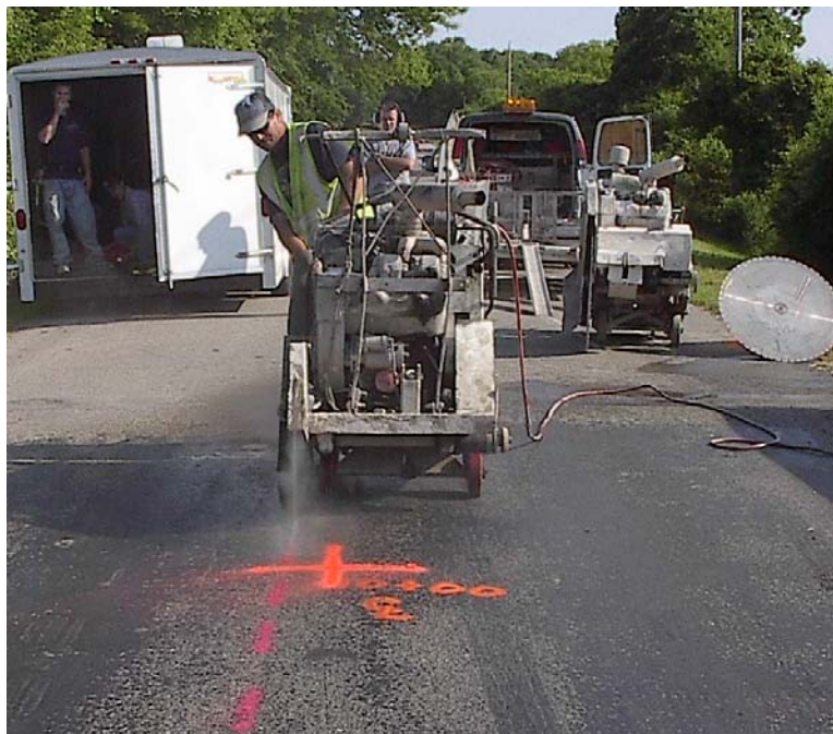
Figure 6.1. Contractor cutting the bridge deck (Cut #1)
