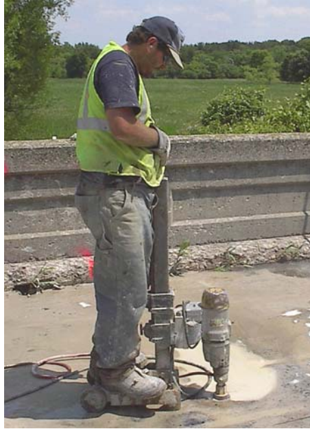
Figure 6.6. Contractor drilling through depth of bridge deck
