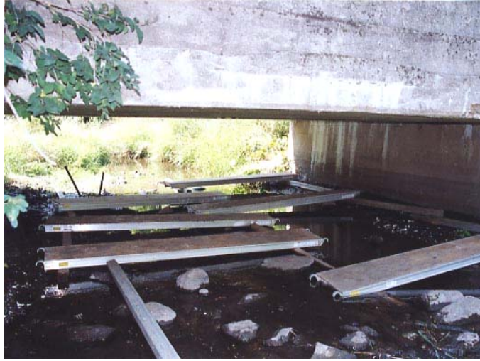
Figure 4.17. Working platform under the bridge
