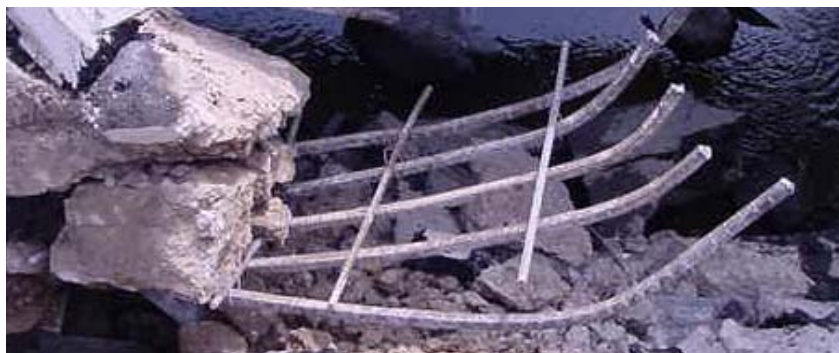
Figure 6.26. View of flexural steel spaced six inches on center
