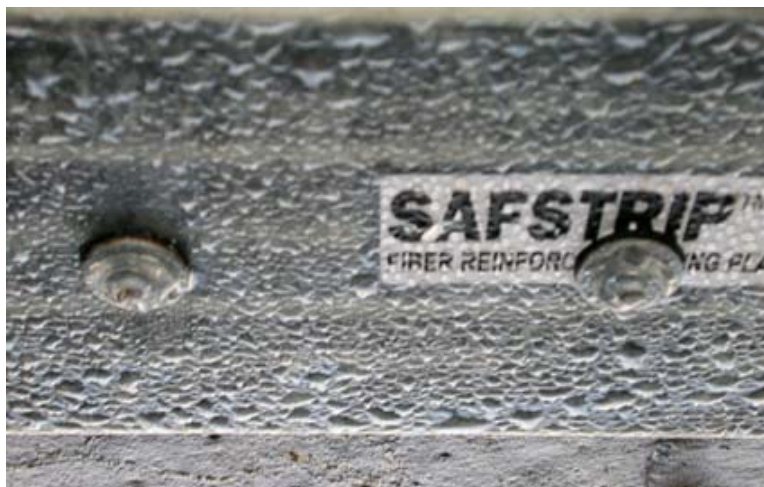
Figure 6.37. FRP strips covered with moisture (spring, 2003)
