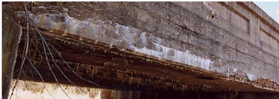
Figure 4.5. Stalactites and efflorescence seen on the underside of the slab of P-53-702
