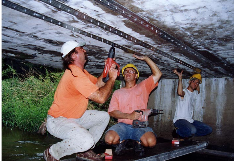
Figure 4.21. Fastening of the FRP strip at the midspan
