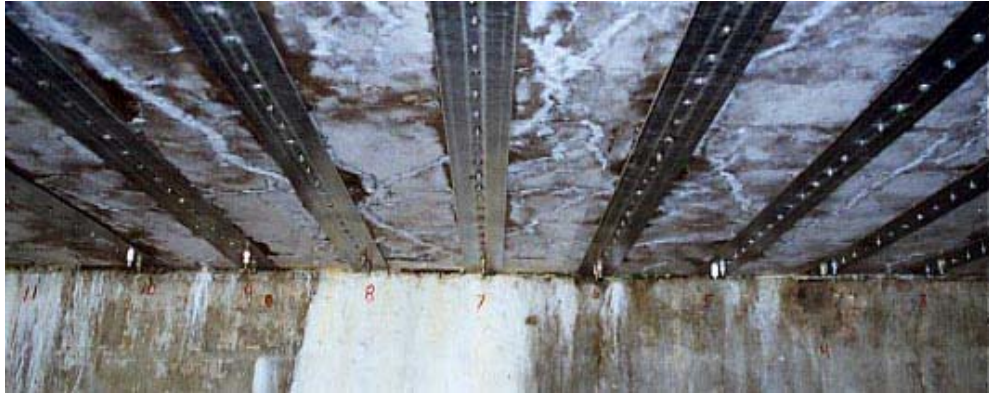
Figure 4.25. 12 in. Strip spacing between FRP strips
