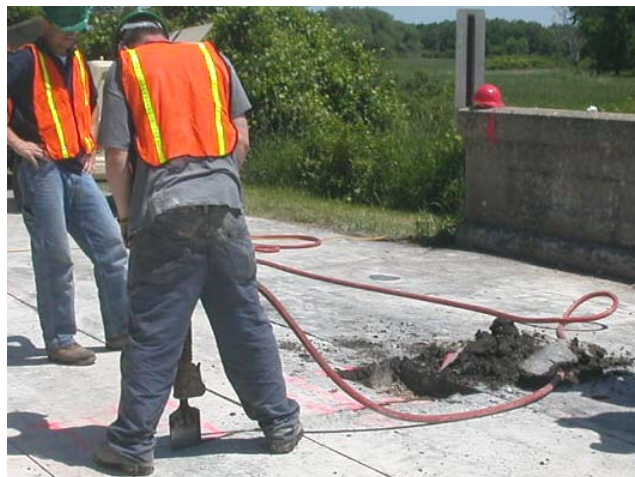
Figure 6.7. Removing the asphalt overlay
