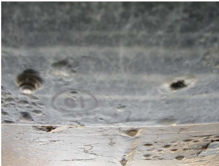
Figure 6.44. Deterioration of FRP strip at location of missing fastener
