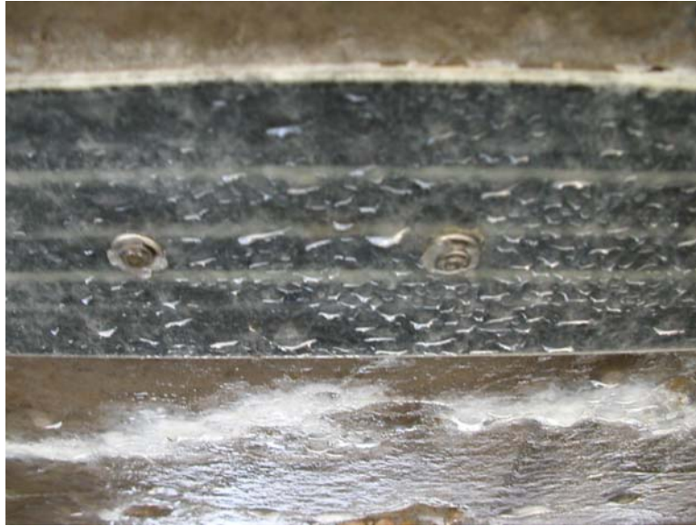
Figure 6.45. Edge of FRP strips covered with water
