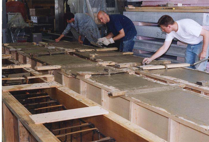
Figure 5.5. Finishing of the concrete
