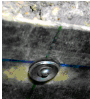
Figure 4.28. Over-driven fastener in the FRP strip
