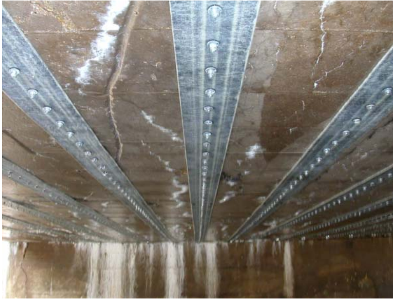
Figure 6.36 Overall view of the retrofitted bridge deck after ten months
