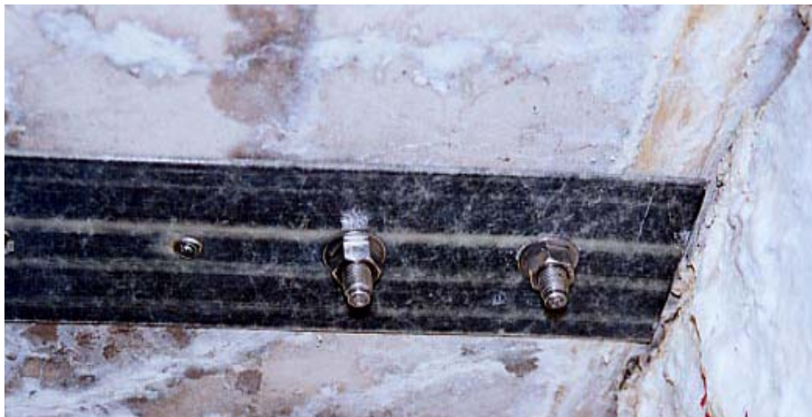
Figure 4.24. Installed end anchor next to the abutment
