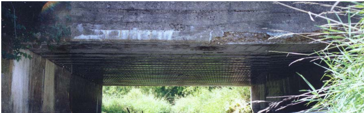
Figure 4.26. Bridge P-53-702 strengthened using MF-FRP system
