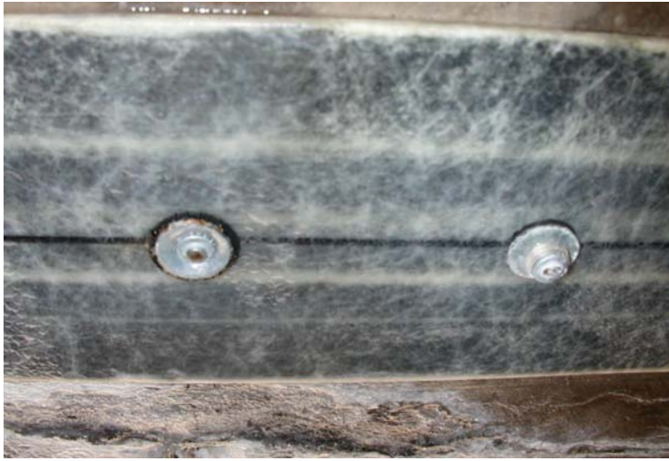
Figure 6.38. Small amount of corrosion seen at the southern end
