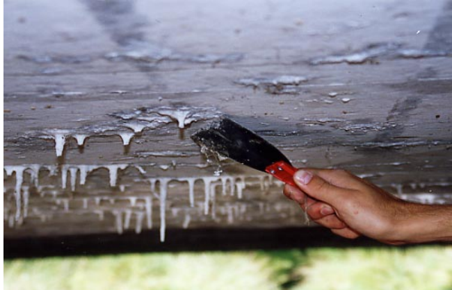
Figure 4.19. Surface preparation of the concrete prior to application of FRP strips
