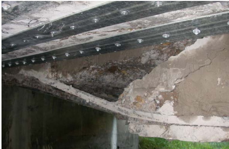
Figure 6.19. Shear failure and spalling along southeast portion of west section
