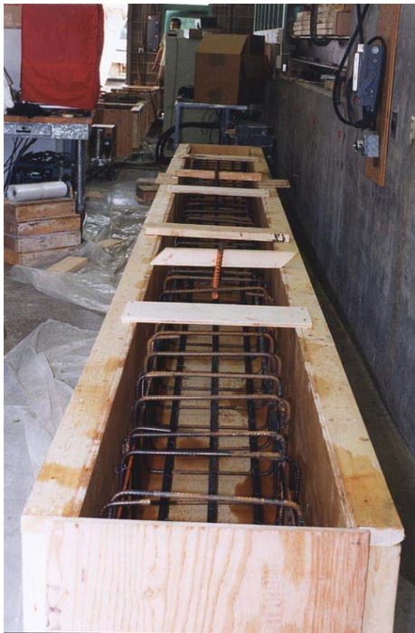
Figure 5.3. Formwork and reinforcement cages
