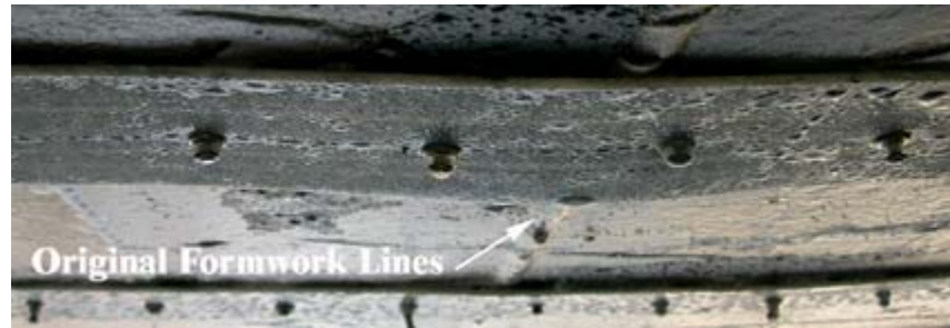
Figure 4.31. FRP strips fastened over original formwork lines
