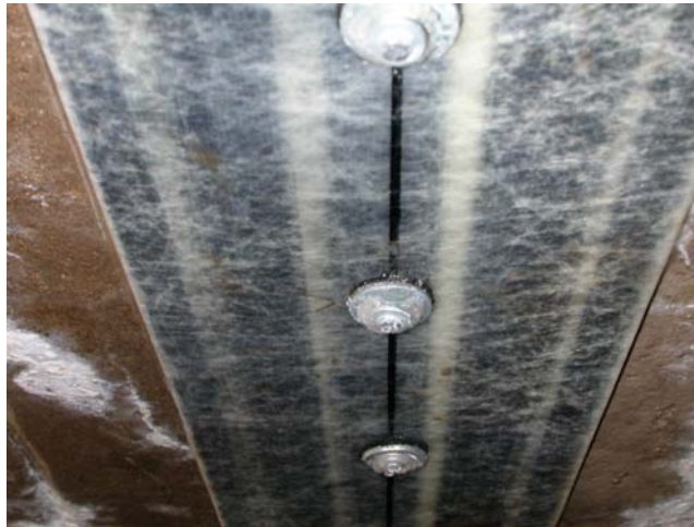
Figure 4.22. Properly installed ALH fasteners at the midspan
