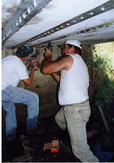
Figure 4.23. Simultaneous drilling and fastening of the FRP strip
