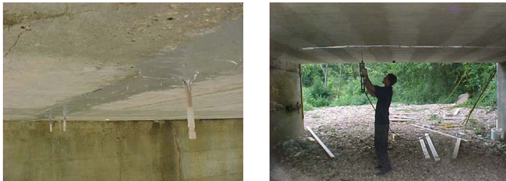
a) Crack Sealed Previous to Injection b) Crack Injection under the Bridge
