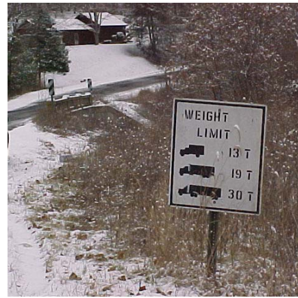
b) Load Posting Prior to Strengthening
