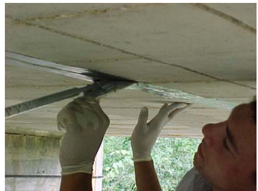
b) Inserting Epoxy Paste into the Groove
