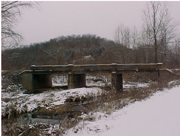
a) Side-view of the Bridge
