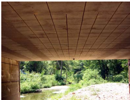
a) Grooves Prepared as per Design Geometry
