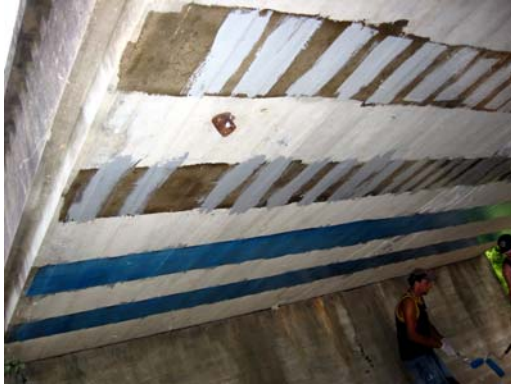
a) Surface Preparation with Primer and Putty
