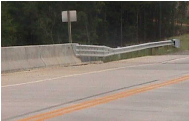
Figure 1.1- Br. A5934, Rte. 21 Crossing the Little Black River in Southeast Missouri.
