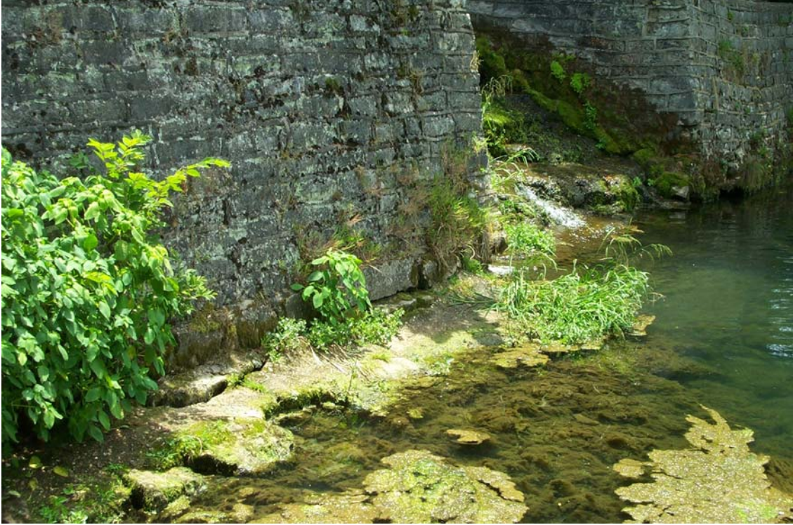
Figure 14: Toe of Dam near Double spillway.
