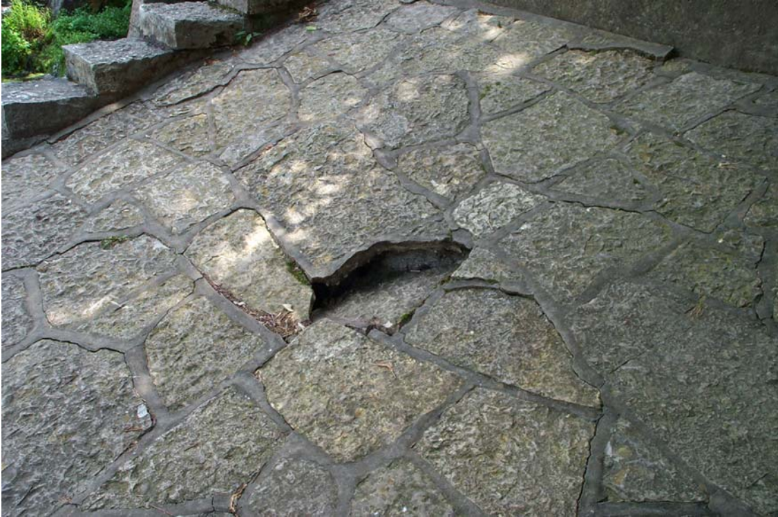
Figure 12: Interior erosion near double spillway.
