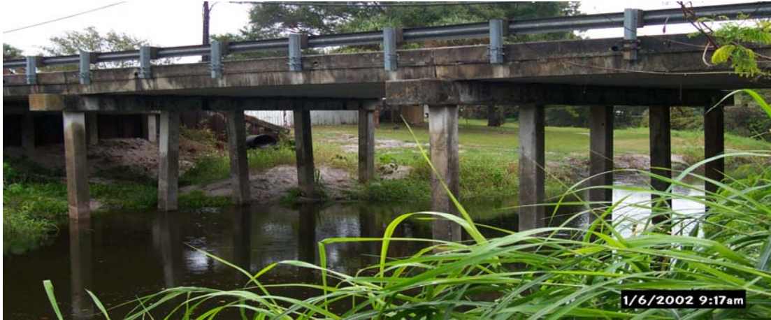
(a) Original Bridge
