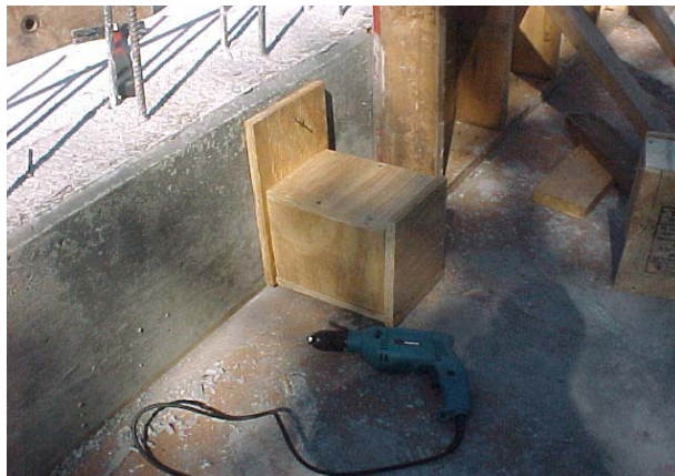
(b) Box housing cables
