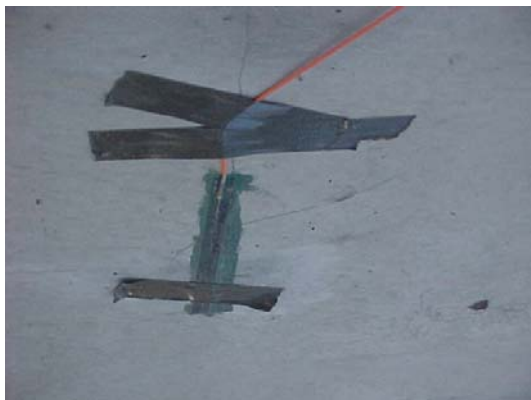
FIGURE 9 Surface-mounted sensors on bottom deck
