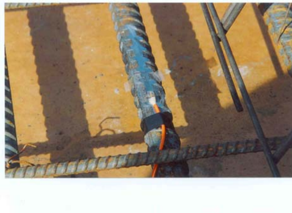
(b) Sensor bonded to rebar
