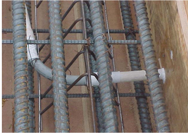
(a) Cable safely moved out of deck
