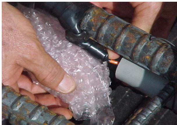
(b) Sensor wrapped in Nitrite rubber
