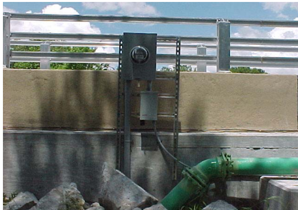
(c) Electric meter and disconnect
