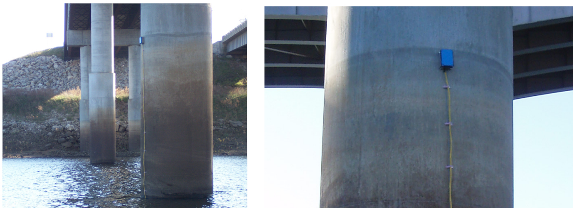
Figure 5. Installation of the Flood Frog on Bridge A6531 in Osage Beach, MO.
