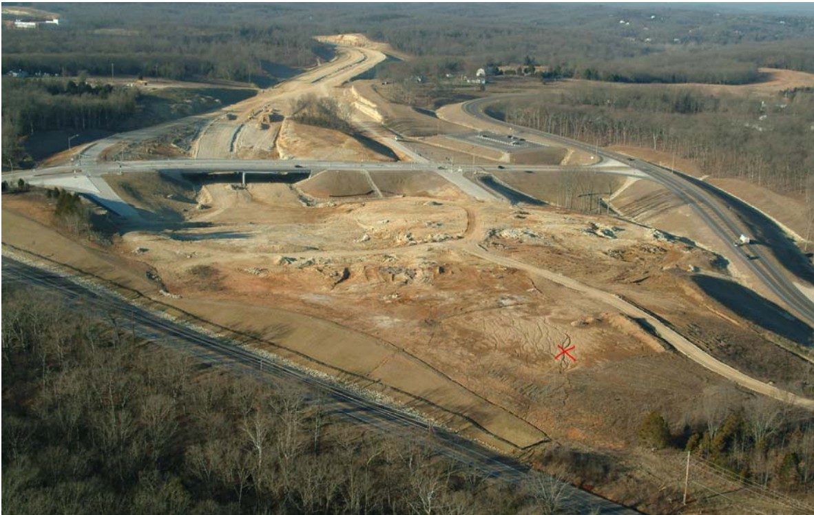
Figure 11: Aerial photograph of the Jefferson County site, prior to the “emptying” of the sinkhole. The approximate location of the sinkhole has been superposed on the photograph.
