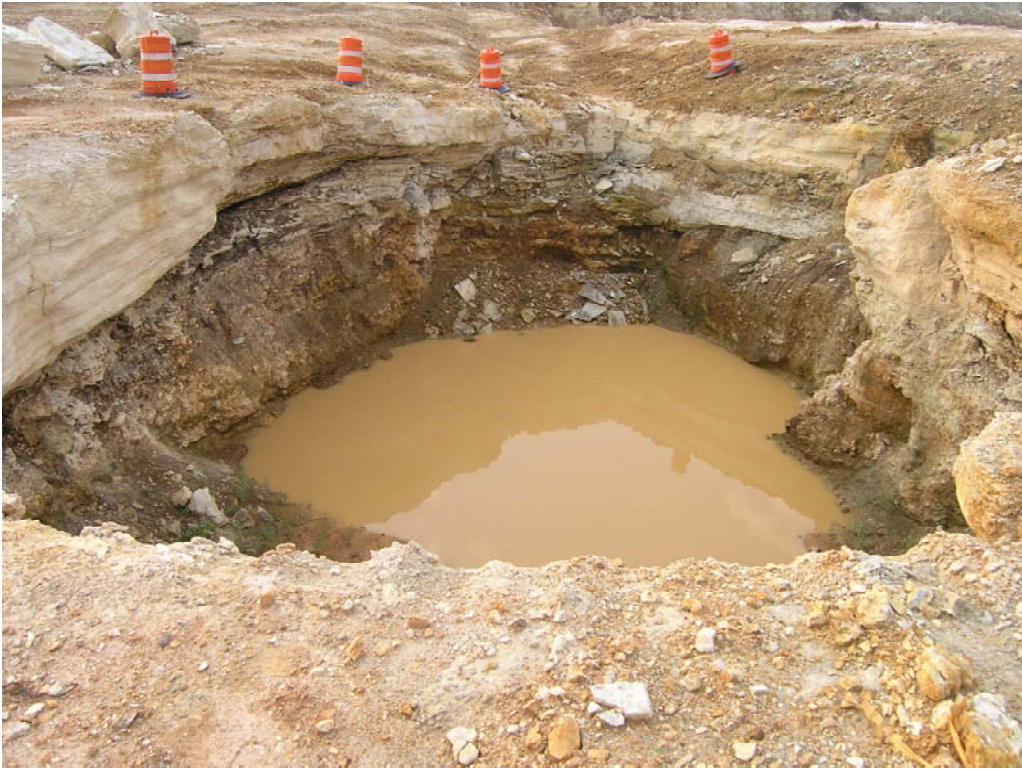
Figure 12: Photograph of the sinkhole, taken from a location immediately to the south of the feature.
