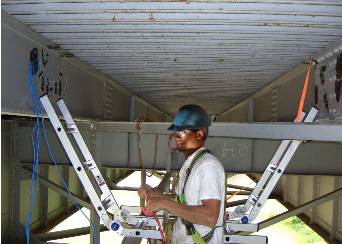
Strain gage installation.
