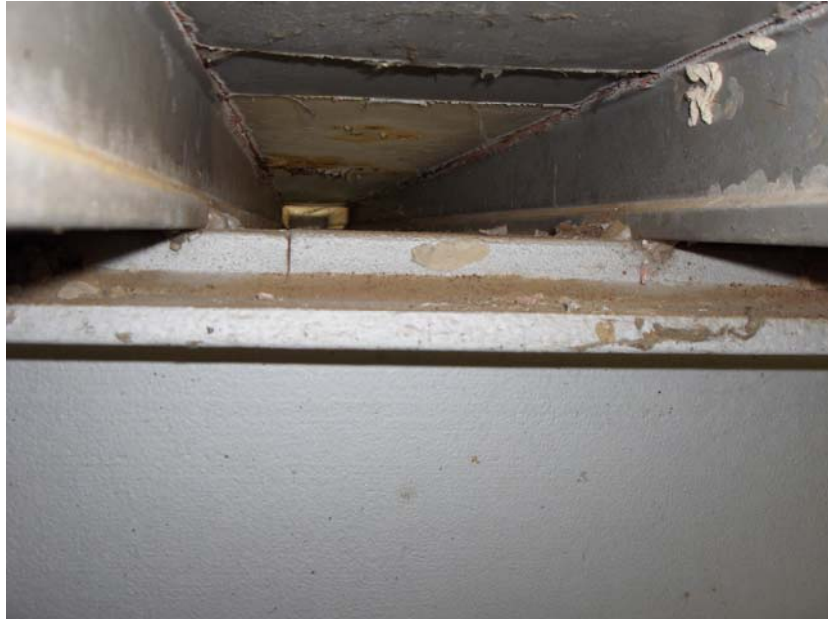
Shim plate and weld detail on stringer top flange.
