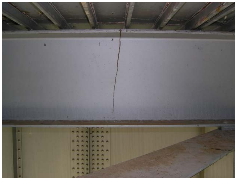
Cracked stringer found during 2005 inspection (prior to repair).
