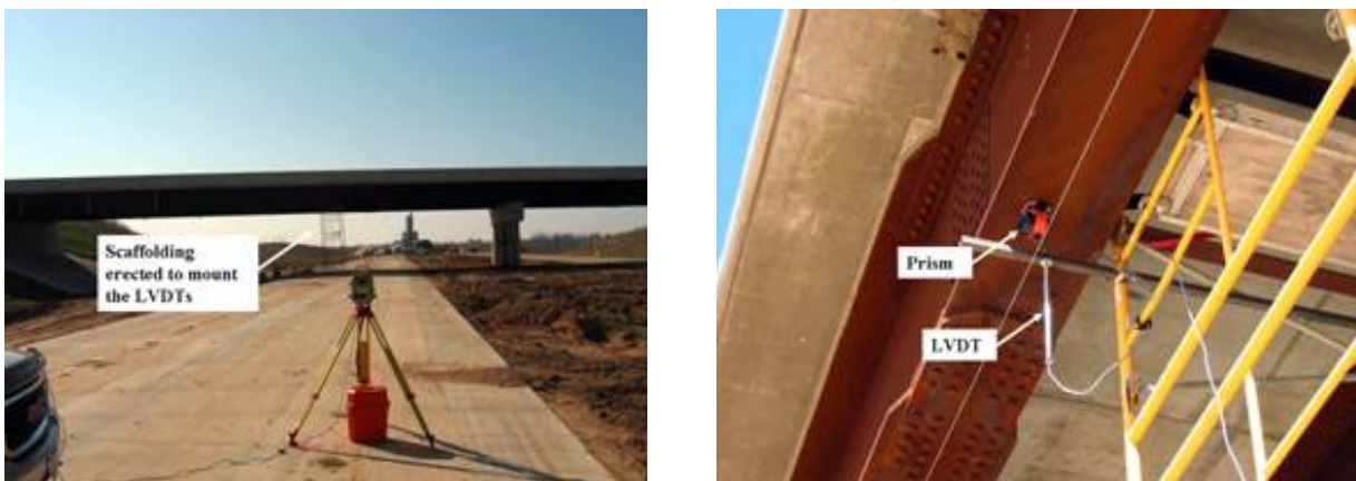
Figure 7 Scaffolding Tower to Mount the LVDTs
