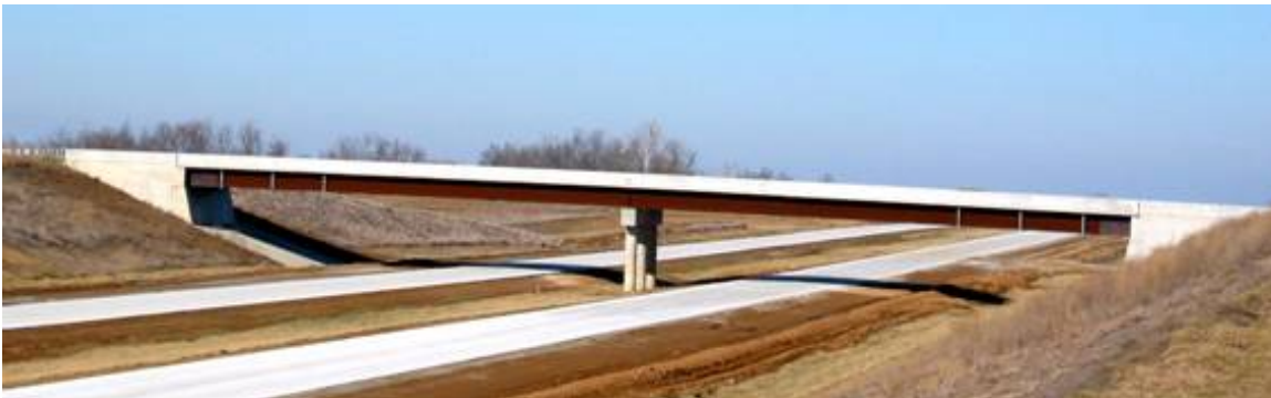
Figure 3 Side View Bridge A6101
