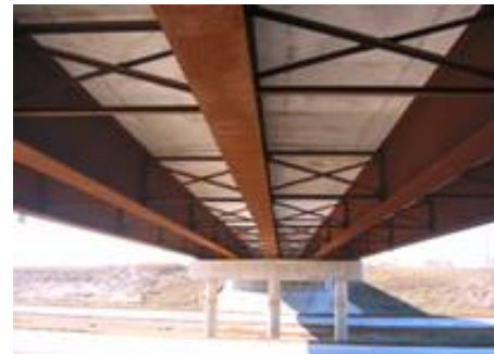
b) Typical Diaphragm (Drawing not in scale, Steel Grade 345 W unless specified)
