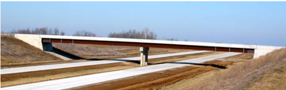
Figure 3 Side View Bridge A602
