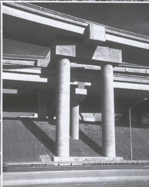
Alemany (I-280/U.S. 101) Interchange San Francisco, California
