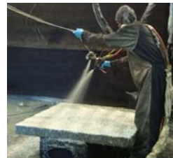
Polyurea application process
