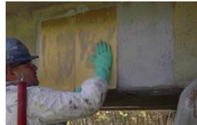
Steel Reinforced Polymer (SRP) Installation
