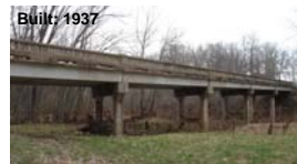
Built: 1937 Bridge T-530, Crawford Co., MO System: Manual Wet-Layup, Plates
