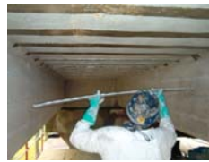
Pre-cured Laminate FRP Installation
