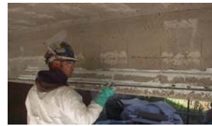
Near Surface Mounted (NSM) Bar Installation
