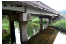
Built: 1948 Bridge X-495, Iron Co., MO System: Manual Wet-Layup
