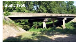
Built: 1956 Bridge P-962, Dallas Co., MO System: Manual Wet-Layup, SRP
