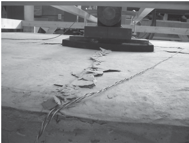
FIGURE 6 Concrete crushing on top surface of SafPlank panel.
