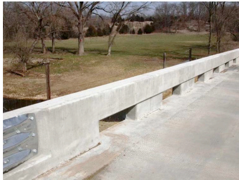
Fig. 2. Reconstruction of Bridge No. 14802301: (a) GFRP reinforcement cages prior to casting of railing; (b) open-post railing in service
