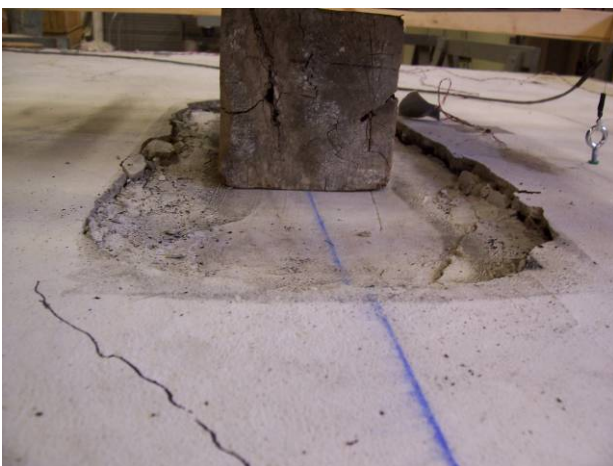
Figure 14 – Imprint of punching shear failure initiation on specimen G1
