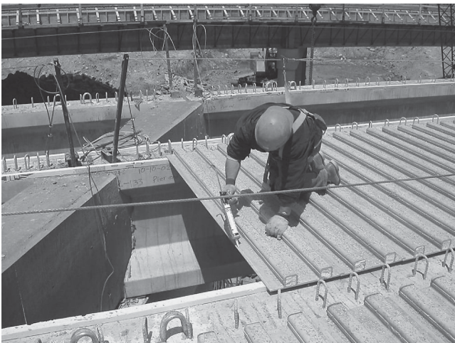
FIGURE 1 Installation of CDS deck panels.
