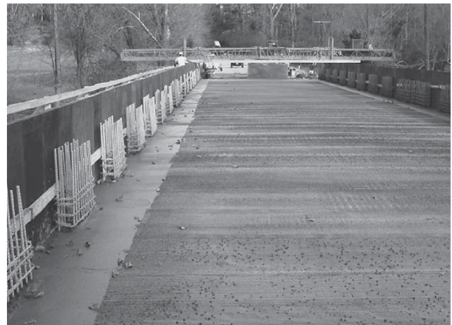
FIGURE 12 Finished bridge deck with rail dowels.
