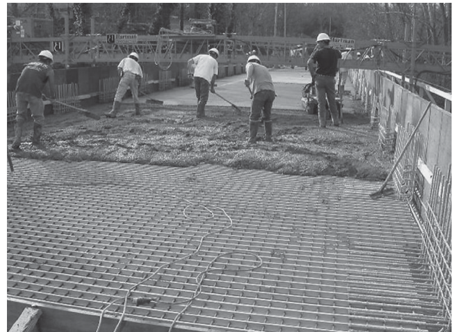
FIGURE 11 Placement of deck concrete with Gridform system.
