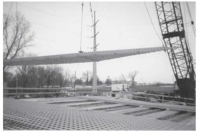
FIGURE 2 Installation of full-width double-layer grid.
