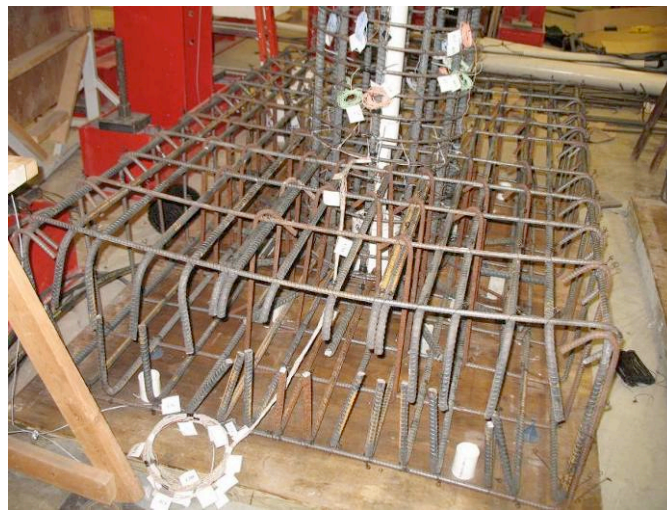
Figure 3.15 Finished Foundation Reinforcement with Column Cage
