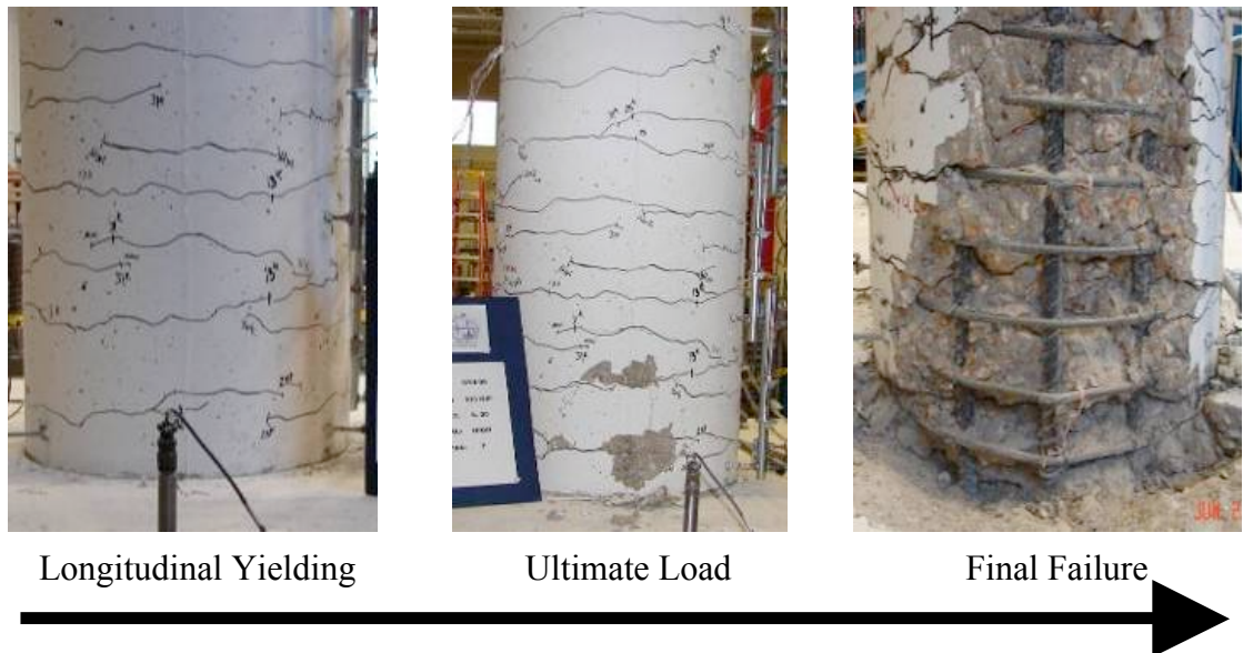
Figure 4.4 Damage to Column H/D(6)-T/M (0.0)-0.73% under Flexure
