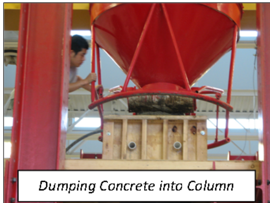
Figure 3.18 Concrete Pour for Foundation and Column
