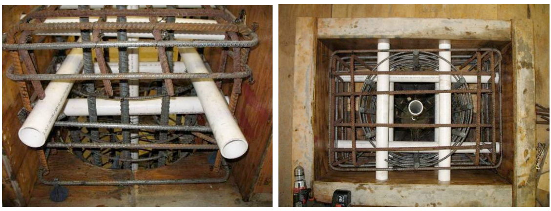
Figure 3.16 Formwork and PVC Layout on Loading Block
