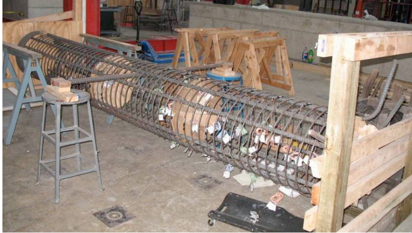
Figure 3.13 Fabrication of Column Cage
