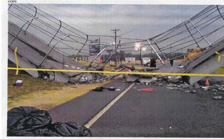
Figure 3: Collapse of a pedestrian bridge outside Lowe’s Motor Speedway North Carolina.
