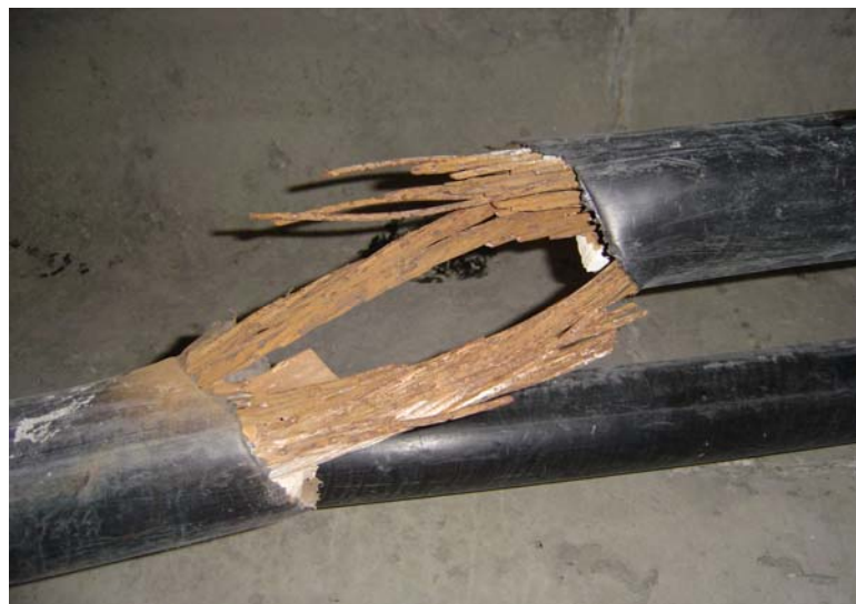
Figure 1: Failure of Prestressing strands in a post-tensioned tendon.
