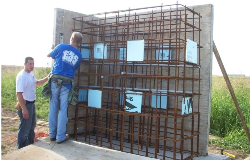
Figure 3.3 : Photograph of the test block during construction showing the targets mounted on the rebar cage.
