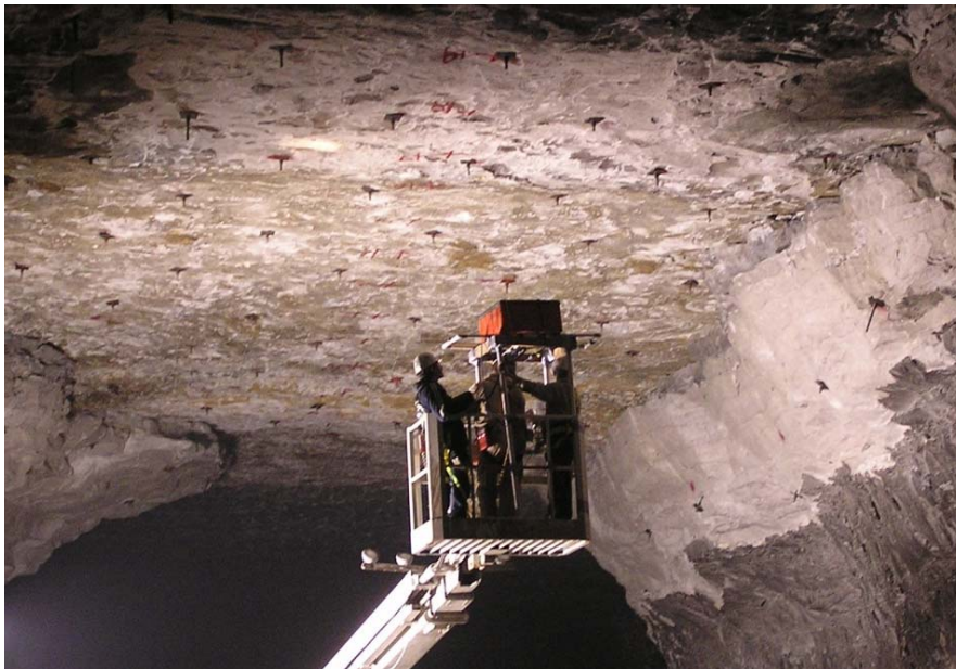
Figure 2: Photograph of ceiling of access tunnel several tens of feet to the west of the zone of failure. Newly installed rock bolts are observed. The crew is acquiring GPR data using a 200 MHz GSSI antenna in an effort to locate clay-filled solution-widened fractures.
