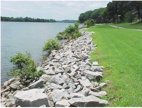
(c) Lake Boundary Erosion Control
