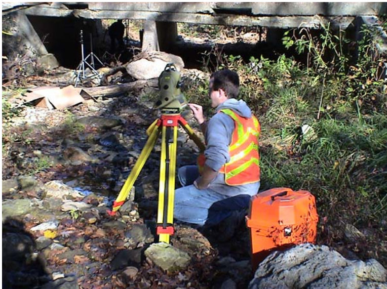
Figure 4.7. Total Station Setup
