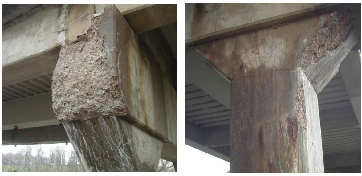
Figure 7.13. Bridge X-596 Corrosion of Bents
