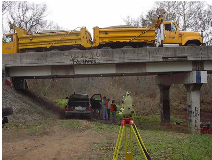
Figure 4.1. Loaded Trucks Used to Test a Bridge
