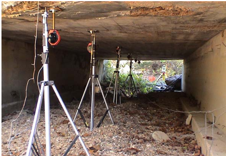
Figure 4.6. LVDTs and Target Prisms
