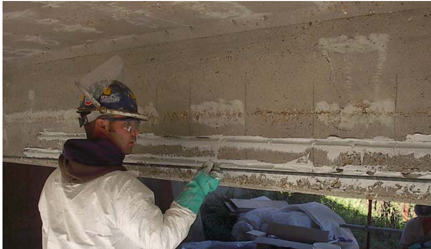
Figure 2.3. NSM Bar Installation
