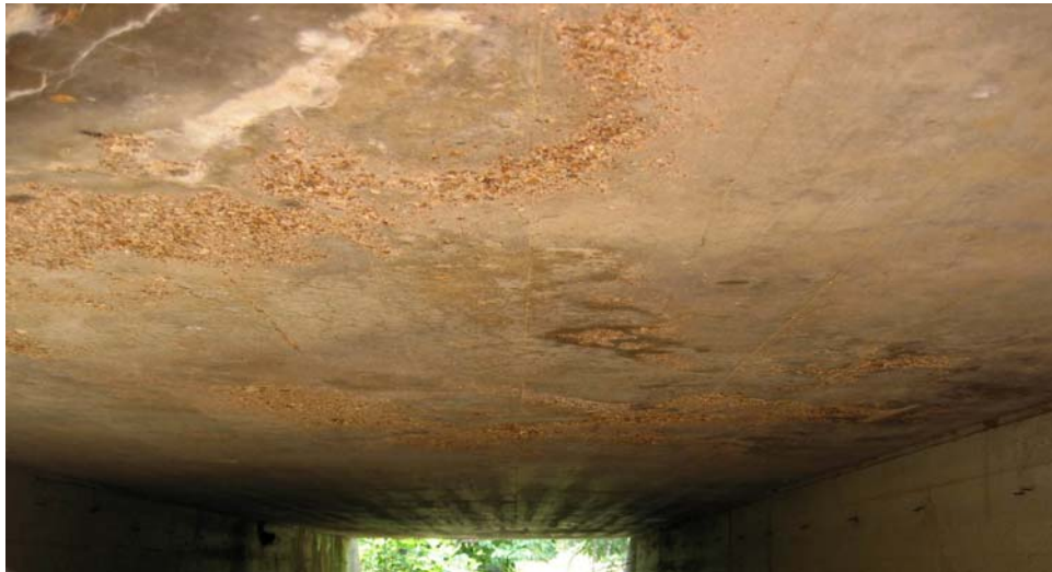
Figure 3.14. Bridge Y-298 Substructure
