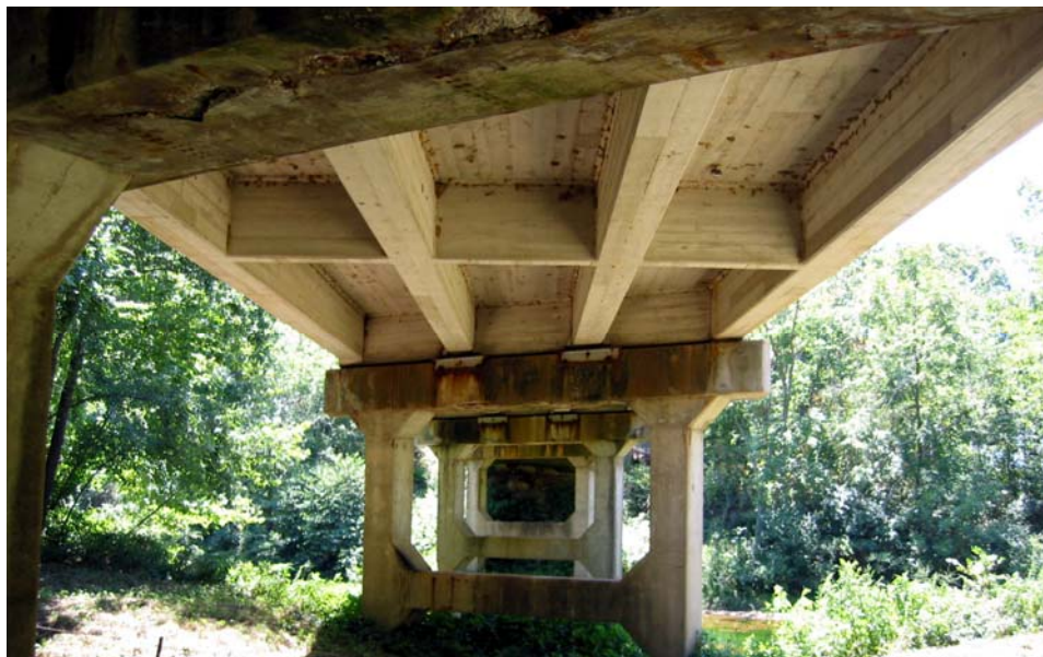
Figure 3.8. Bridge T-530 Substructure
