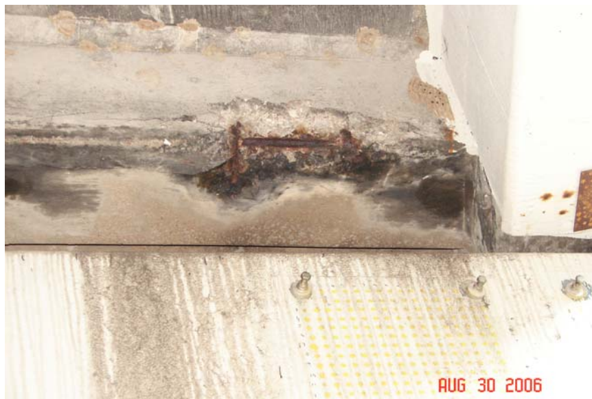
Figure 3.11. Evidence of corrosion 50 years after construction of bridge P-0962
