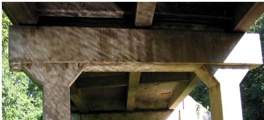
Figure 1.4. Superstructure of bridge P-0962
