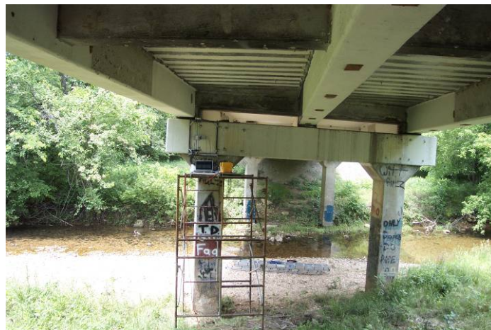
Figure 17 - A picture of the bent with CFRP patches and 2D scanning mechanism with the microwave reflectometer testing CFRP patch #1.
