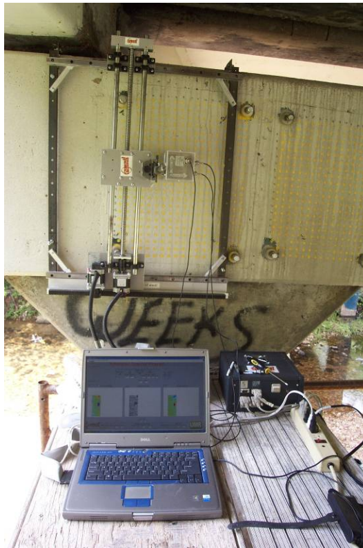
Figure 18 - The dual-polarized microwave reflectometer attached to a scanning platform while inspecting a CFRP patch #1 bonded to the bent of a bridge.
