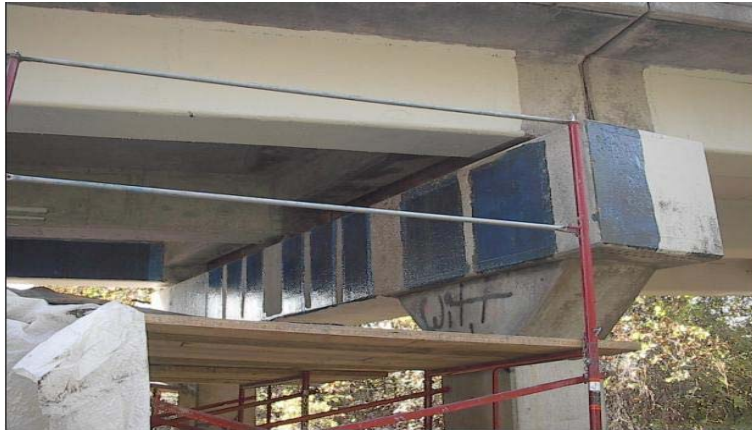
Figure 4 - Picture of bent-A of the bridge P-0962 with FRP bonded patches before they were painted.
