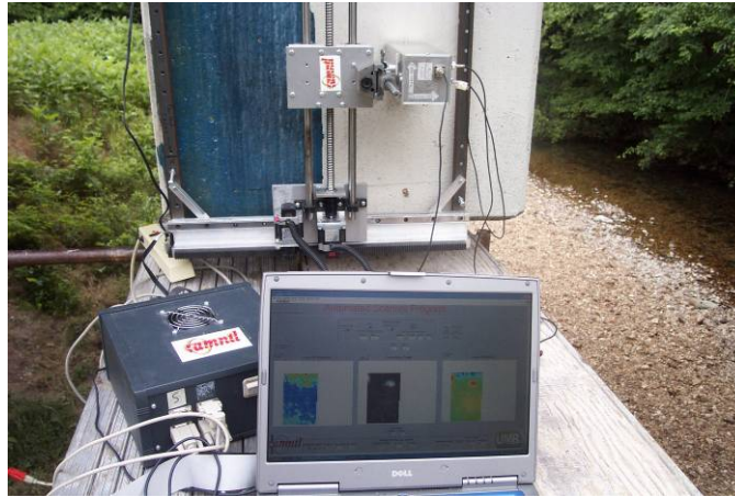
Figure 20 - A picture of the 2D scanning mechanism and the microwave reflectometer testing CFRP patch bonded to the side wall of the bent.
