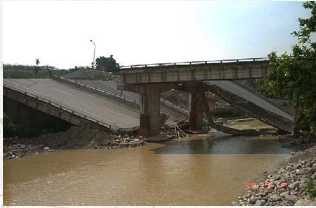
Shi-wei Bridge Collapse during the Chi-Chi Earthquake
