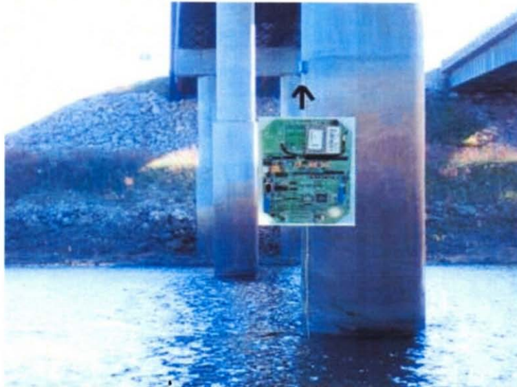
The Flood Frog, a monitoring device developed by researchers at the University of Missouri Rolla was placed on the Osage River Bridge during a field study. The device measures a number of elements including water level, temperature and acceleration. It transmits the information via a wireless network. The goal is to aid in improving the safety and reducing the maintenance cost of infrastructure including bridges. Photos courtesy of Valerio Plessi
