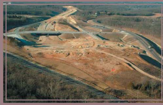
Aerial photograph of the Jefferson County site, prior to the "emptying" of the sinkhole. The approximate location of the sinkhole has been superposed on the photograph with an "x."
