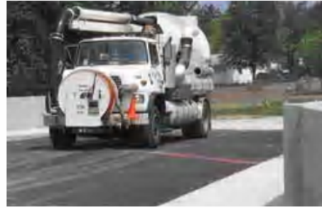
The bridge that crosses Carter Creek on Southview Drive in Rolla has a split personality, with one lane using conventional technologies (left) and the other lane employing the latest in fiber-reinforced polymer composites.
