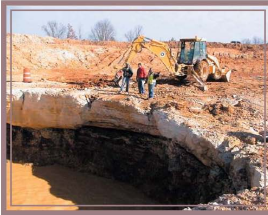
Close-up photograph of the walls of the emptied sinkhole, taken from a location immediately south of the feature.
