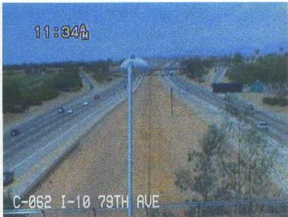
I-10 and 79 th Ave in Phoenix, Arizona (ADOT)
