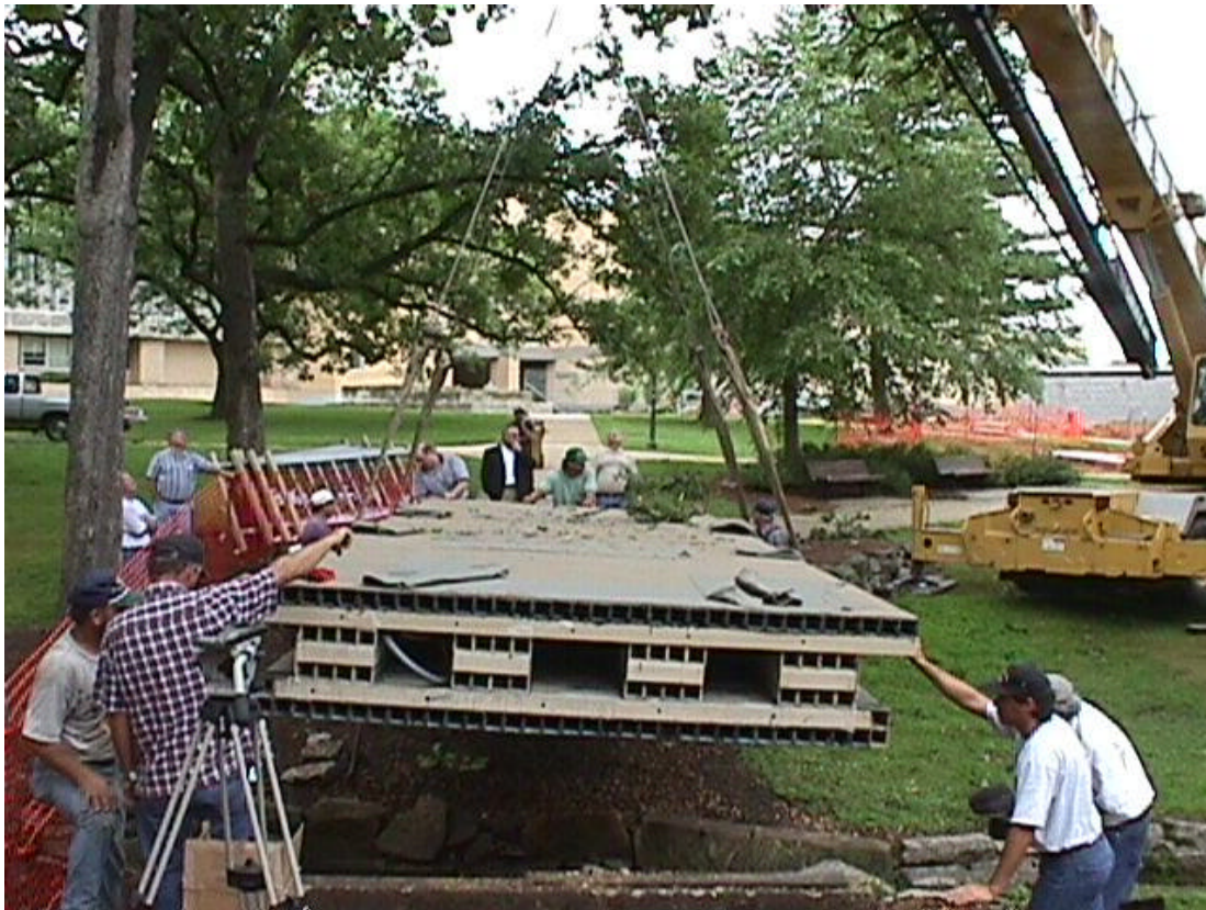
Figure 26: Installation of bridge deck
