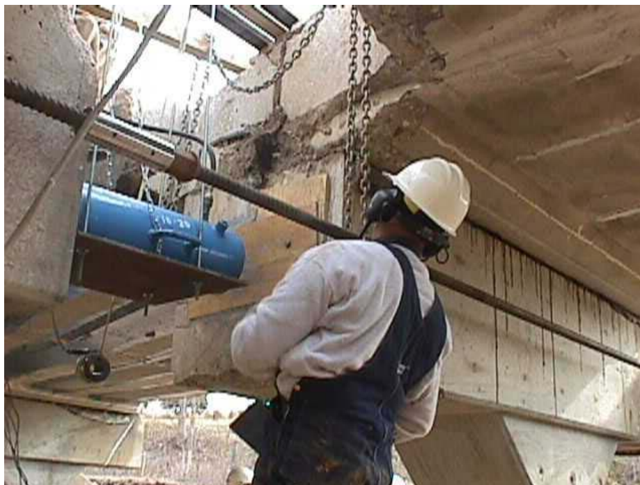
Figure 3.9. Placing the middle jack.
