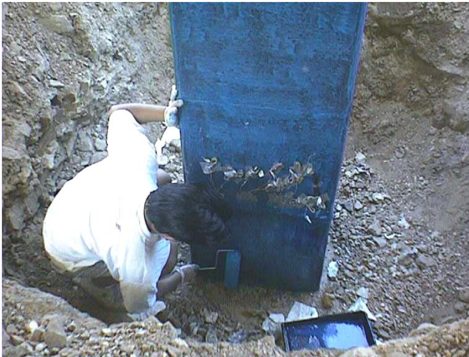
Figure 2.11. Applying the bottom lift of the jacket.
