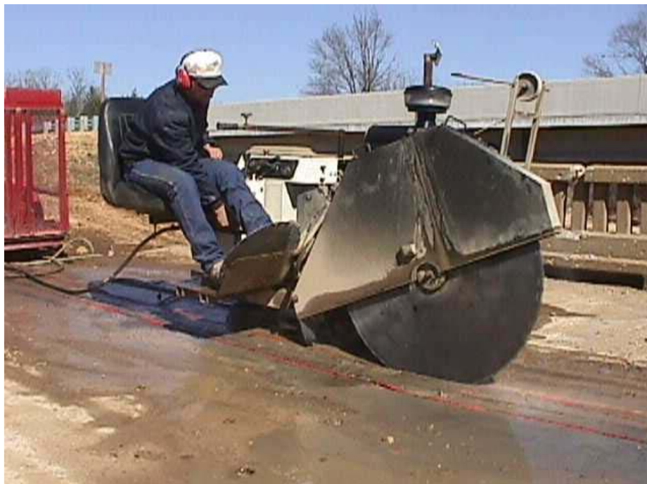
Figure 3.1. Cutting the bridge deck.
