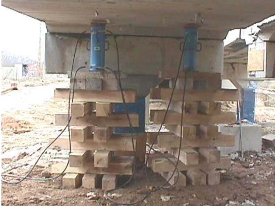
Figure 3.12. Set up for jacking the decks.
