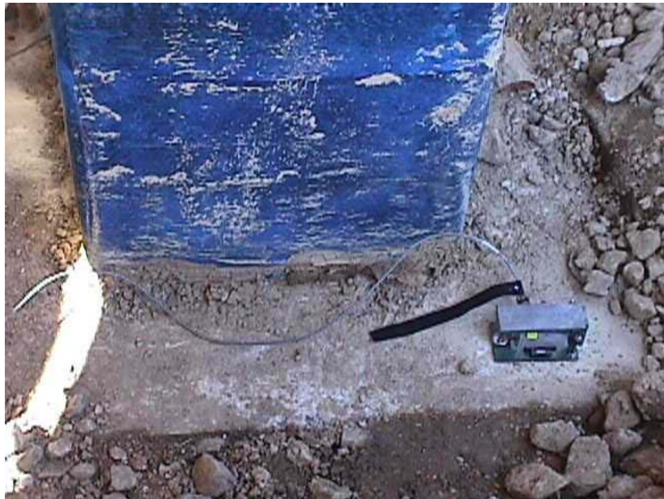
Figure 3.17. Inclinometer on the surface of the footing.
