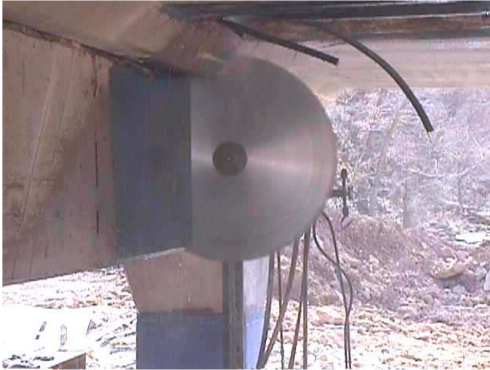
Figure 3.2. Cutting the cap beam.
