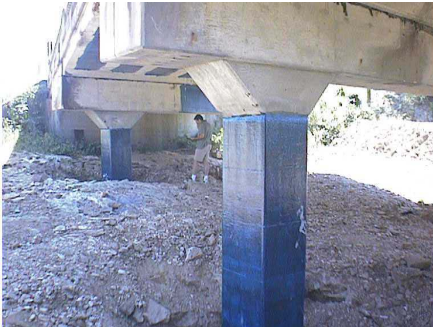
Figure 2.13. Photo showing the bridge after strengthening.
