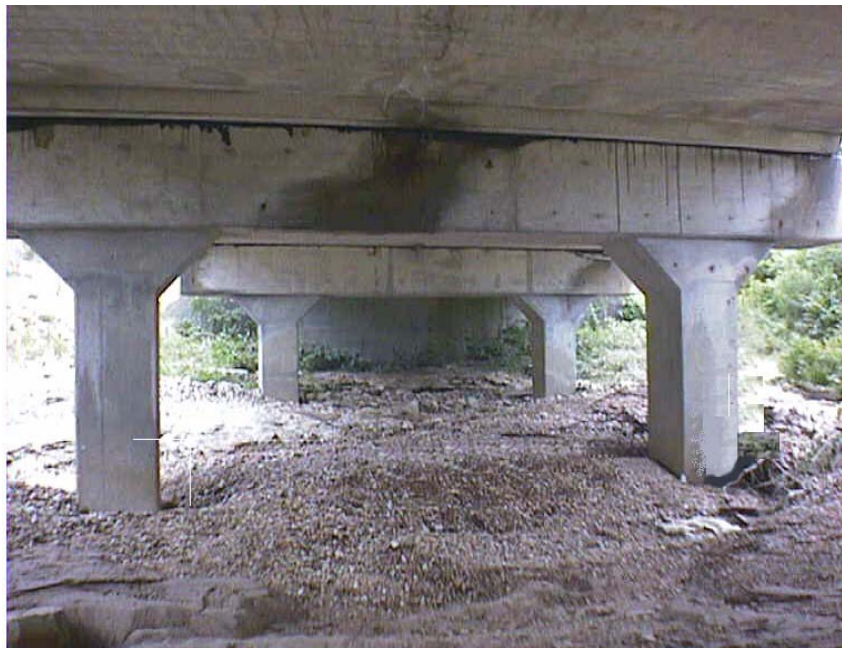
Figure 2.1. Photo showing bridge columns.
