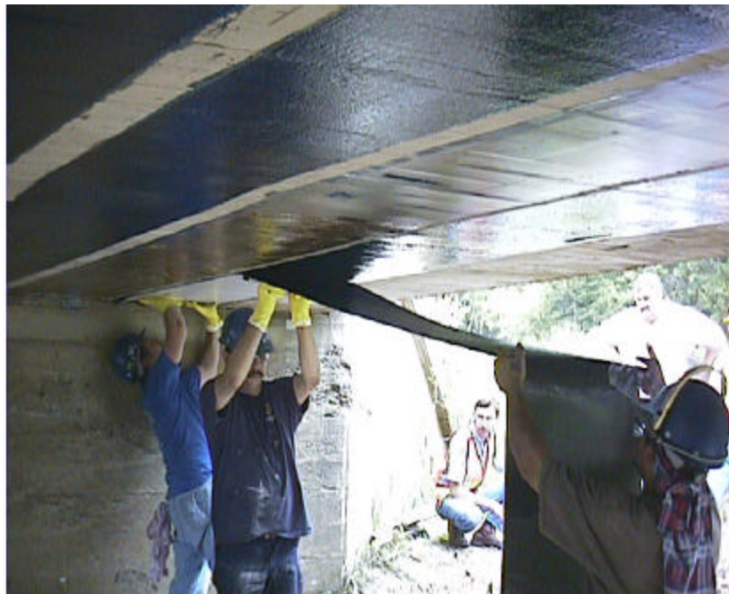
Figure 6.2. Installation of the CFRP Sheets
