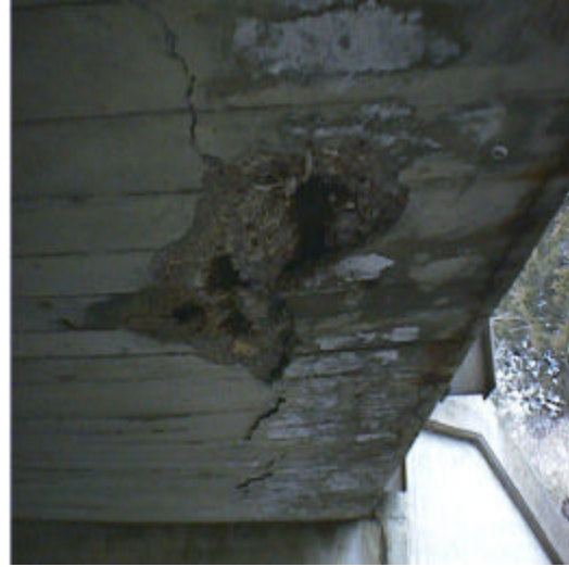
Figure 7.2. Corrosion on North Side
