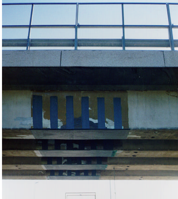
Figure 2.5. Pattern of CFRP Strips
