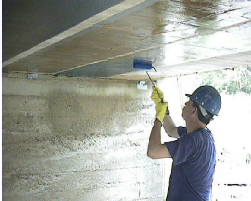
Figure 6.1. Application of the Saturant
