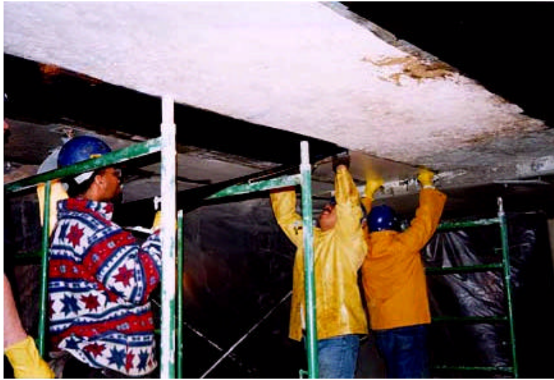
Figure 2.9. Application of CFRP Sheet
