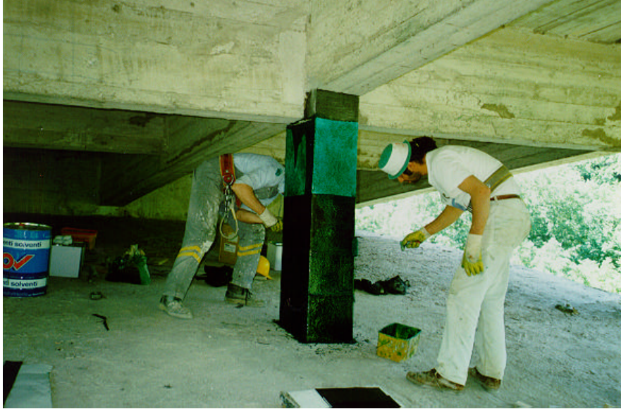
Figure 2.8. Application of the CFRP to Column
