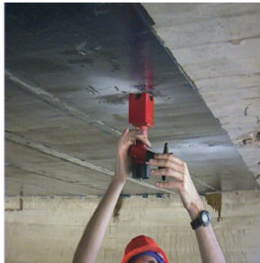
Figure 7.9 Pull-off Test Apparatus
