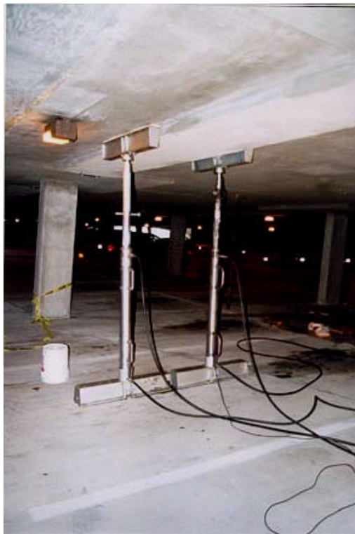
Figure 2.10. Site Load Test of the Repaired Structure
