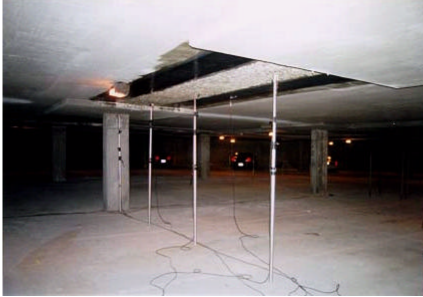
Figure 2.11. Measurement of Deflection During Loading
