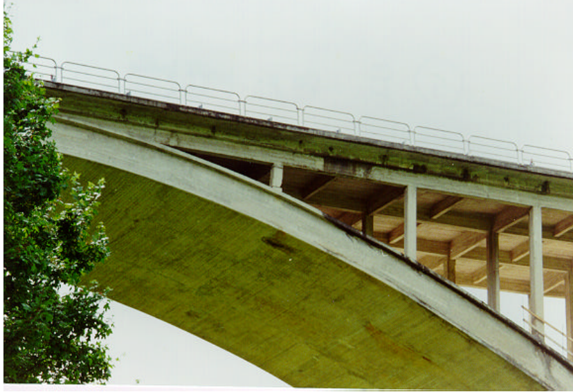
Figure 2.6. View of Bridge
