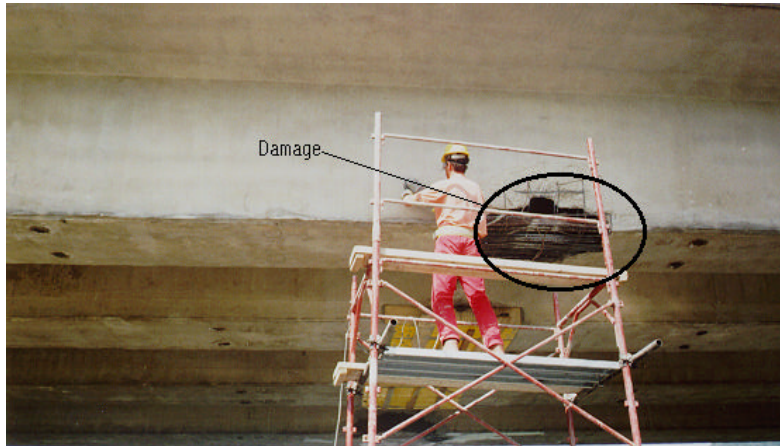
Figure 2.4. Girder Damage Due to Vehicular Impact
