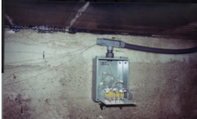
Figure 7.4. Junction Box of the Fiber Optic Sensors
