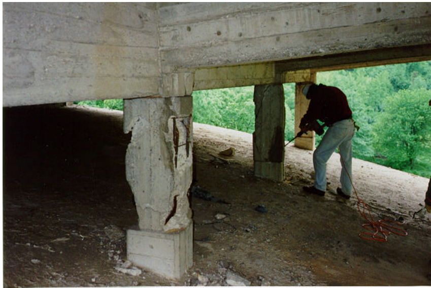
Figure 2.7. Deteriorated Columns
