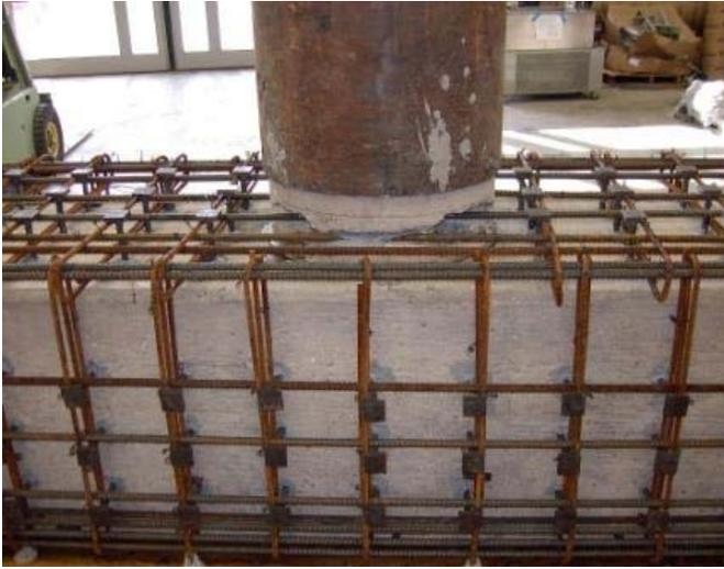
**Figure 0-24. Retrofit Section Reinforcing Cage**
