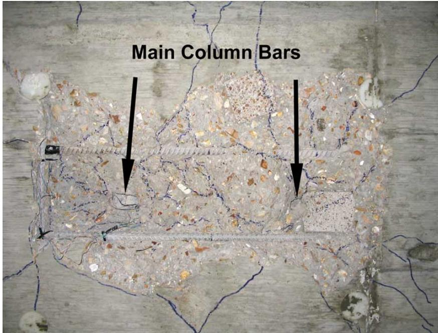
**Figure 0-35. Underside of Bent Cap Cracking Pattern**
