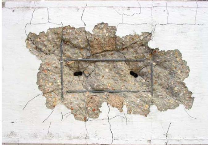
**Figure 0-18. Underside of Bent Cap Ultimate Damage**
