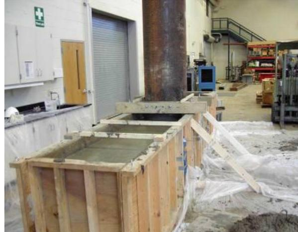
**Figure 0-17. Casting of the Bent Cap**
