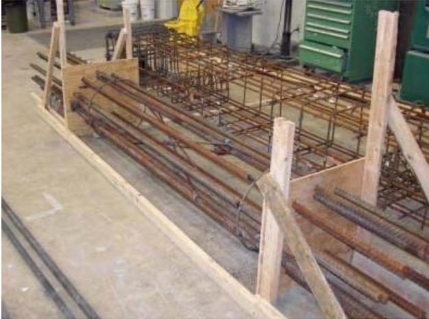
**Figure 0-12. Column & Cap Reinforcing Cage**
