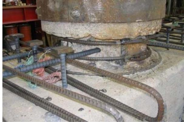
**Figure 0-4. Detail at Bent Cap Interface**
