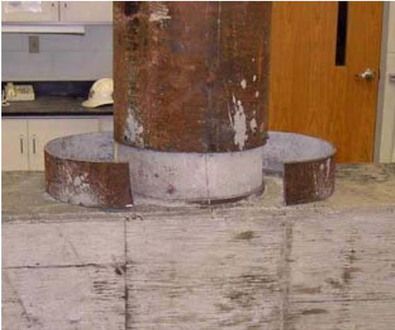
**Figure 0-20. Cutting Steel Shell Casing**
