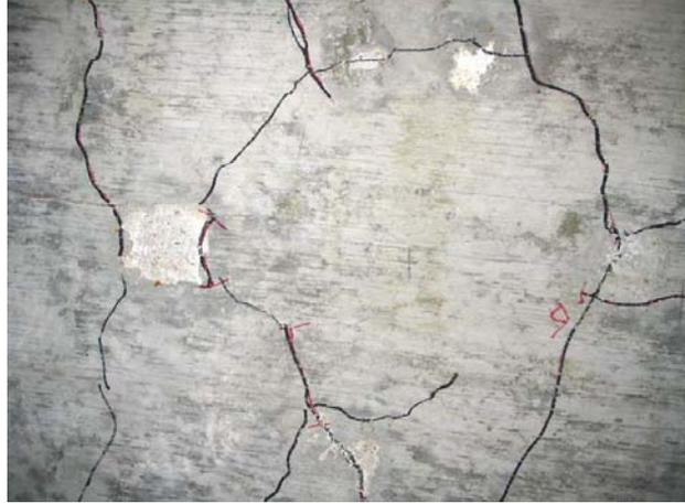
**Figure 0-23. Cracking on Underside of Bent Cap**
