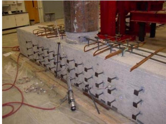
**Figure 0-21. Installing Headed Reinforcing**
