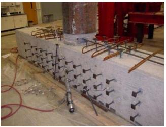
Figure 0-21. Installing Headed Reinforcing
