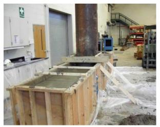
Figure 0-17. Casting of the Bent Cap
