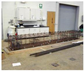
Figure 0-12. Column & Cap Reinforcing Cage Figure 0-13. Bent Cap Reinforcing Cage
