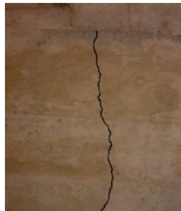
b) Vertical Crack in the Abutment
