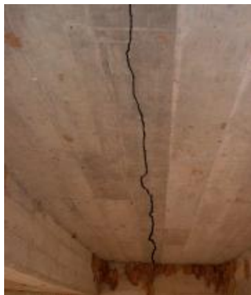
a) Longitudinal Crack in the Deck
