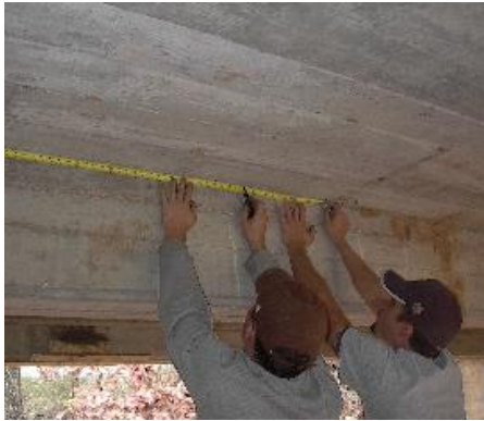
Figure E. 2. Positioning of the Pre-cured FRP Laminates
