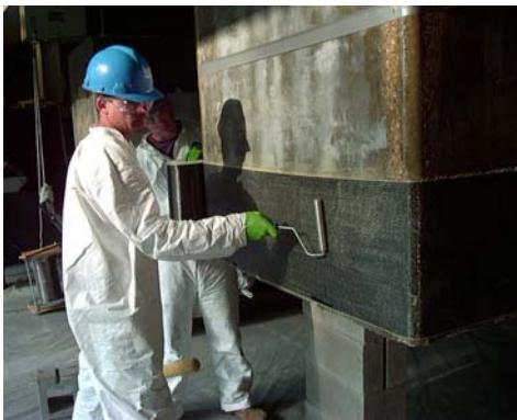
(c) Rolling to eliminate bubbles
