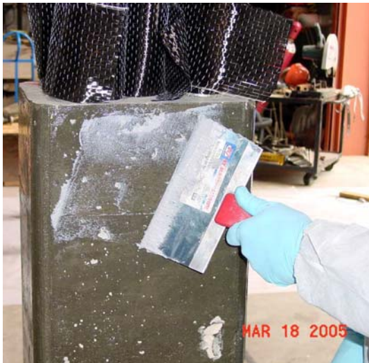
Figure 6-16 Application of Mapewrap 11 (Putty)
