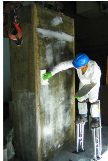
Figure 6-16 Application of Mapewrap 11 (Putty)
