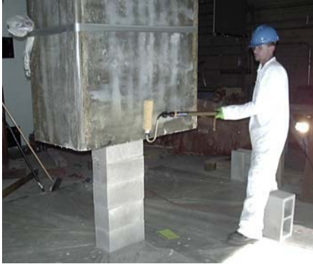
(a) First coat of saturant
