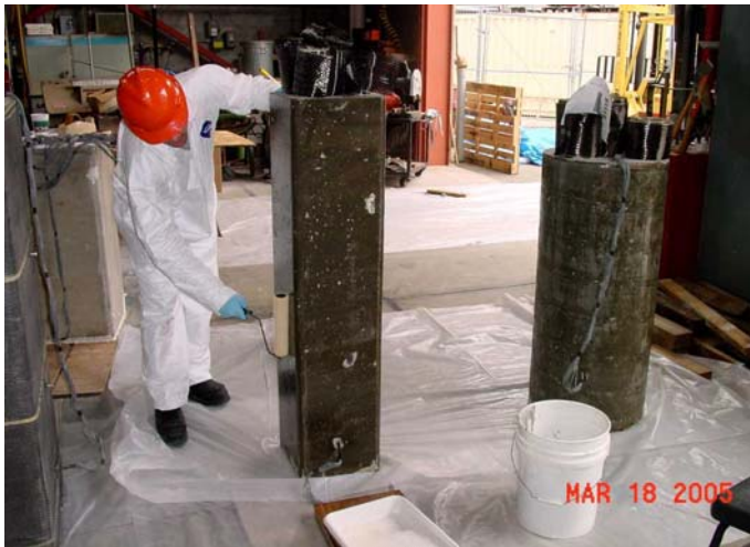
Figure 6-15 Application of Mapewrap 1 Primer to Concrete Surface
