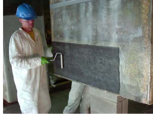
(b) Placing the carbon fabric
