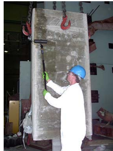
Figure 6-15 Application of Mapewrap 1 Primer to Concrete Surface
