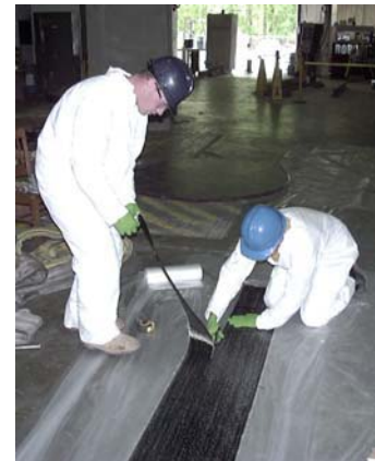
Figure 6-14 Layout and Cutting of the Fibers
