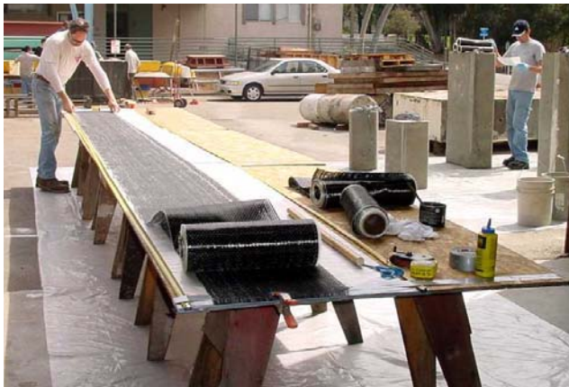
Figure 6-14 Layout and Cutting of the Fibers
