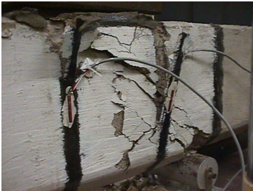
Fig. 13 – CFRP debonding in failure of Beam 3
