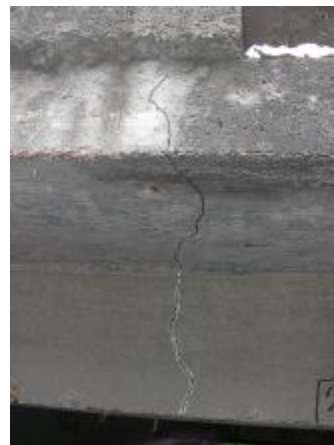
b) Bending Cracks in the Girders
