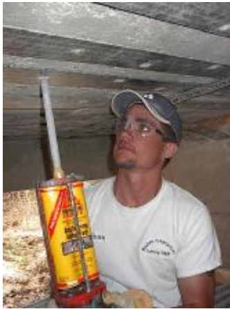
a) Hole Filling with Epoxy
