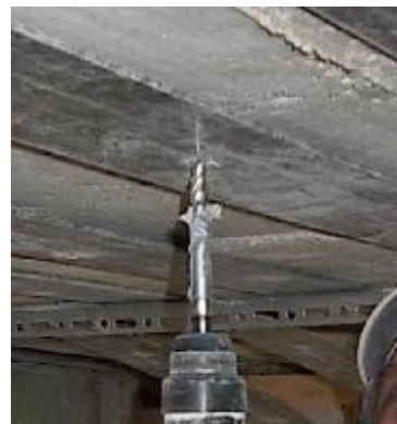
Figure C. 3. Drilling of the Holes in the Concrete
