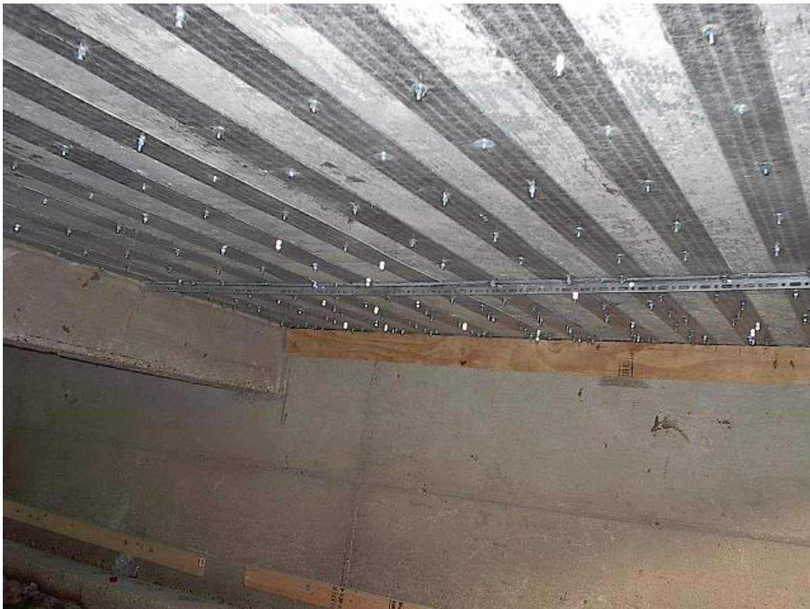
Figure C. 5. Bridge No. 3855006 after Strengthening
