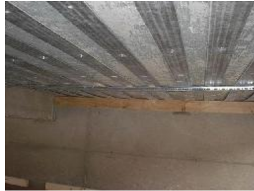
b) Temporary Attachment of the Laminates
