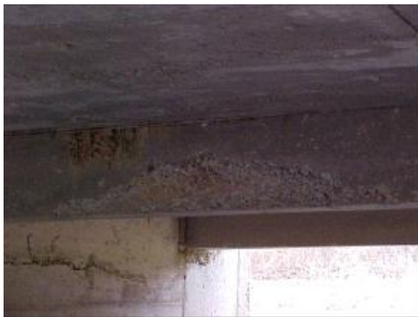
a) Girders and Deck
