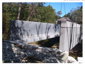
c.) Non-Instrumented HSC Beam Set on Embed Plates
