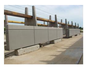
a.) Sand-Blasted Side of Spandrel Beam Storage
