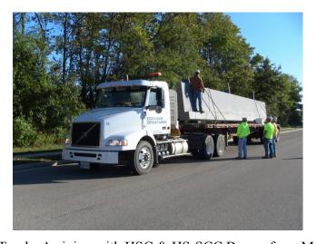
Figure 4.9. Trucks Arriving with HSC & HS-SCC Beams from Marshall, MO.
