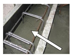
Figure 4.3. Scribed Crosses Used to Prevent Cold-Joint in HS-SCC Beam.
