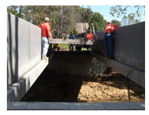
Figure 4.12. Slabs Placed on Top of Neoprene Pads on Top of HSC Beams.
