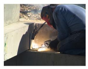
Figure 4.11. HSC Beam Welded to Abutment.
