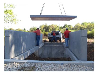
Figure 4.14. HS-SCC Deck Panel Erection.
