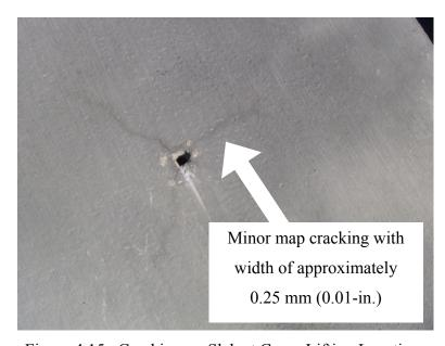
Figure 4.15. Cracking on Slab at Crane Lifting Location.
