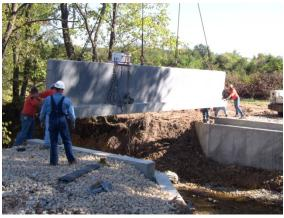
a.) Crane Lifting Instrumented HS-SCC Beam
