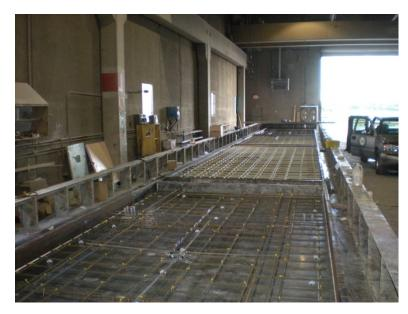
Figure 4.5. Formwork, Steel, & GFRP for the Deck Panels.
