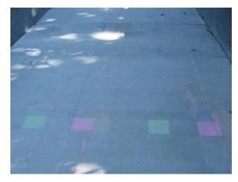
Figure 11.2. Example Fork Lift Load Path Markings.
