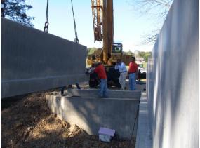
c.) Non-Instrumented HS-SCC Beam Set on Embed Plates
