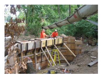
Figure 4.8. Abutment Placement for HSC Bridge Location.
