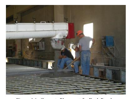
Figure 4.6. Concrete Placement for Deck Panels.
