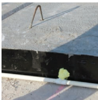
Protecting gage cables from exposure to moisture and Data collection system
