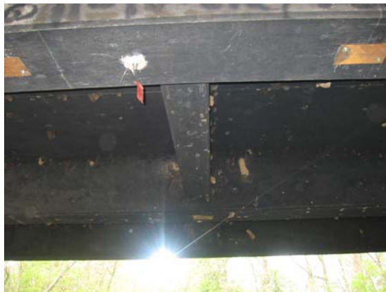
Figure 3. Condition of deck
