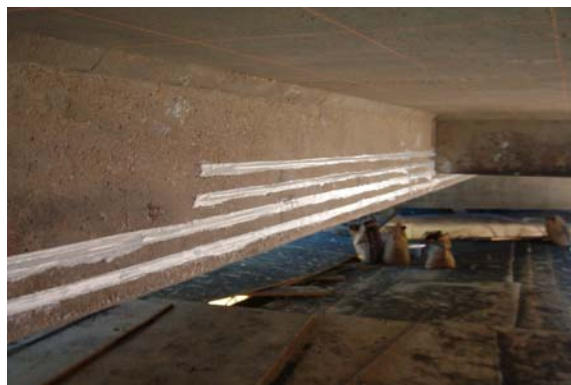
Figure 16. Installed NSM bars
