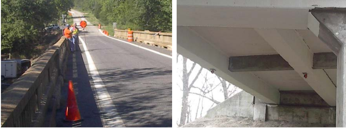
Figure 12. Traffic control and topcoat protection
