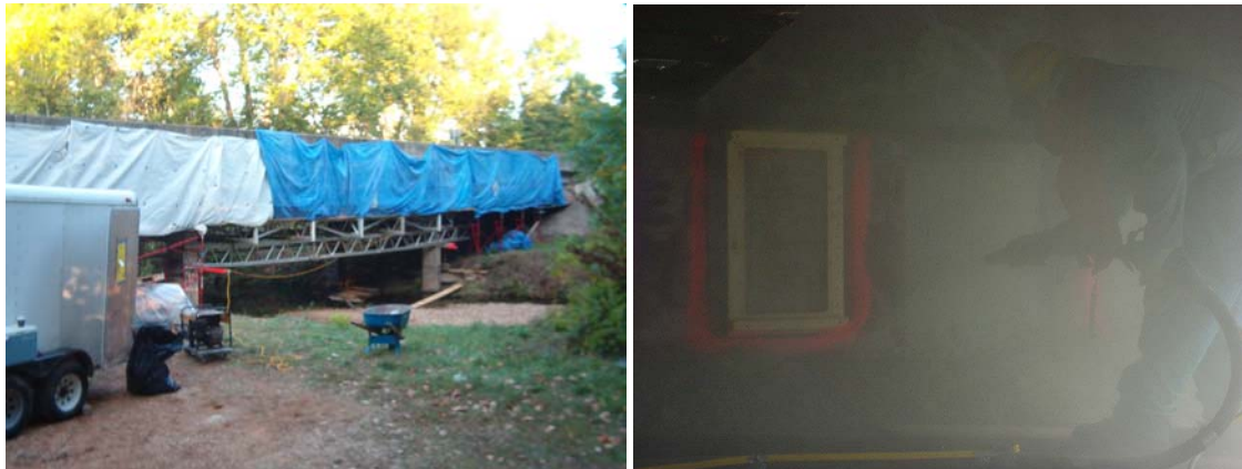
Figure 6. Preparation of appropriate roughness by sandblasting
