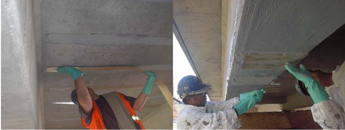
Figure 18. SRP installation and full impregnation by rolling
