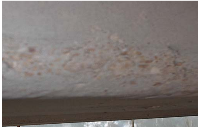
Figure 5. Rounding of corners on girder
