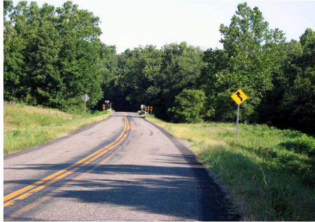
Figure 1. Approach to the bridge
