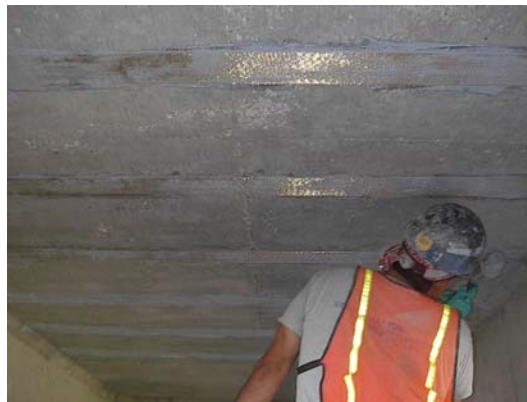
Figure 19. Full impregnation by a second epoxy application
