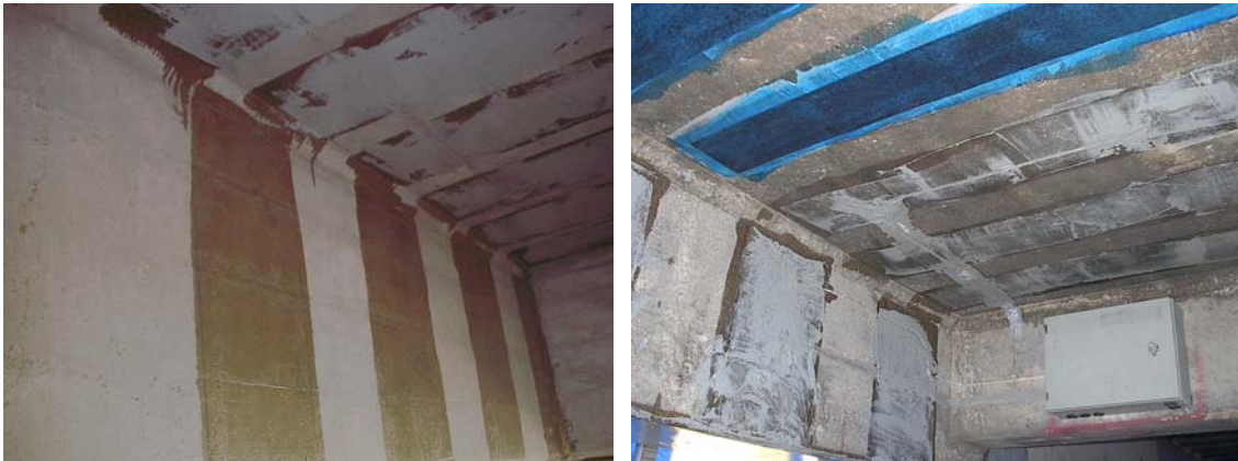
Figure 7. Filling of voids and defects by primer and putty collocation
