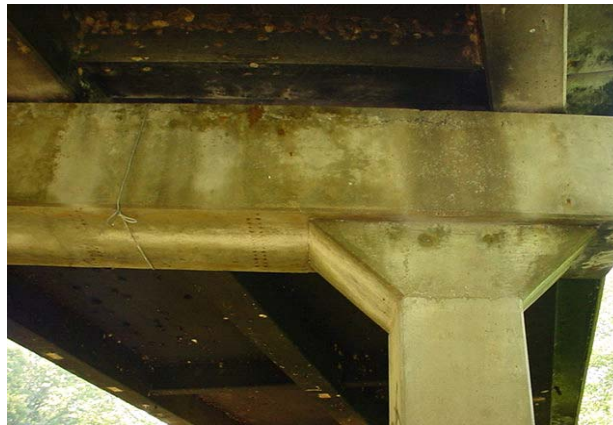
Figure 2. Condition of bent
