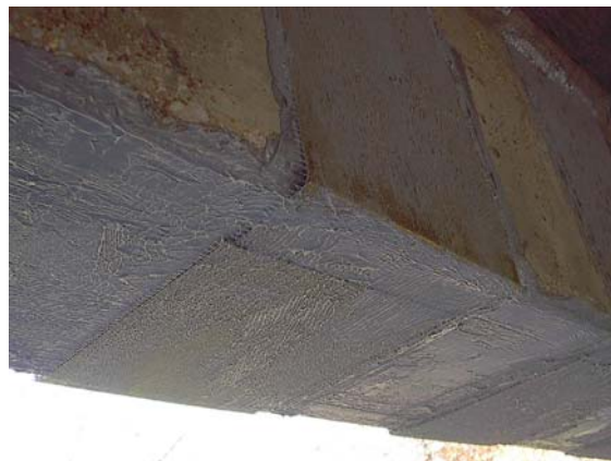
Figure 21. Overlapping to form a U-Wrap
