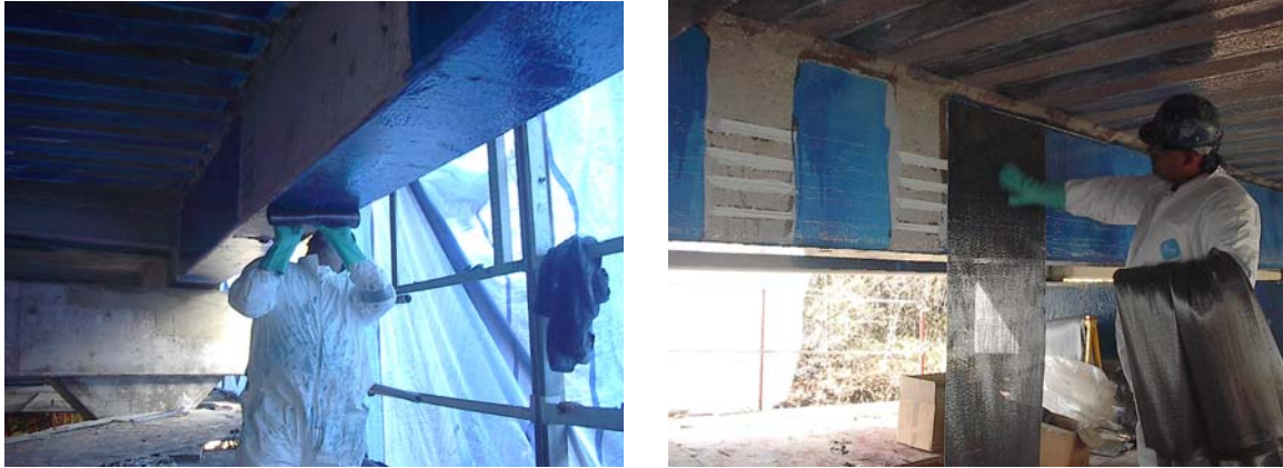
Figure 10 Manual lay-up CFRP sheet installation.
