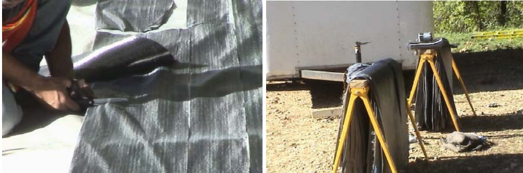
Figure 8. Cutting process of CFRP sheet
