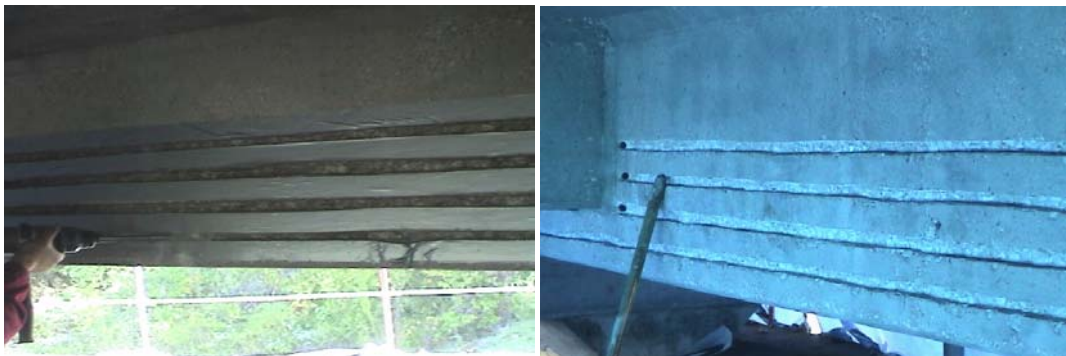
Figure 13. Grooving of girder surface for the NSM bars
