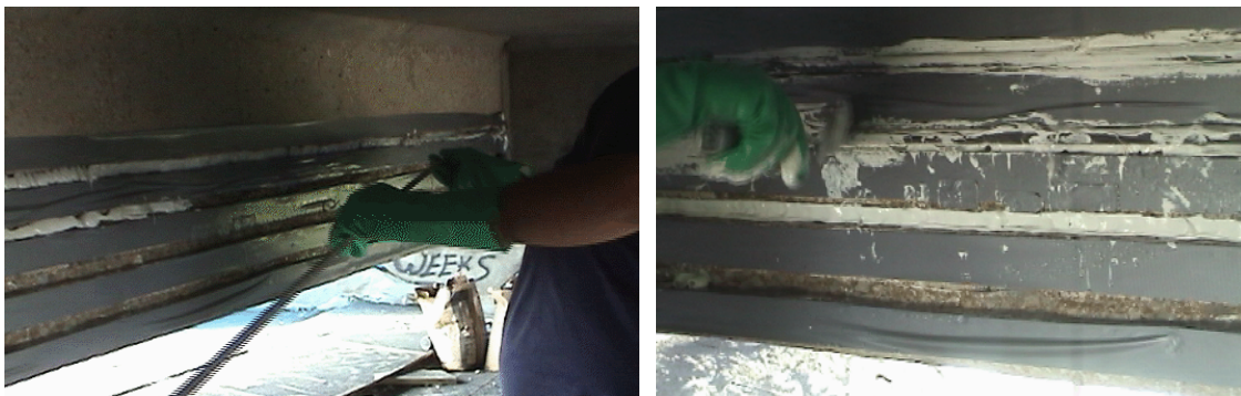
Figure 15. Bar installation
