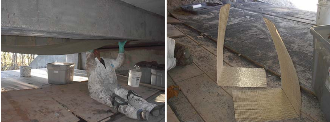
Figure 20. Installation of flexural reinforcement. U-Wrap formed by two L-Shapes
