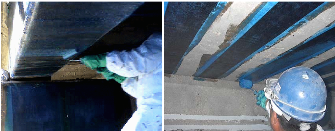
Figure 11. Squeezing of air bubbles and saturation over laminates
