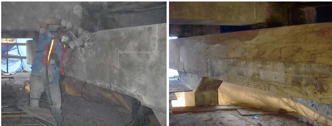
Figure 4. Repair of deteriorated areas on one bent. Bent after repair
