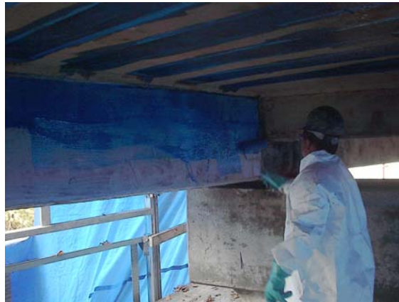
Figure 9. Saturant application
