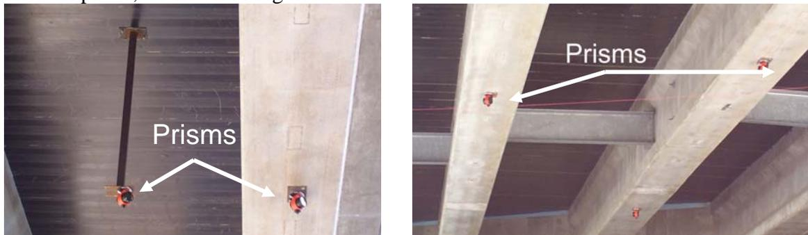
Figure 8 Targets Mounted on Bridge Girders and Deck
