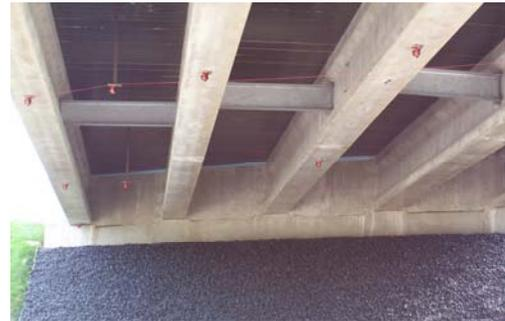
b) Typical Diaphragm (Drawing not in scale)
