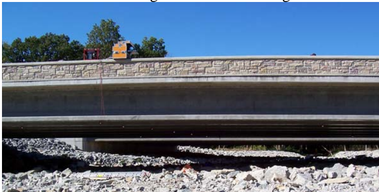
a) Bridge B-20-148
