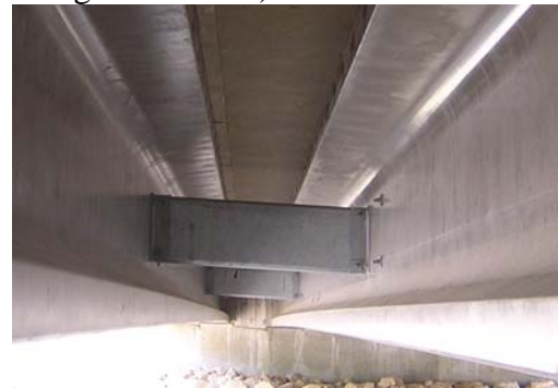
b) Typical Diaphragm (During Construction Phase of Bridges)
