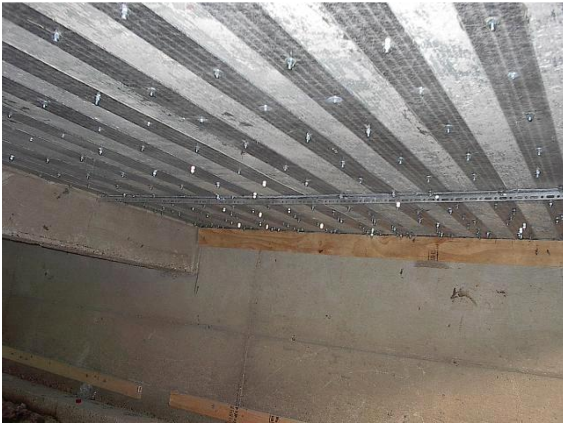
Figure C. 5. Bridge No. 3855006 after Strengthening
