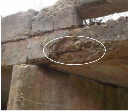
c) Exposed Bar in the Lateral Side
