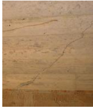
d) Crack Parallel and Normal to the Traffic Direction
