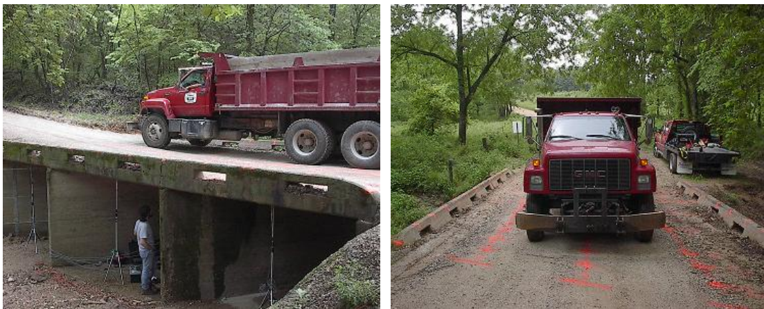
Figure 5.1. Load Tests after Strengthening on Bridge No. 2210010
