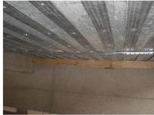
b) Temporary Attachment of the Laminates
