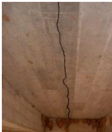
a) Longitudinal Crack in the Deck
