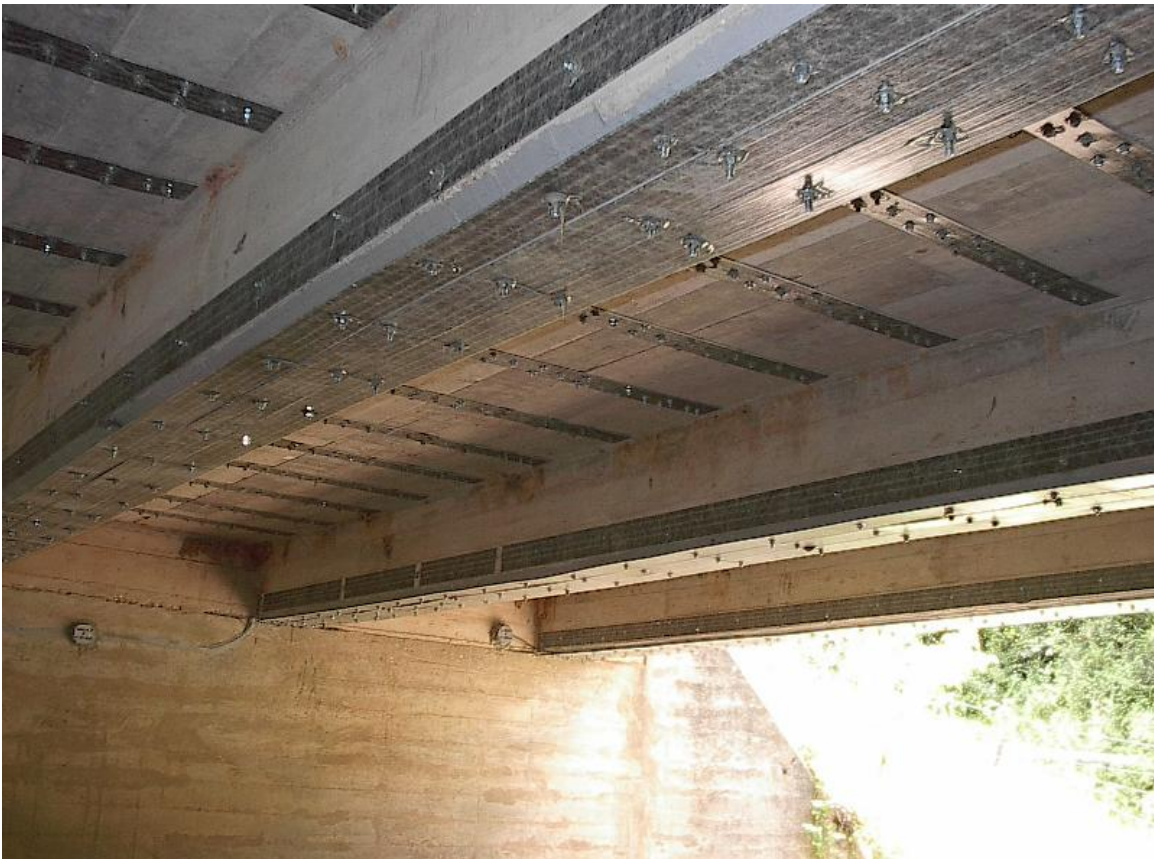
Figure E. 5. Bridge No. 1330005 after Strengthening
