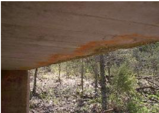
a) Steel Rebar Corrosion on the Deck
