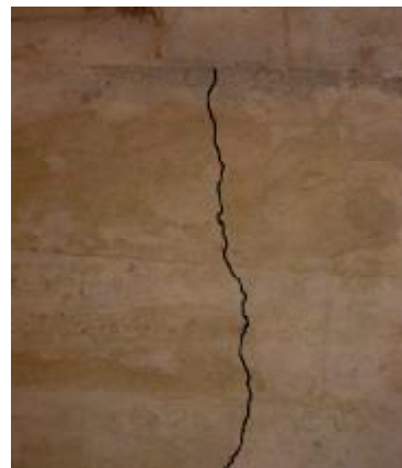
b) Vertical Crack in the Abutment
