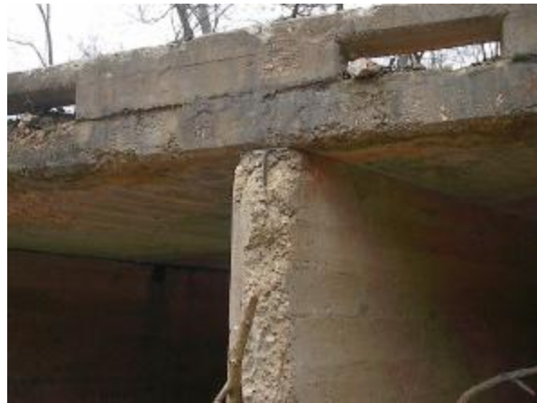
b) Exposed Bar in the Corner
