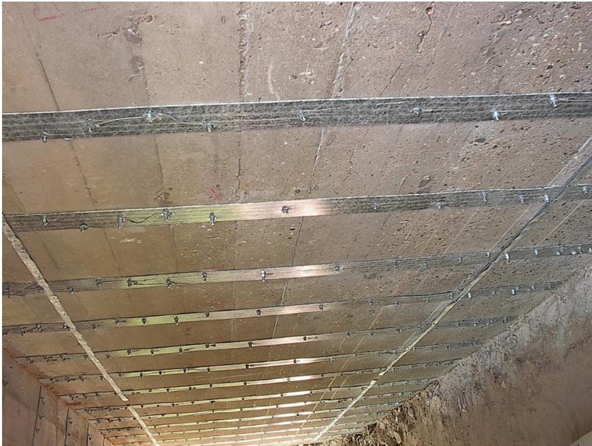
Figure C. 5. Bridge No. 2210010 after Strengthening
