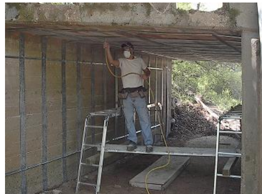
Figure C. 3. Drilling and Dusting of the Holes in the Concrete
