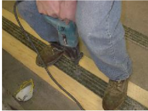
Figure E. 1. Drilling of the Pre-cured FRP Laminates
