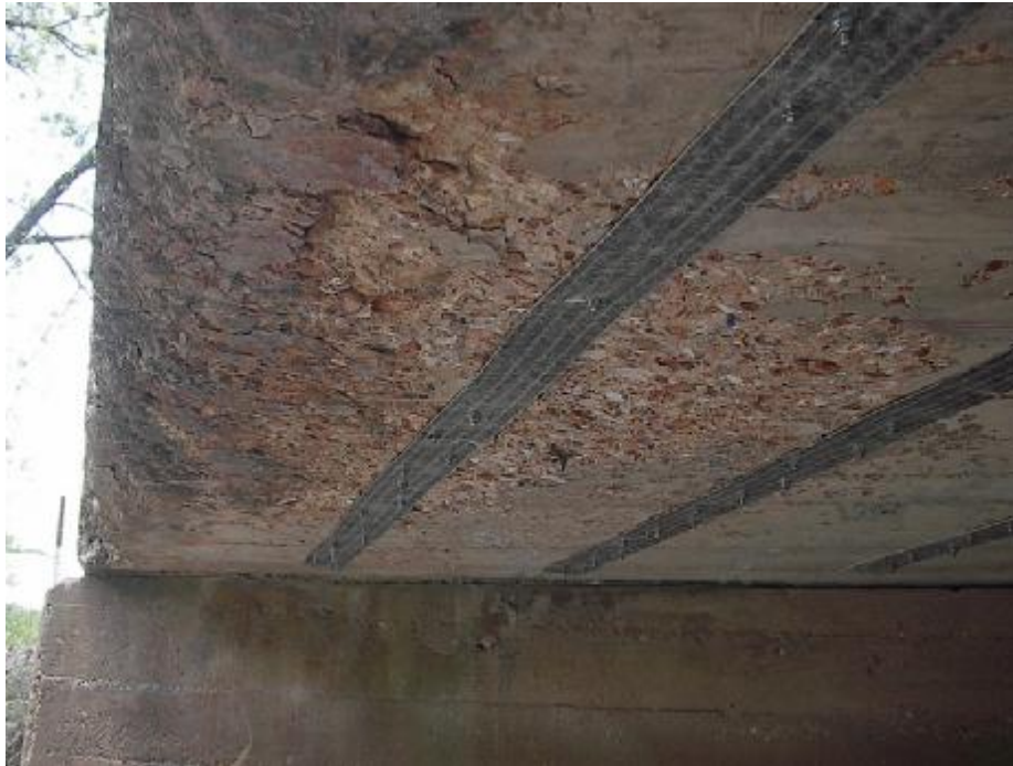
a) Pre-cured FRP Laminate Fastened beneath a Highly Deteriorated Part of the Deck
