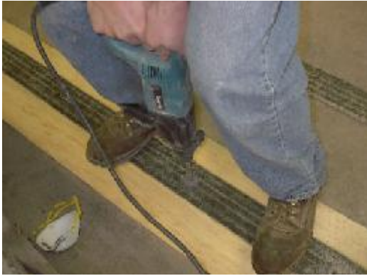
a) Drilling of the Pre-cured FRP Laminates
