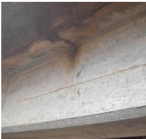
a) Girders and Deck
