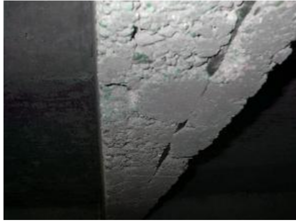
b) Exposed Bar in the Bottom Side
