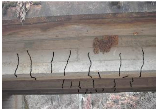
b) Bending Cracks in the Girders
