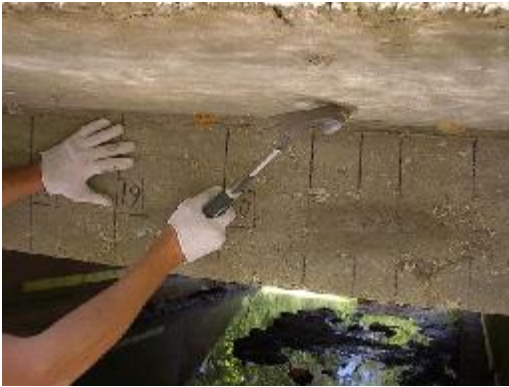
a) Removal of Surface Unevenness
