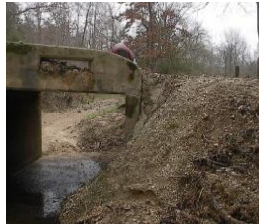
b) Soil not in Perfect Contact with the Surface of the Abutment
