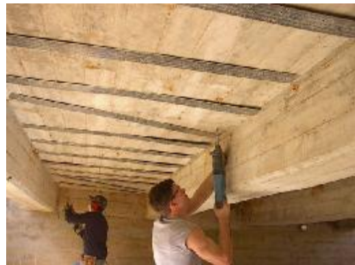
Figure E. 3. Drilling of the Holes in the Concrete
