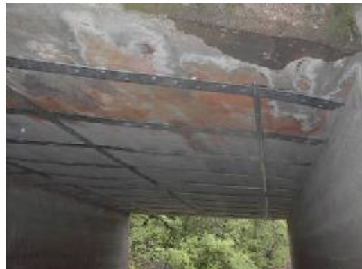
b) Temporary Attachment of the Laminates
