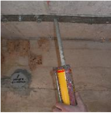
a) Hole Filling with Epoxy
