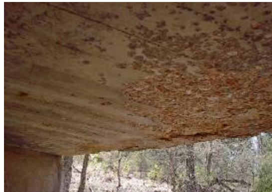
b) Erosion on the Deck
