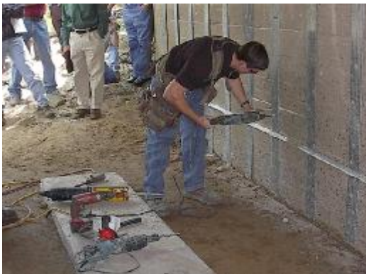
Figure C. 3. Drilling and Dusting of the Holes in the Concrete
