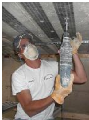
Figure C. 3. Drilling of the Holes in the Concrete
