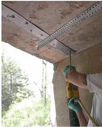
a) Hole Filling with Epoxy
