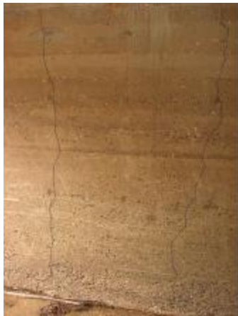
a) Vertical Cracks
