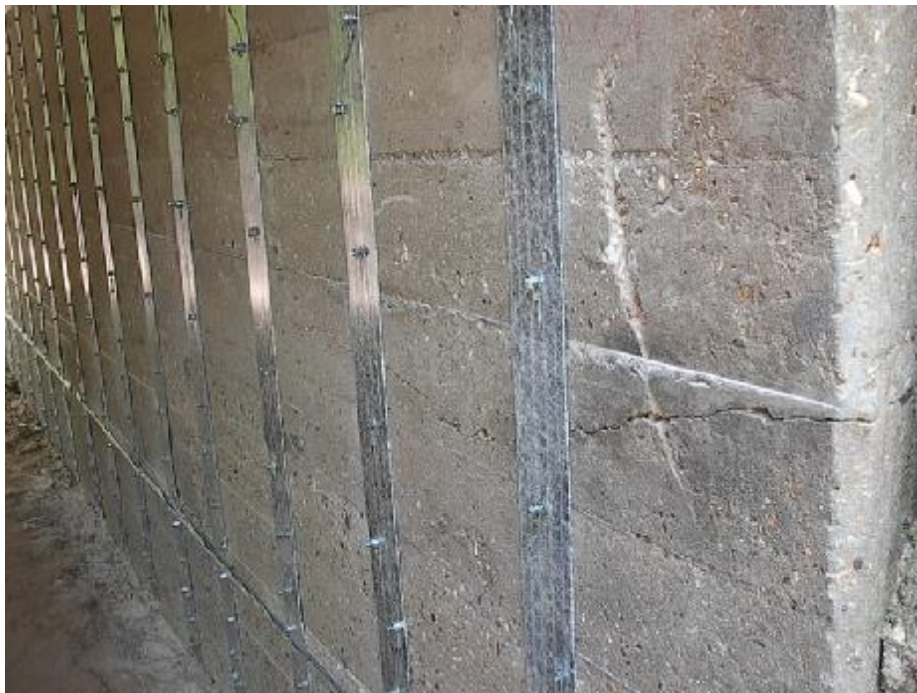
b) Bridging of the Crack Running Through the Abutment S4
