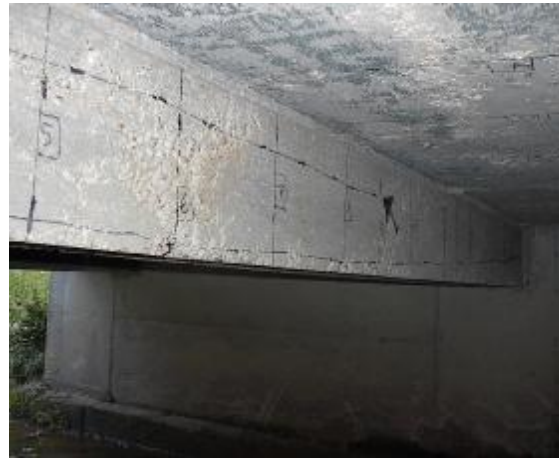
b) Central Girder
