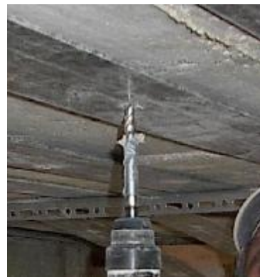
Figure C. 3. Drilling of the Holes in the Concrete
