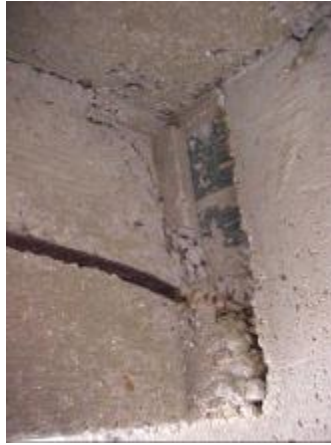
a) Exposed Bar in the Lateral Side
